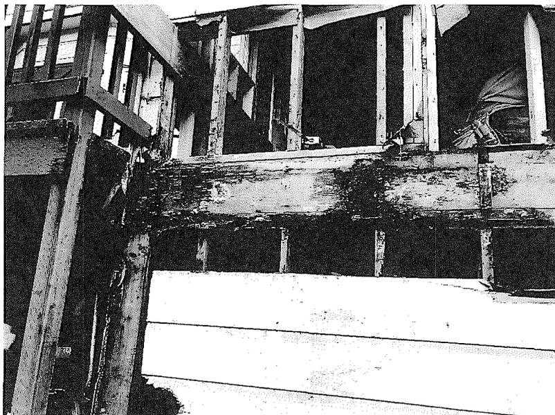
Detail photos of dry rot located at rear of building
