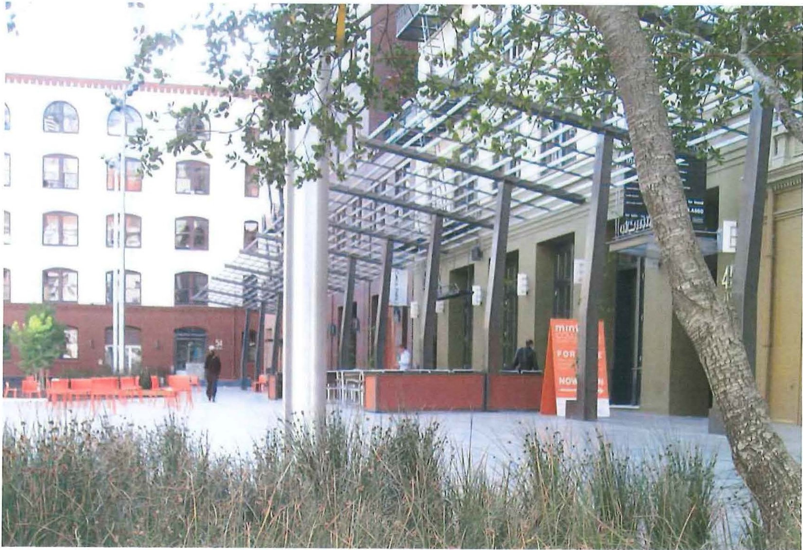
Mint Plaza, San Francisco, CA is an example of how LID can be integrated into an ultra-urban setting. The design includes rain gardens, permeable paving, and a subsurface infiltration gallery.
