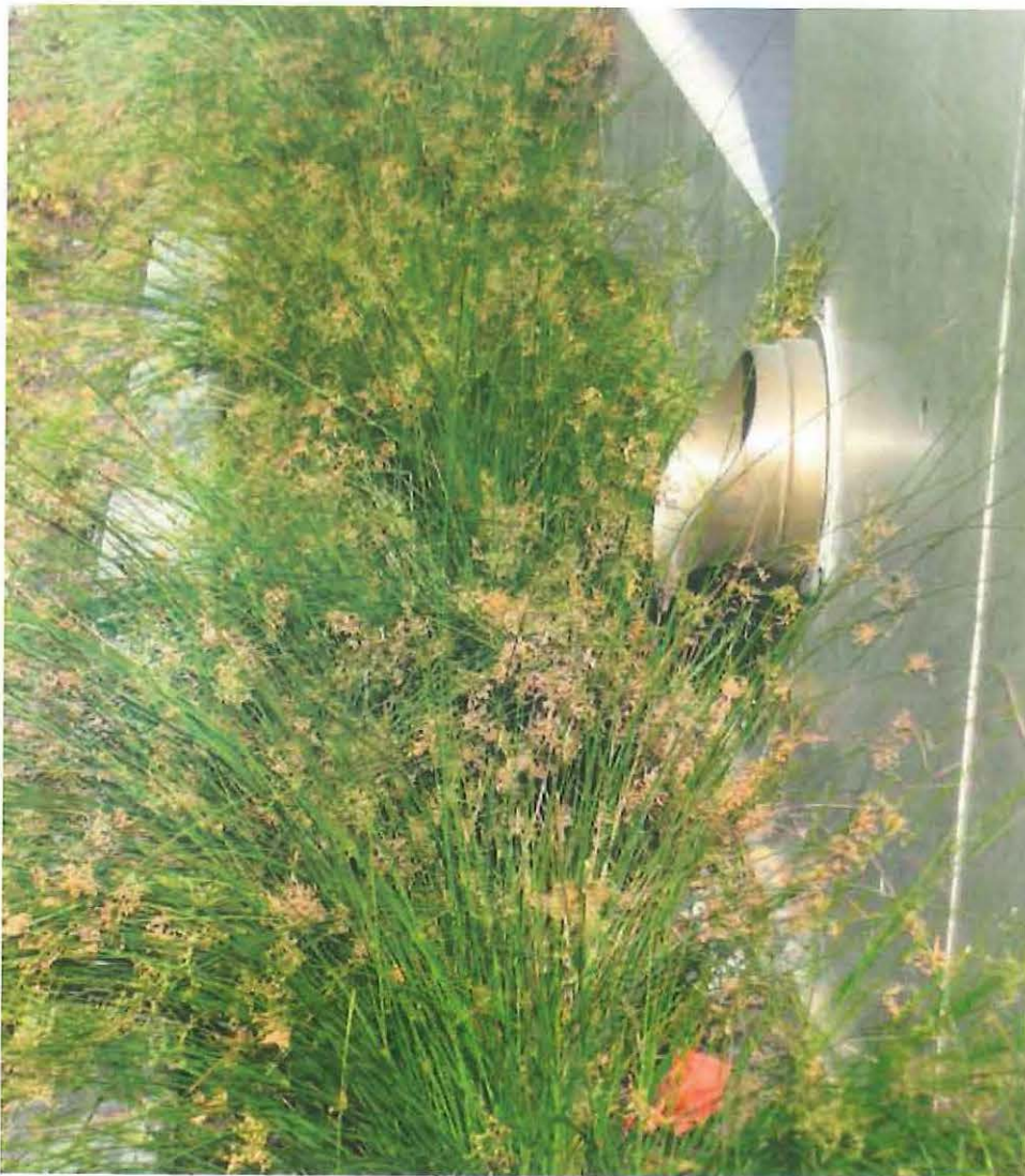
An interior roof drain discharges to a vegetated swale in Emeryville, CA. This properly designed and permitted stormwater facility is an example of an “approved alternate location” for stormwater discharge.
