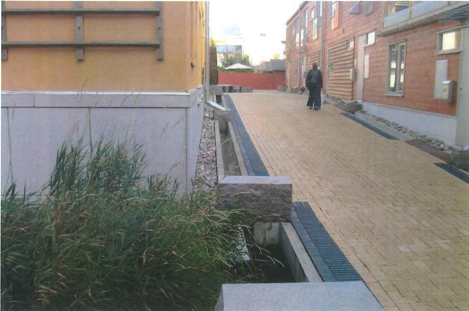
The Western Harbor, located in Malmö, Sweden, conveys and treats stormwater by implementing both parcel and block-scale surface systems that direct runoff to vegetation and ponds, which double as amenities throughout the neighborhood. Habitat value is enhanced through the use of various vegetation types. Photo: Andres Power
