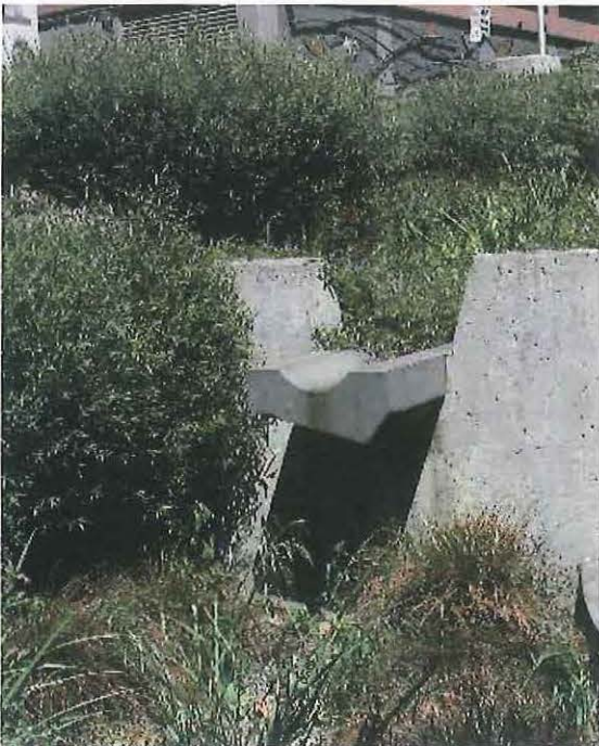
Weirs (top) and cascades (bottom) make street-side bioretention possible on steep slopes in Seattle, WA.
