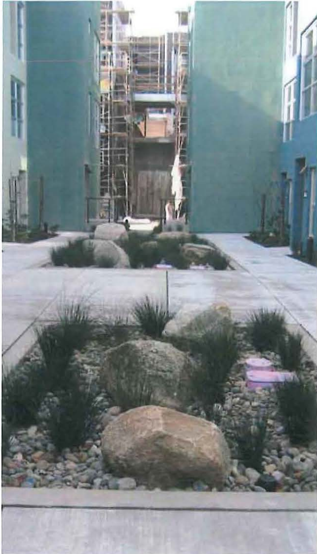
Linked bioretention cells are a central part of the design for the Glashauss development in Emeryville, CA.
