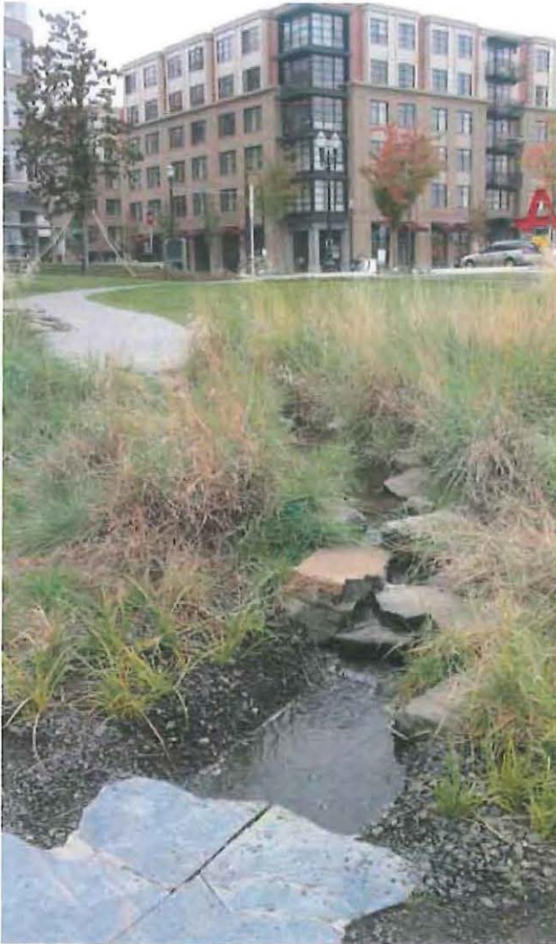
LID measures like the stormwater wetland in Portland's Tanner Springs Park treat polluted street runoff, thereby minimizing negative impacts to water quality.
