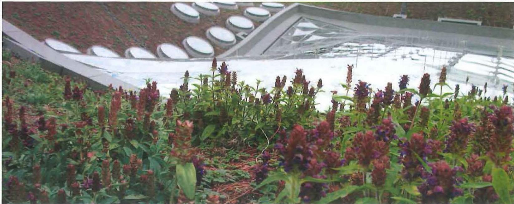
The Academy of Sciences in Golden Gate Park is targeting LEED Platinum certification and includes a 2.5 acre vegetated roof. Photo: Rana Creek - Living Architecture
