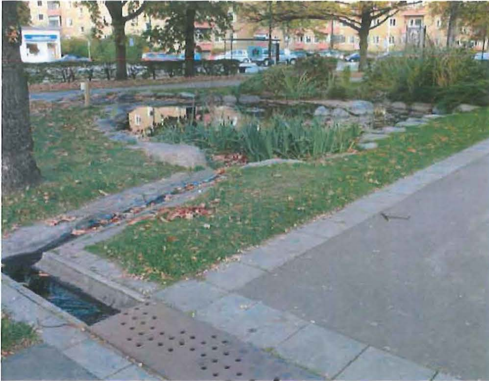
The Ekostaden residential development in Malmö, Sweden, channels all stormwater runoff through BMP treatment features such as bioswales, ponds, and wetlands as shown here. Photo: Brooke Ray Smith
