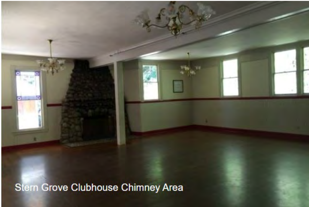
Trocadero Clubhouse, Social Hall/Meeting Room with fieldstone fireplace, view northwest, c. 2020. Source: San Francisco Recreation and Park Department website, accessed via https://sfrecpark.org/664/Stern-Grove-Clubhouse .
