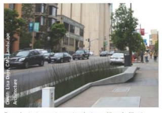
Example steetscape stormwater planters, with and without integrating seating elements.
