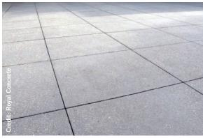
Enhanced cast-in-place concrete with saw-cut joints.
