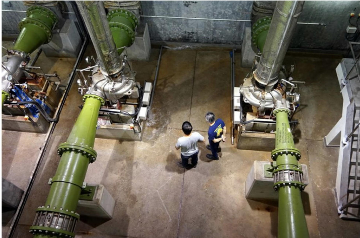
Figure 2-9: Pumps at Wan Chai Seawater Treatment Facility Supply Toilet Flushing Water
