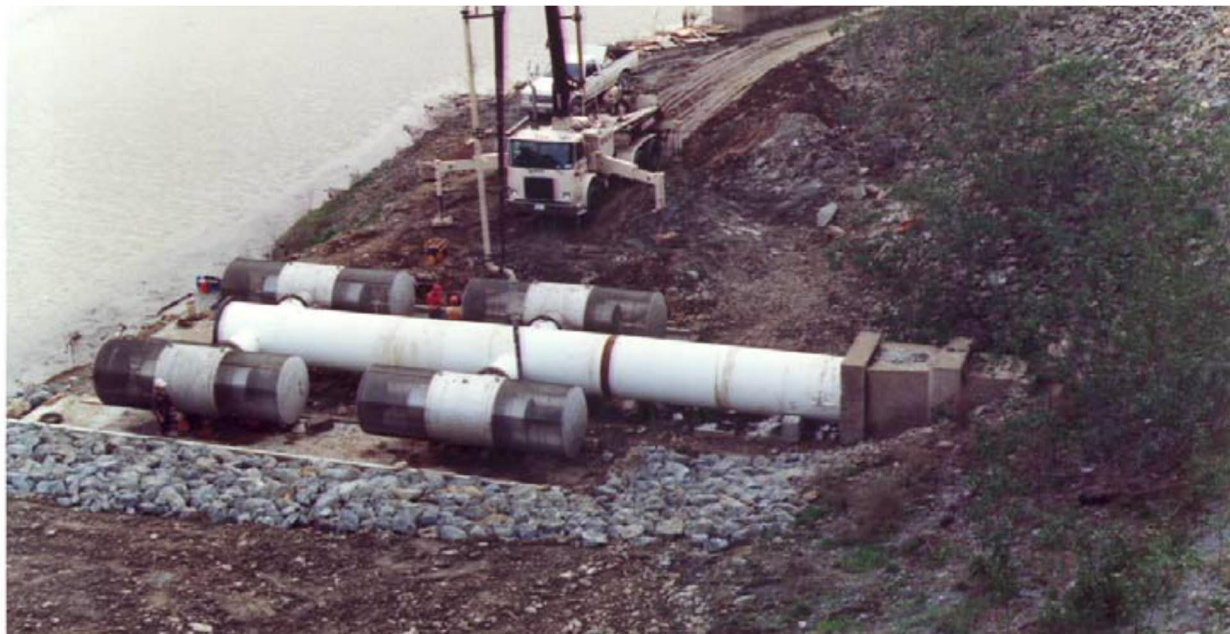
Figure 7-2: Completed Intake Screens on Open-Water Intake Tunnel
