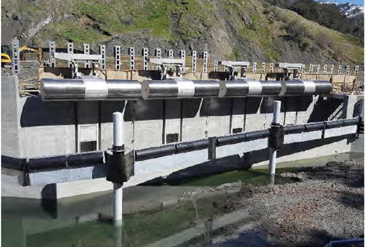
Figure 7-3: Intake Screens at Alameda Creek Diversion Dam
