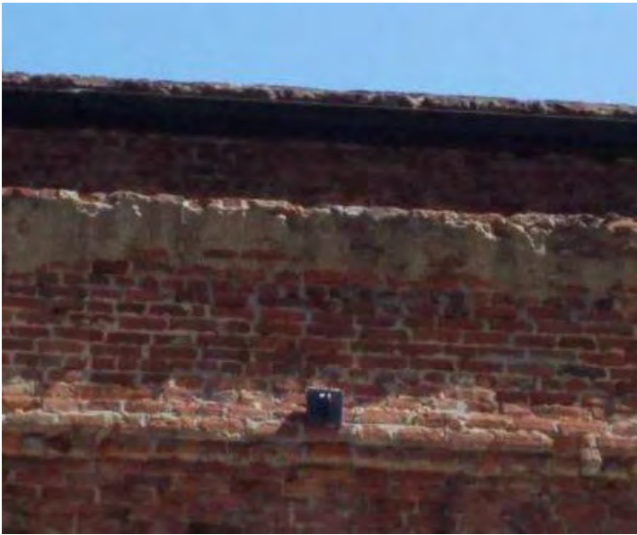
Close up of patched bricks at cornice, 2017. Source: Page & Turnbull, Inc. (2017) report
