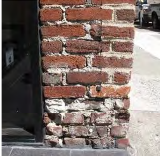
Figure 11. 447 Battery Street primary façade, close-up of street level brick variation and patching.
