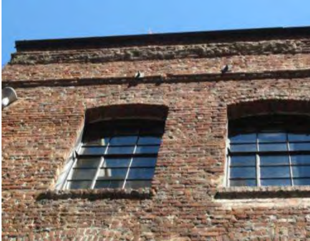
Figure 15. 447 Battery Street, close-up of brick belt line and steel-sash windows.
