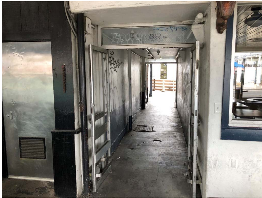
Figure 26 Double doors missing glass
