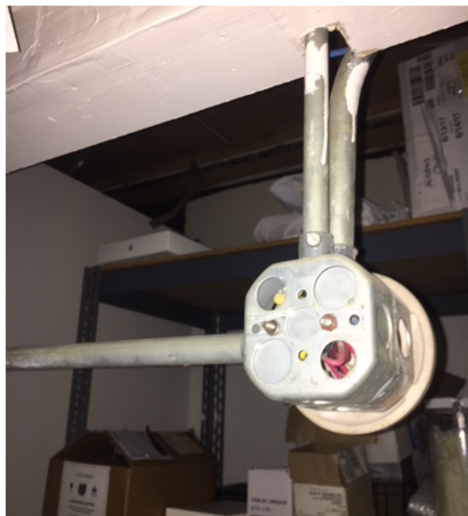
Figure 19 Missing knock outs
