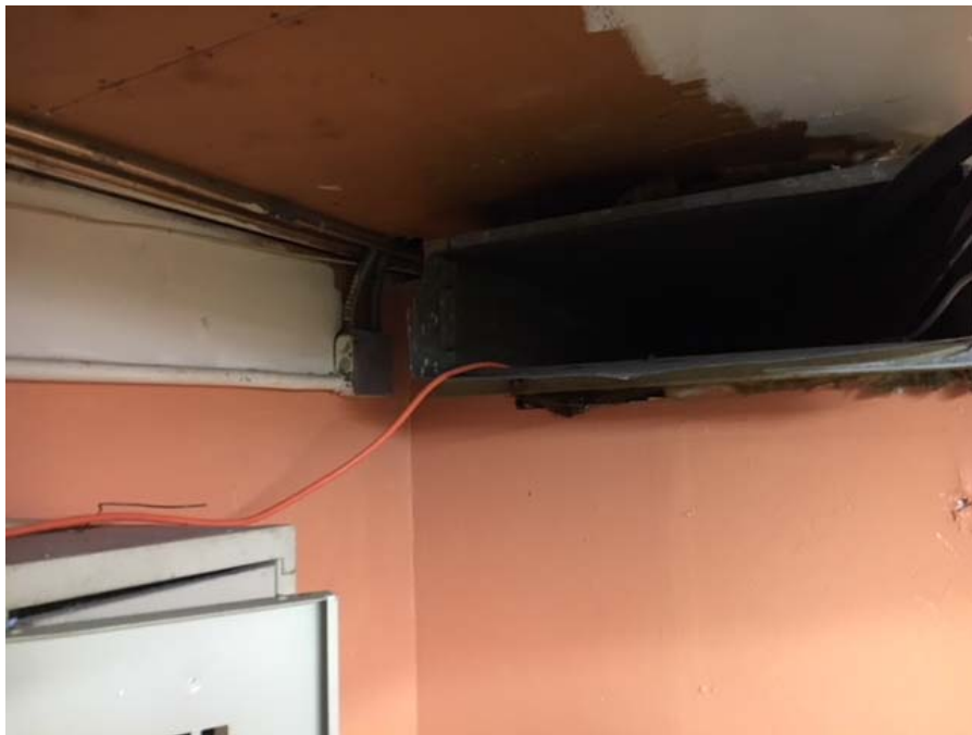
Figure 15 Extension cord inside HVAC duct
