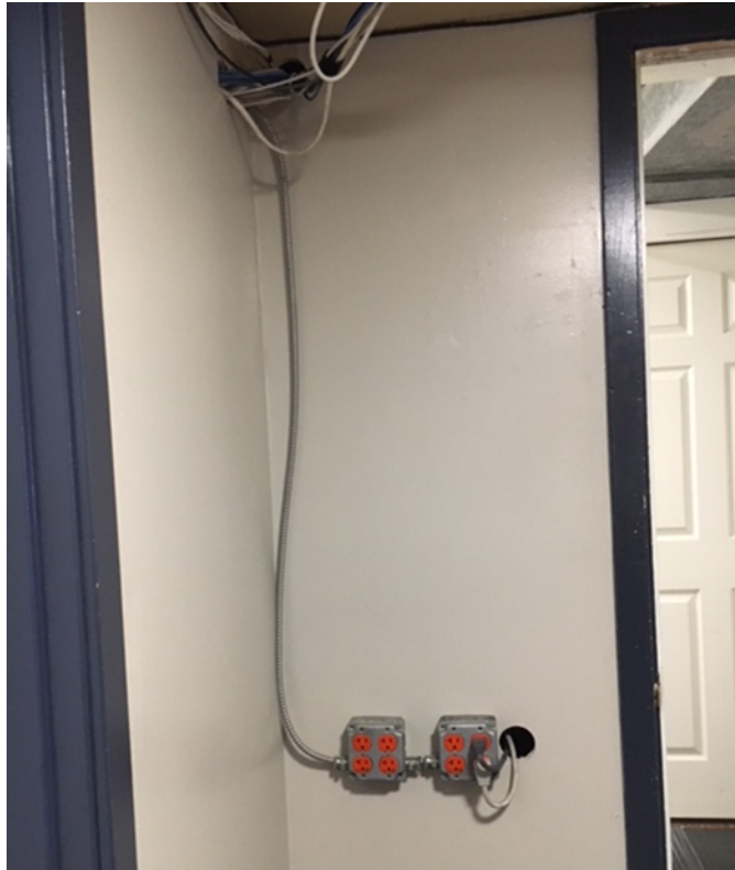
Figure 21 Open wiring, not secured
