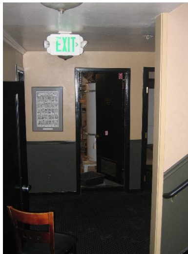
Figure 53: 2 nd Flr. Landing, missing handrail Extensions
