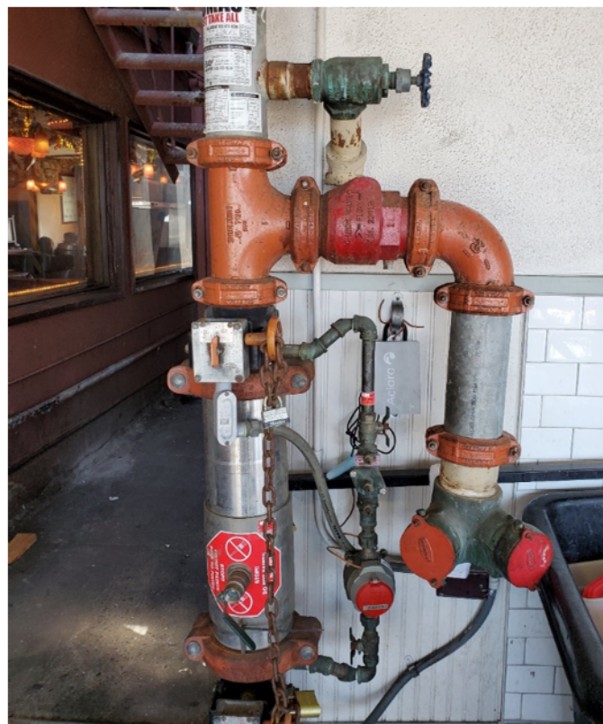
Figure 4 Fire sprinkler riser
