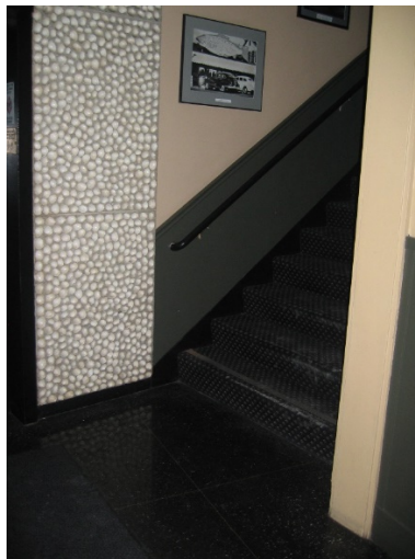
Figure 19: Staircase #1, missing Handrail Extensions
