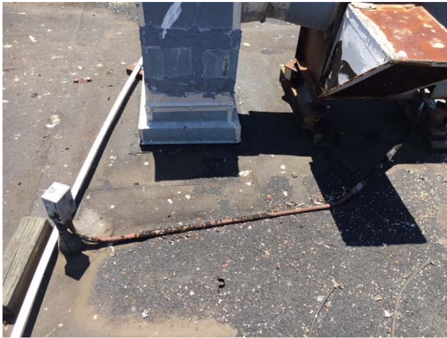
Figure 14 Unsupported conduit
