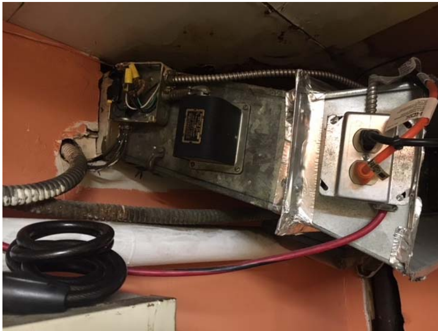
Figure 16 Missing cover, extension cord being used as permanent wiring
