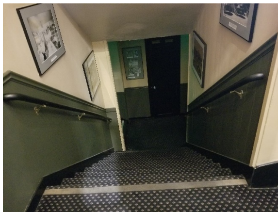
Figure 21: Staircase #1, missing Handrail Extensions
