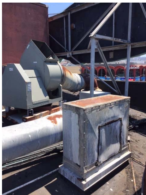
Figure 12 Roof Duct surface rust
