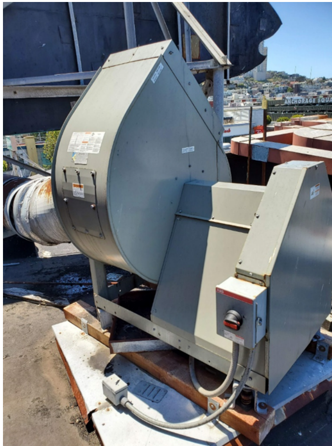
Figure 5 Newer kitchen exhaust fan
