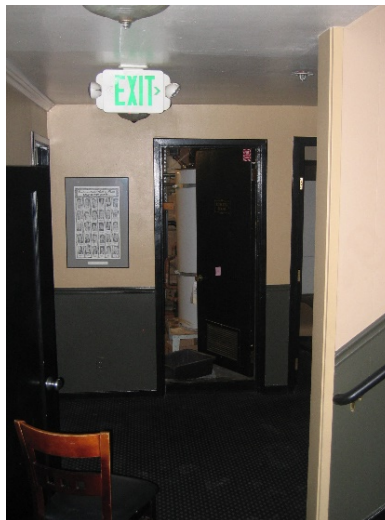
Figure 53: 2 nd Flr. Landing, missing handrail Extensions
