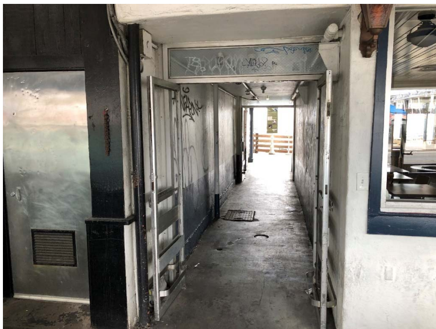
Figure 26 Double doors missing glass
