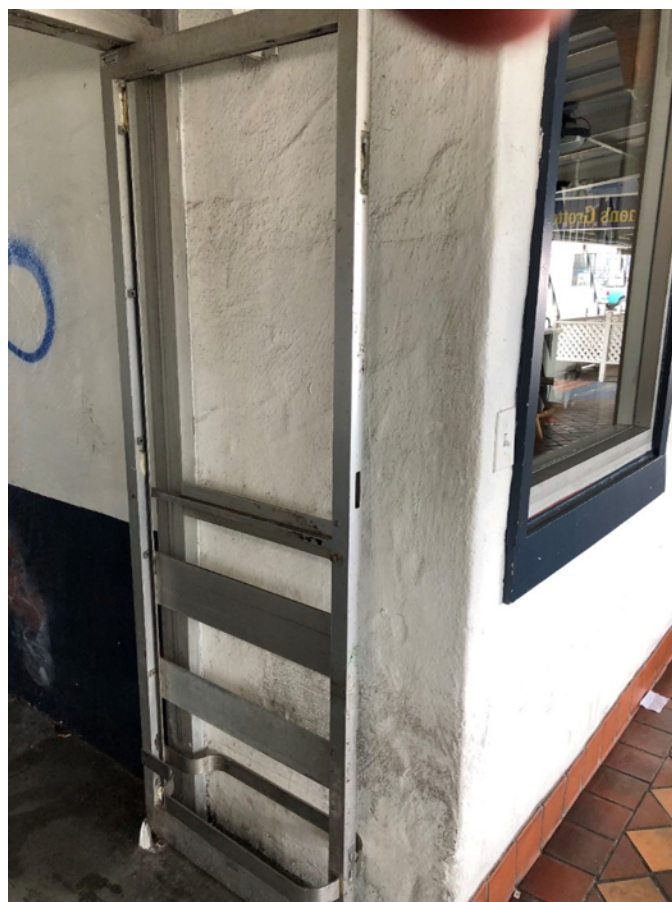
Figure 27 Double doors missing glass (Right)
