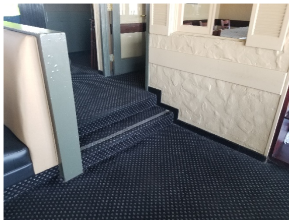
Figure 75: 3 rd Floor Steps to Mid Dining, missing Handrail.
