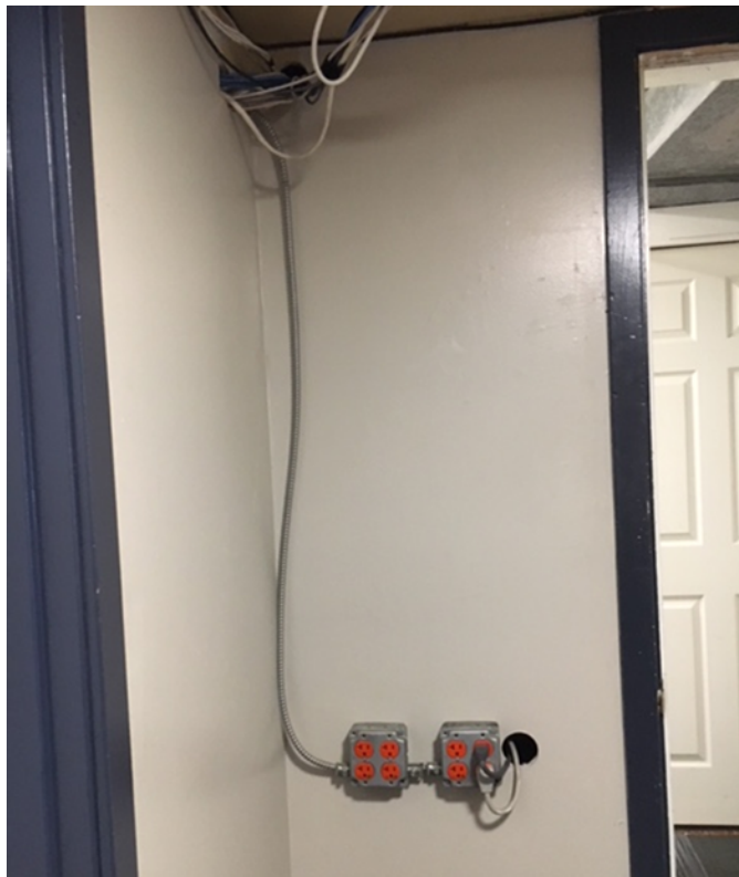
Figure 21 Open wiring, not secured
