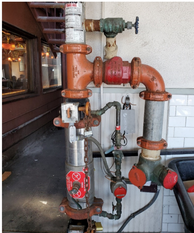
Figure 4 Fire sprinkler riser
