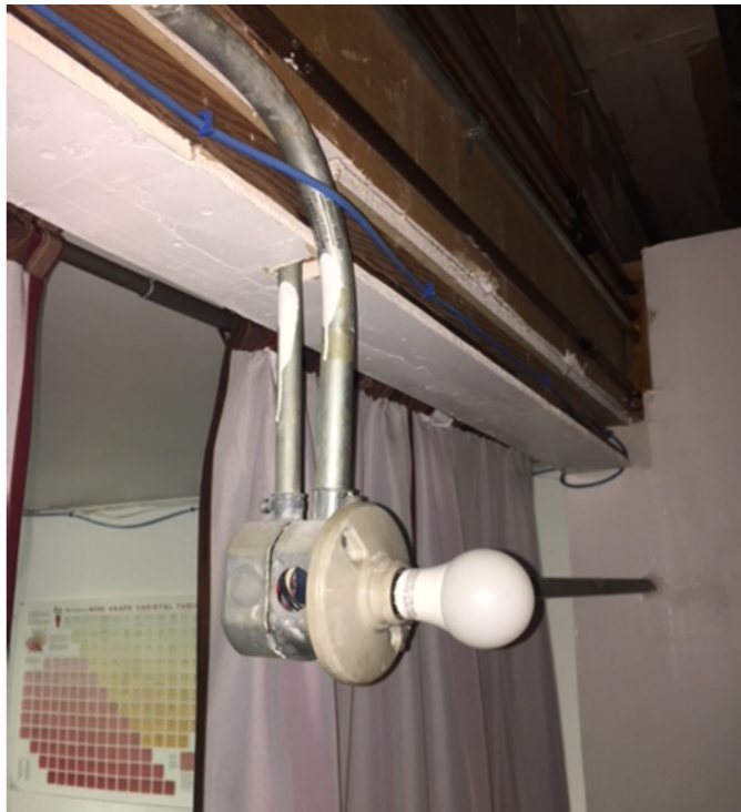
Figure 20 Missing knock outs
