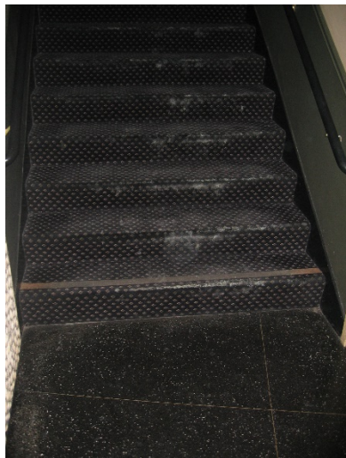
Figure 18: Staircase #1, missing Handrail Extensions
