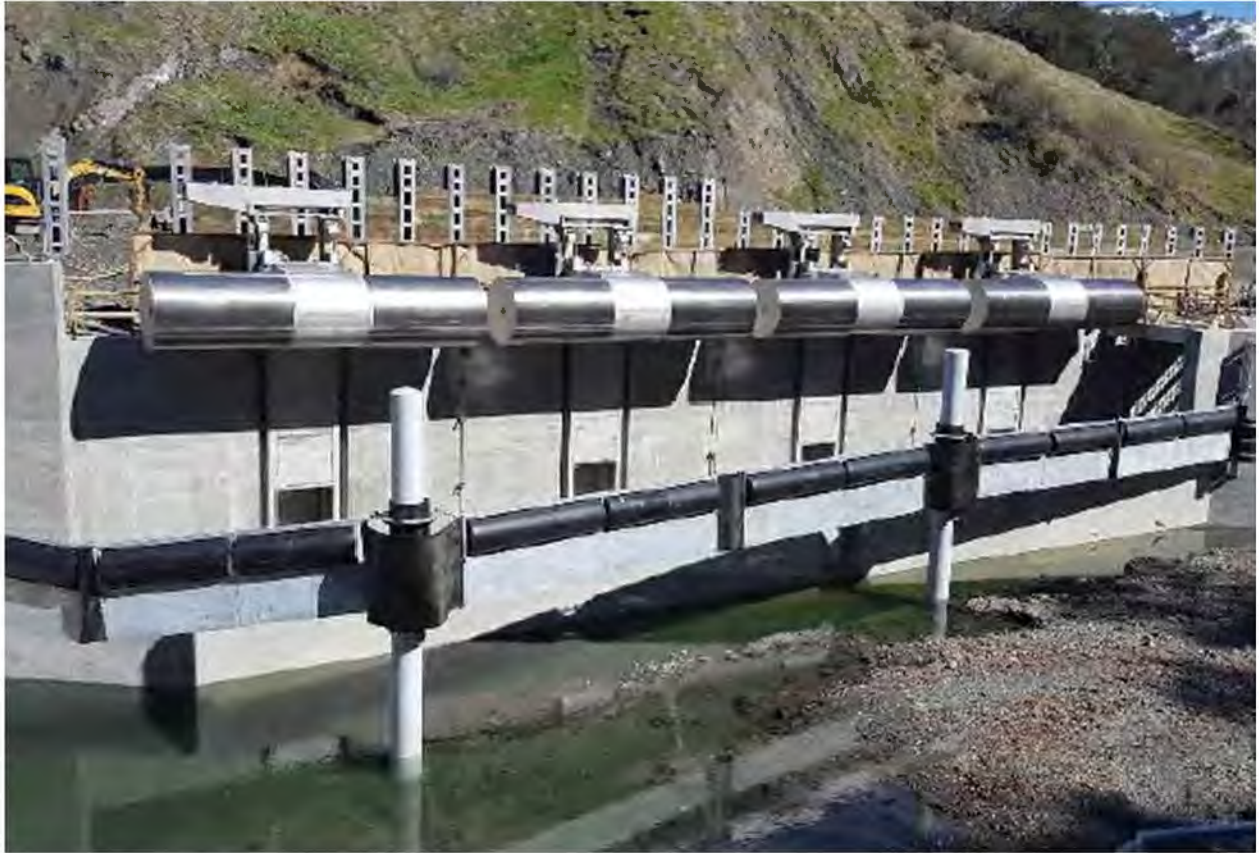
Figure 7-3: Intake Screens at Alameda Creek Diversion Dam
