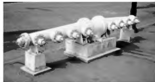
Figure 2-5: Typical Fireboat Manifold Inlet
