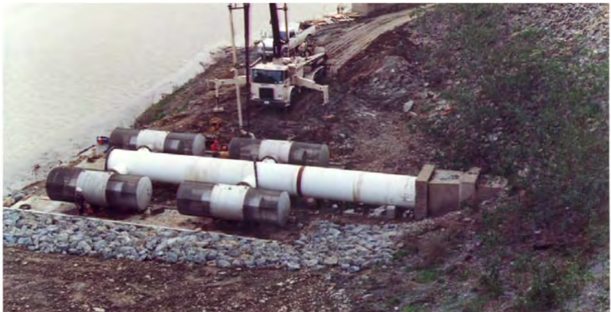
Figure 7-2: Completed Intake Screens on Open-Water Intake Tunnel
