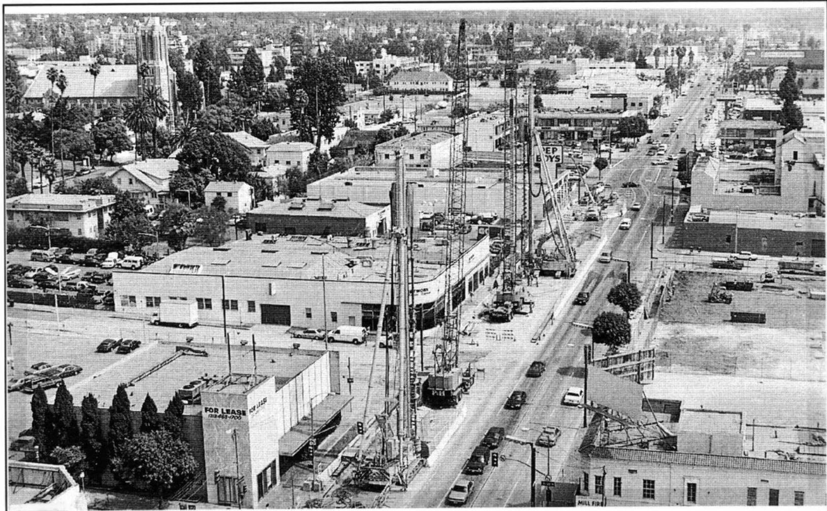
Figure 5.20-1: Soil Cement Wall Augers In Use
