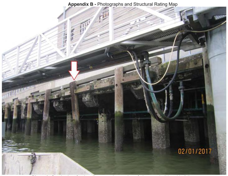
Photo 9. One broken fender pile on northern edge of pier near bulkhead building.
