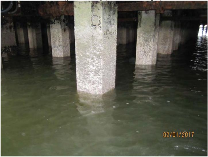
Photo 7. Minimal section loss at the concrete pile jackets near the waterline
