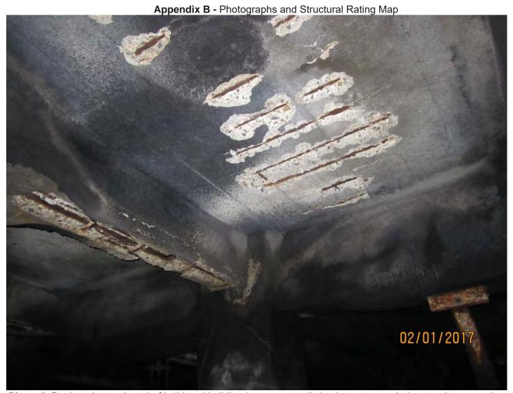
Photo 5. Deck under north end of bulkhead building has more spalls in shotcrete repair due to rebar corrosion
