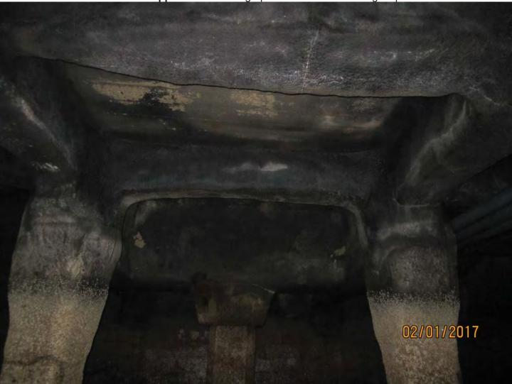
**Photo** 3. Typical conditions of marginal wharf under bulkhead building. Previous shotcrete repair in serviceable condition, some hairline cracks and scour.
