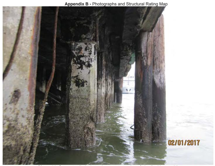
Photo 11. Concrete pile jackets along eastern edge of pier (looking north)
