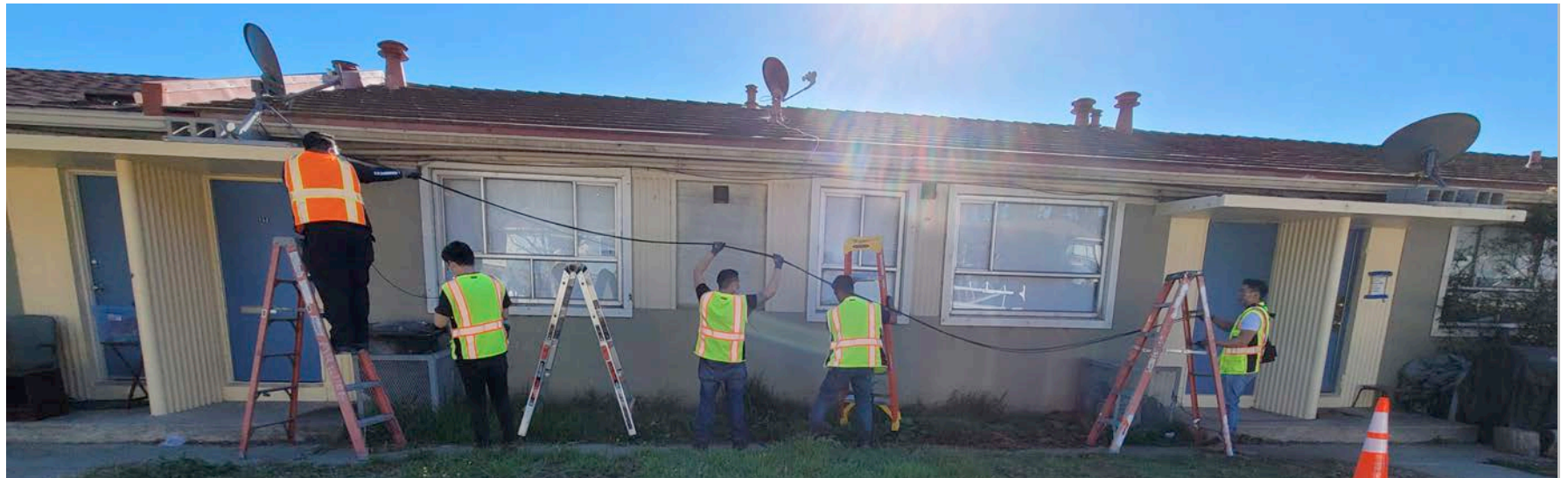
Fiber Broadband Installation
