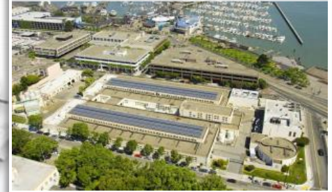
North Point Wet Weather Facility
