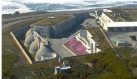
Oceanside Treatment Plant
