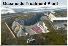
Avg. Dry Weather Flow: 12mgd Wet Weather Cap.: 175mgd
