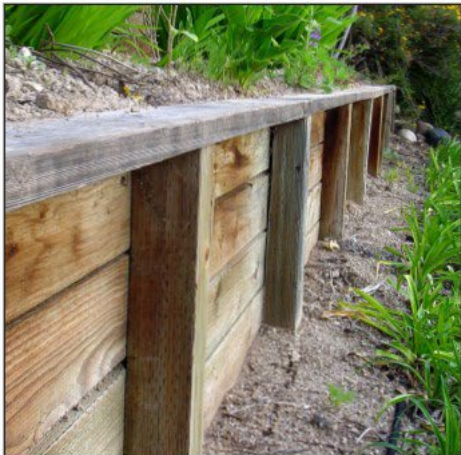
3 REDWOOD RETAINING WALLS
