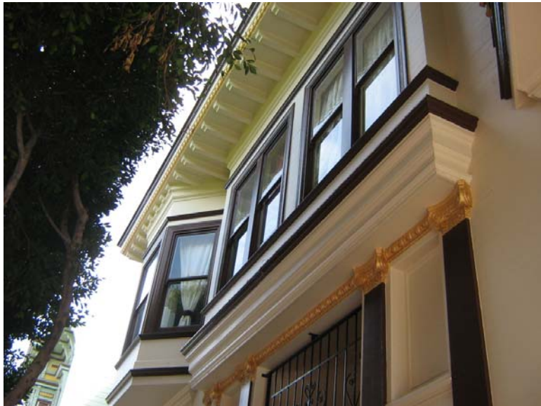
View looking southeast at upper level of primary façade. Source: Page and Turnbull
