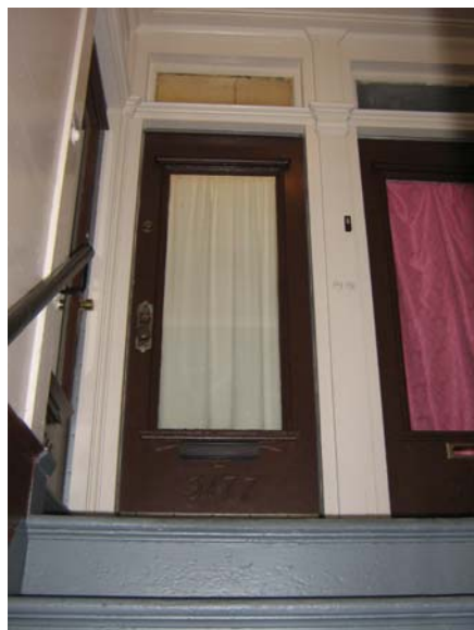
View looking south at primary entranceway. Source: Page and Turnbull
