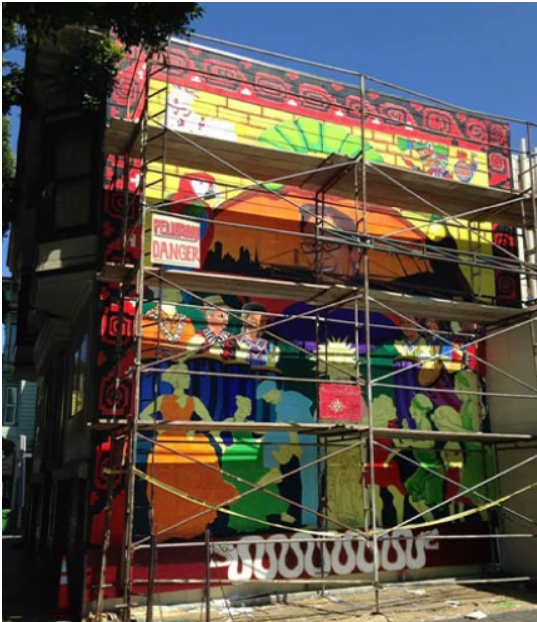
Chata Gutierrez mural under construction, 2015. Source: General 2 — Carlos Kookie Gonzalez (cgonzalezmurals.com)
