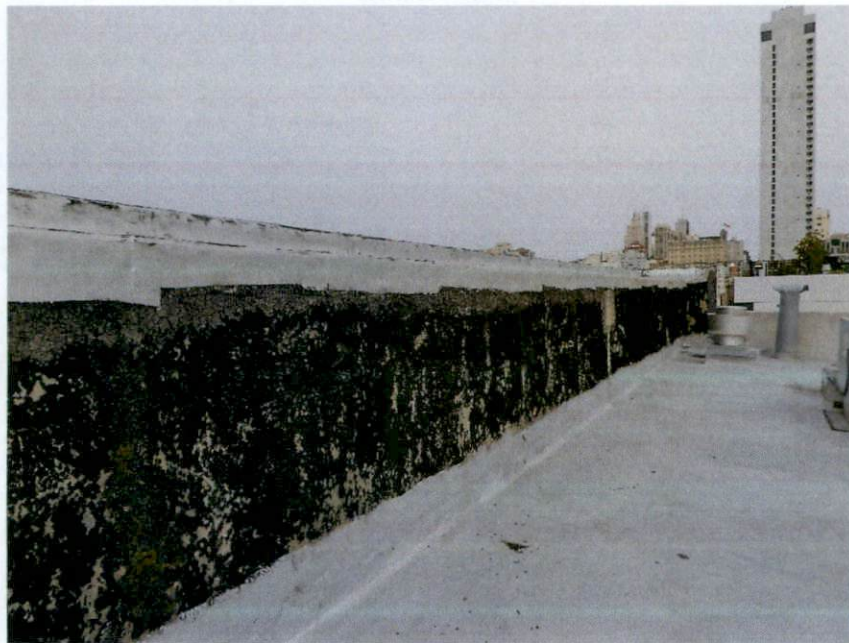
Photo O: View of parapet stem wall at roof level. Image shows damage to cement plaster and asphalt coating and biogrowth.
