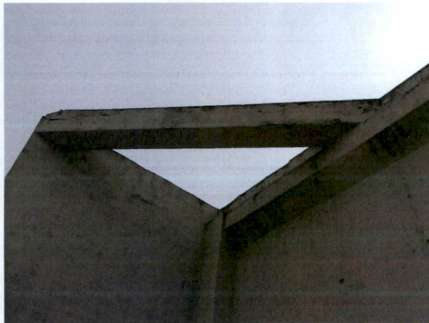
Photo R1: View of lateral bracing at upper parapet along Market Street façade. Looking south.
