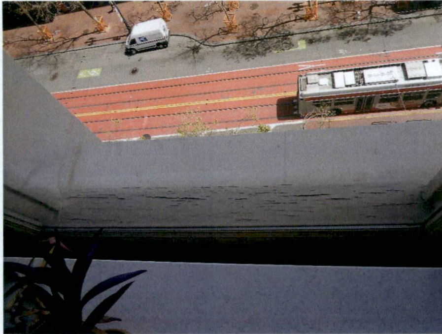
Photo 24: Example of delaminating paint at sixth level wood sill - Market Street.
