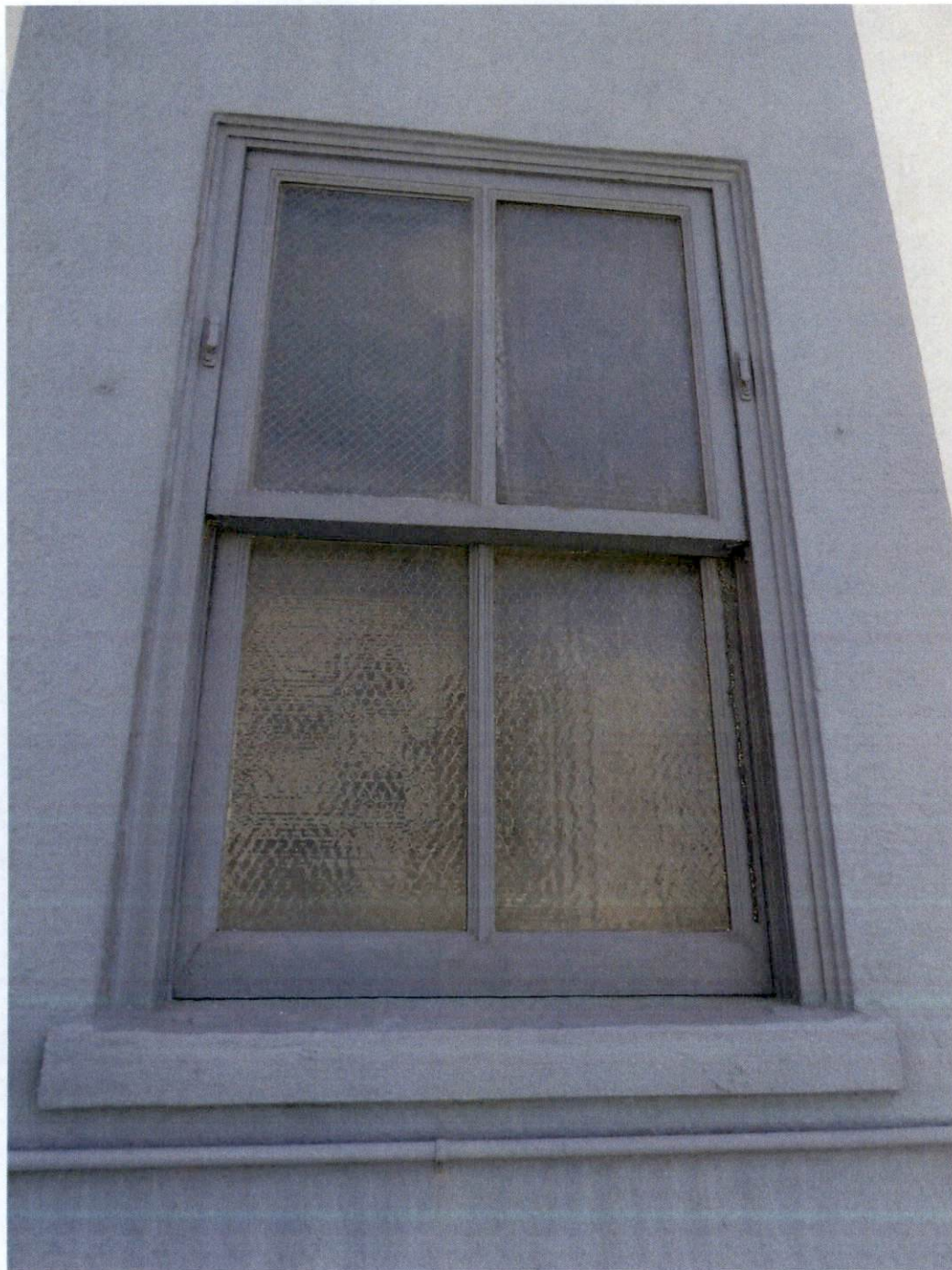
Photo J: View of sheet metal and wood window at north elevation looking south at 7 th level exterior.
