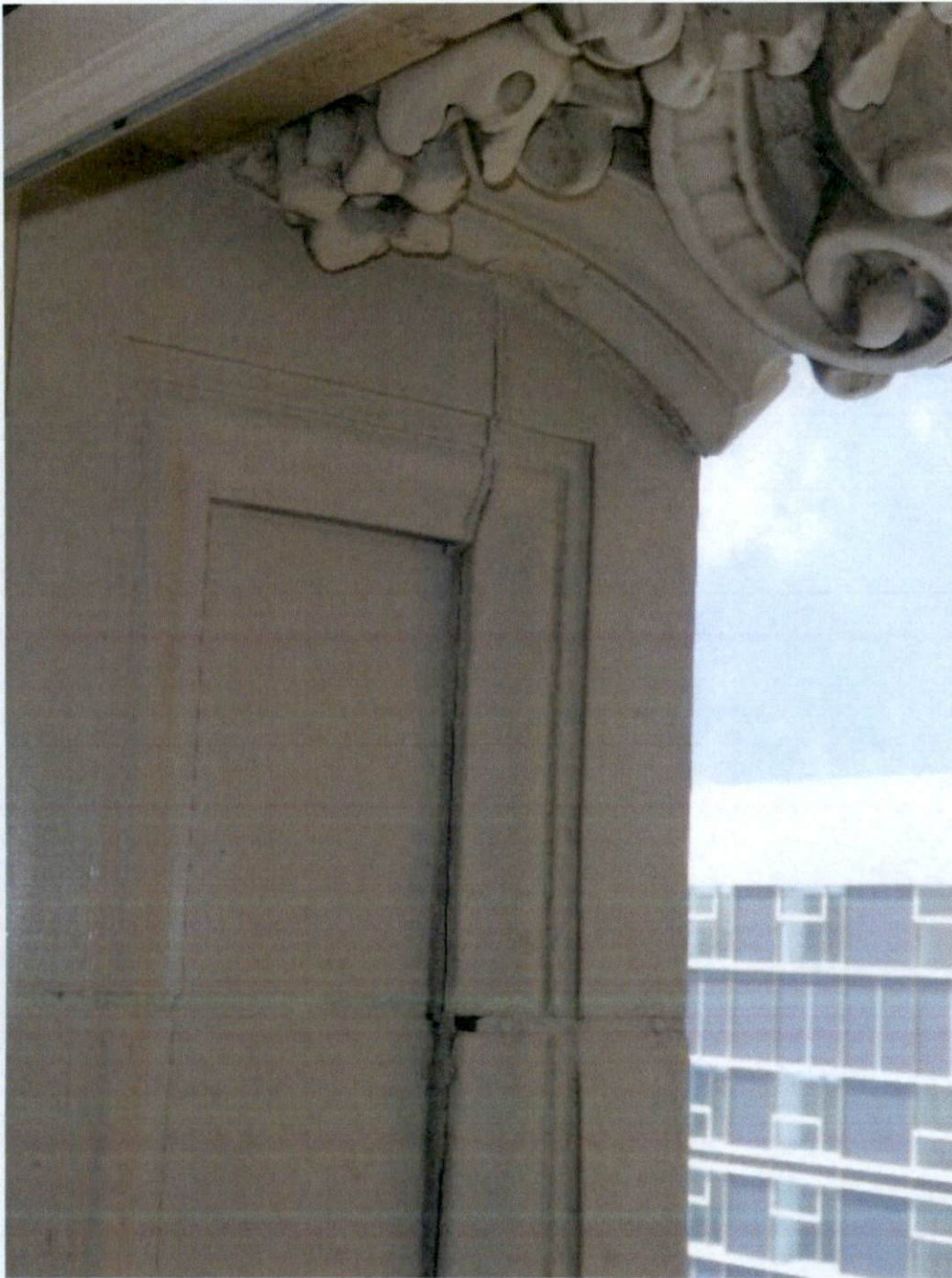
Photo 25: Example of missing mortar at fifth level window head – Market Street.
