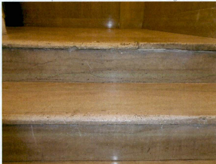
Photo 37: Example of marble spalling at stair nosing – First to Second Floor.
