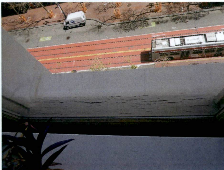
Photo 24: Example of delaminating paint at sixth level wood sill - Market Street.
