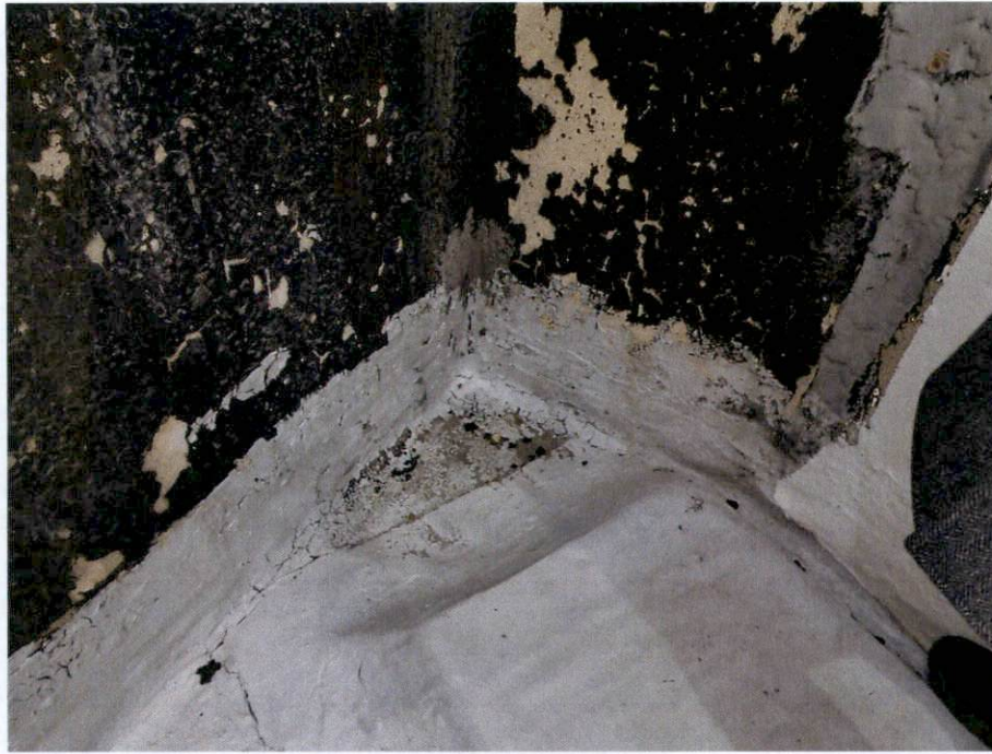
Photo 32: Failure at vertical parapet membrane – Roof.
