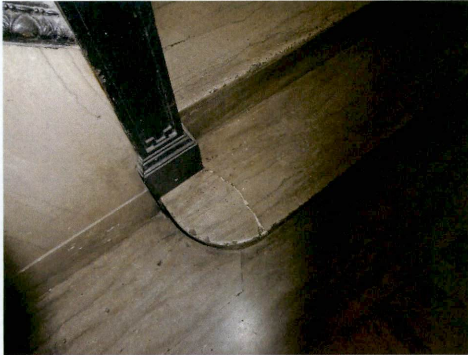
Photo 46: Cracked marble tread - Basement.
