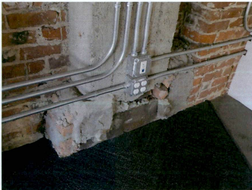
Photo Y: Detail of brick masonry at concrete walls at 3 rd level with exposed steel members and deteriorated mortar joints.
