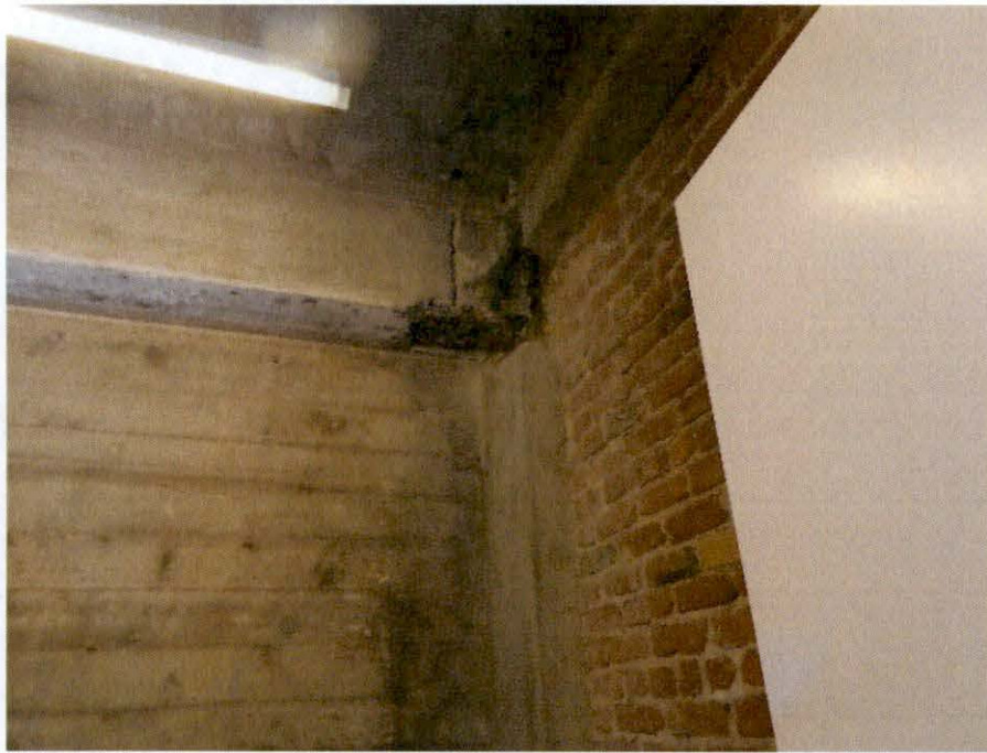
Photo 39: Example of exposed structural steel at steel beam and column connection - Fifth Floor.
