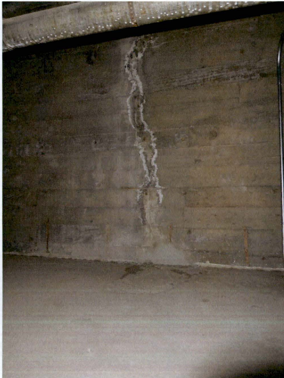
Photo 53: Vertical crack at concrete wall – Tenth Floor.
