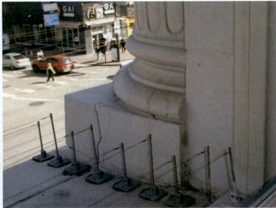
Photo 22: Example of cracks, incipient spalling at third level engaged pilaster base - Market Street.
