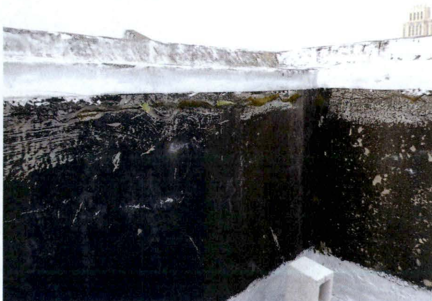
Photo 31: Parapet wall biological growth and cracking - Roof.
