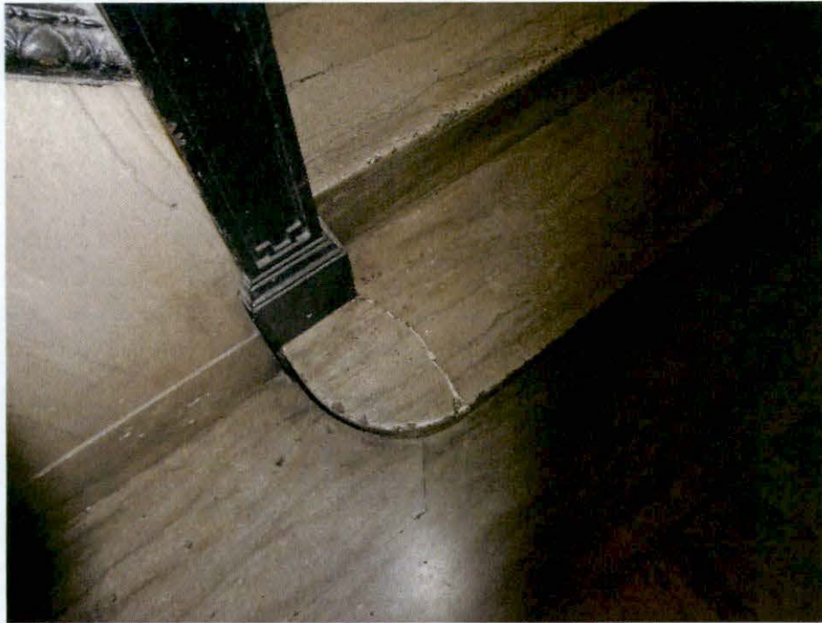
Photo 46: Cracked marble tread - Basement.
