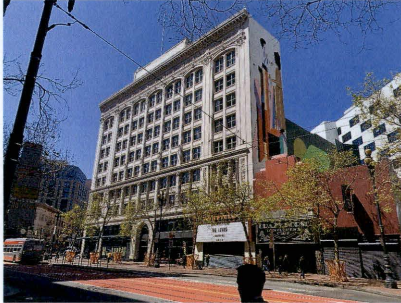
Photo A: Overall view of 988 Market Street façade. Mural along east façade visible at right side of image. Glass storefront visible at ground and second levels with terra cotta elements at the third through tenth levels. (All photos taken by P&T 04/17/2023, unless otherwise noted)
