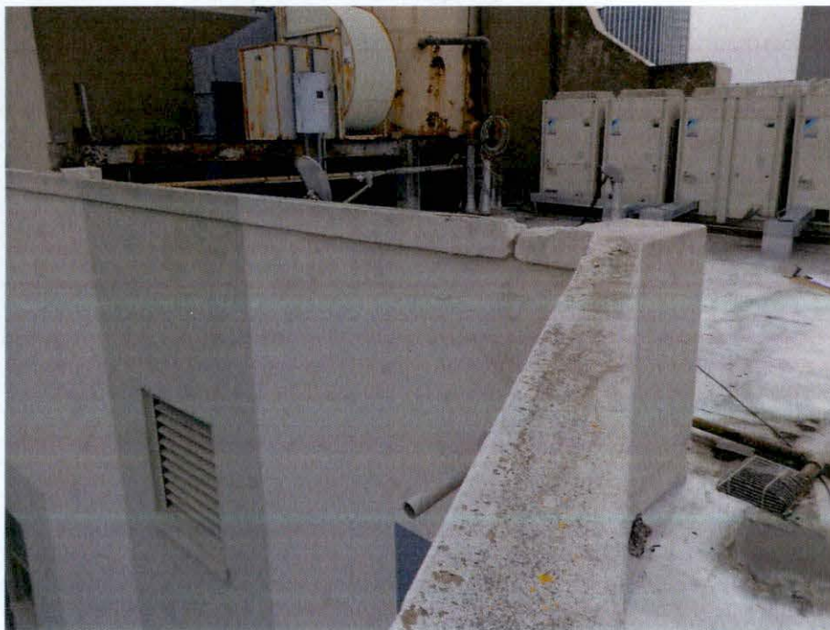
Photo 33: Cracking in cement plaster - Roof.
