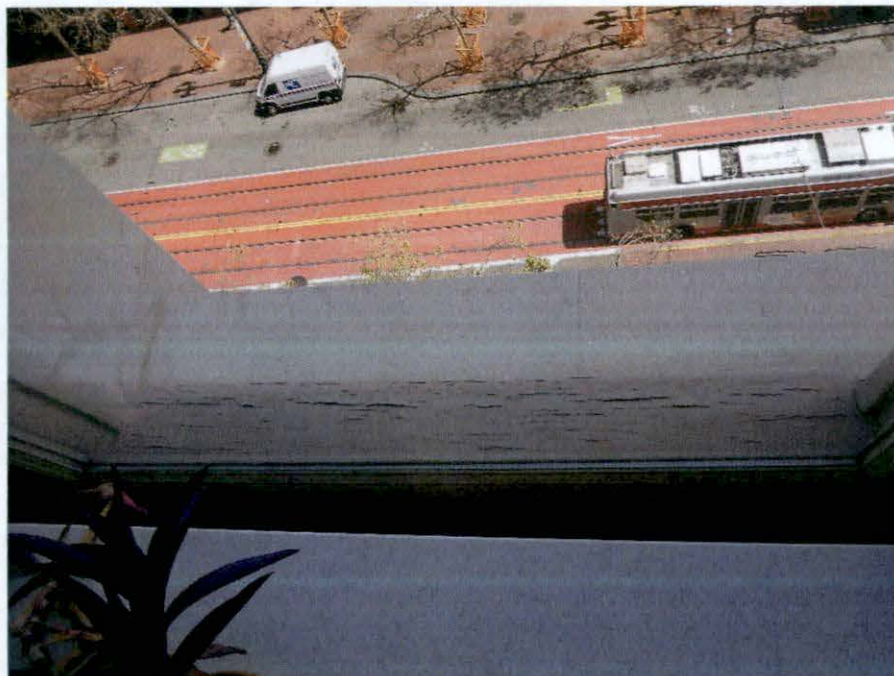
Photo AA: Detail view of deteriorating wood windowsill on sixth level along Market Street elevation, looking south.
