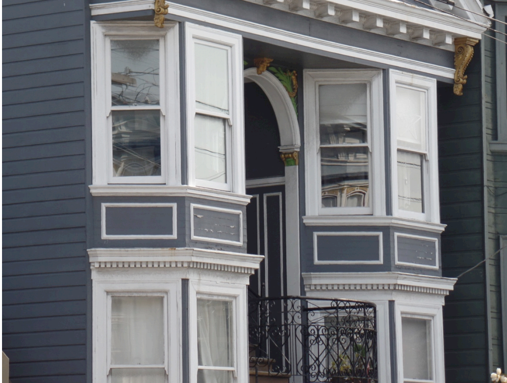
Figure 11: Front elevation view of peeling paint, worn wood elements at bay windows on third level (Garavaglia Architecture, 2023).
