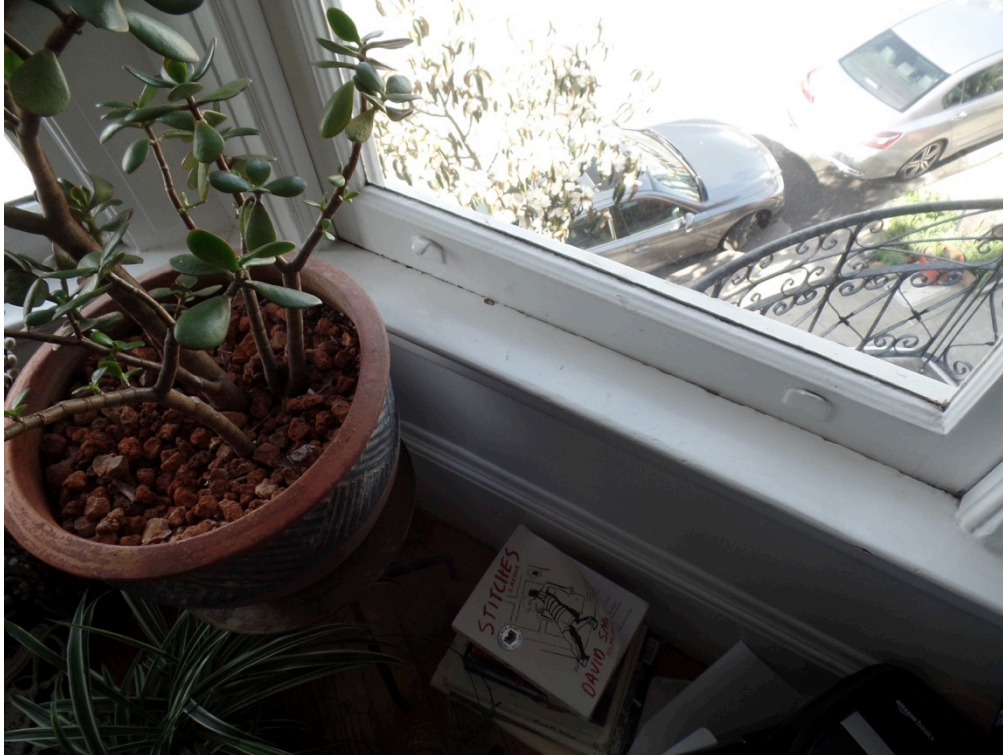
Figure 17: Interior view of front bay window in Unit 152A. Note deterioration at interior sill (Garavaglia Architecture, 2023).
