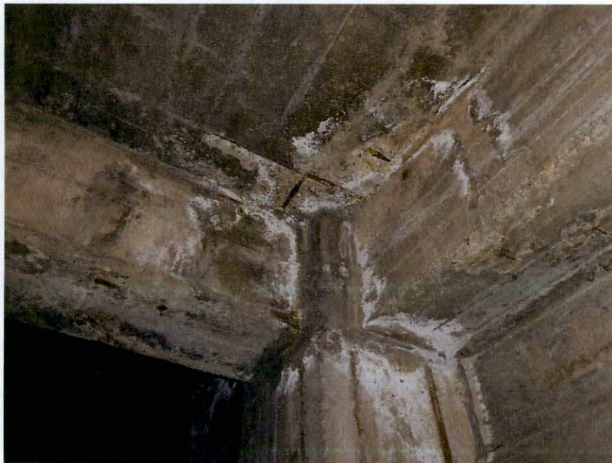
Photo 48: Exposed rebar and efflorescence at corner of concrete encased steel column and beams – Tenth Floor.
