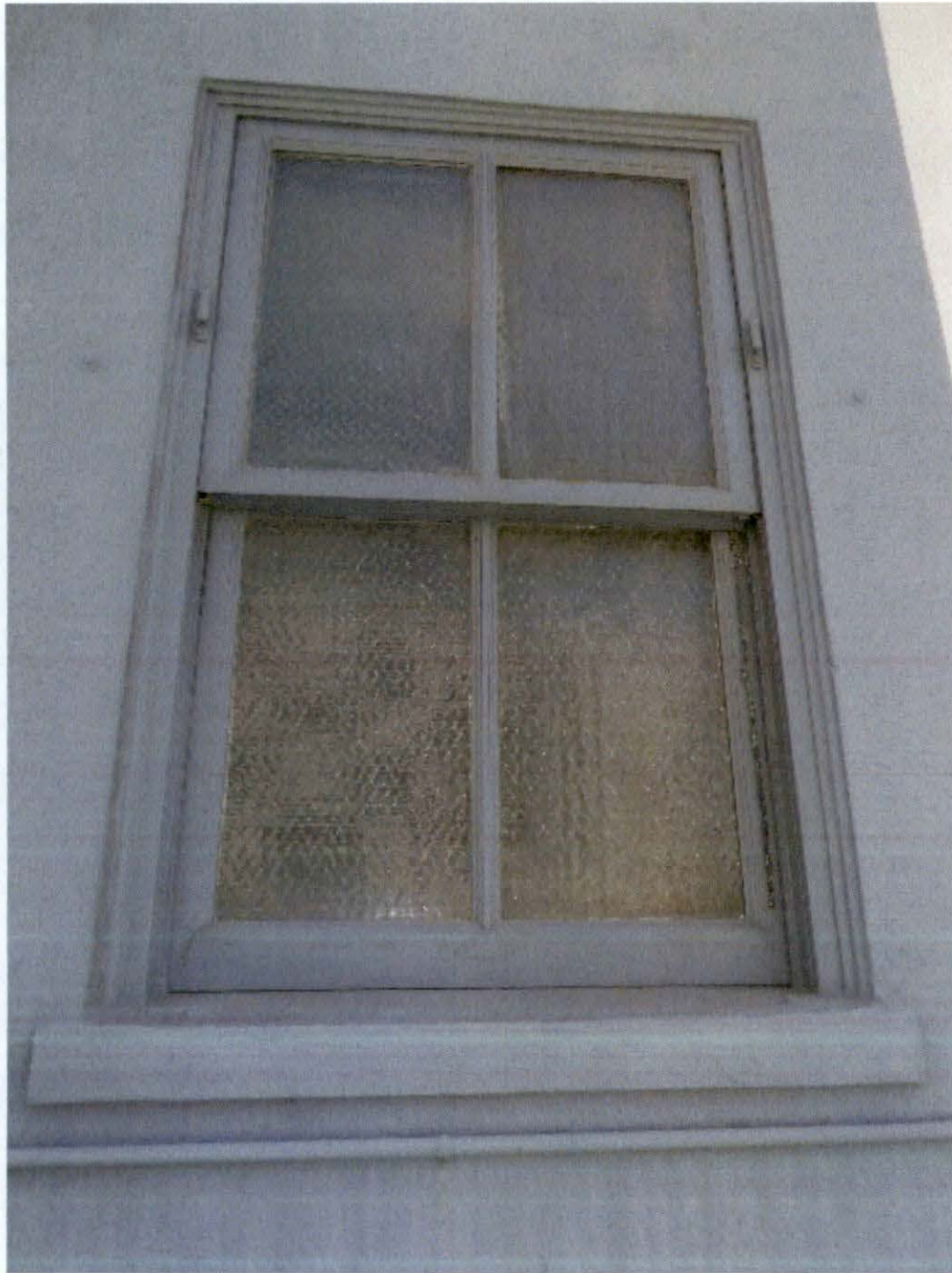
Photo 28: Example of original double hung sheet metal window (2 over 2 lites) with textured wire glass that is in good condition – North Façade.
