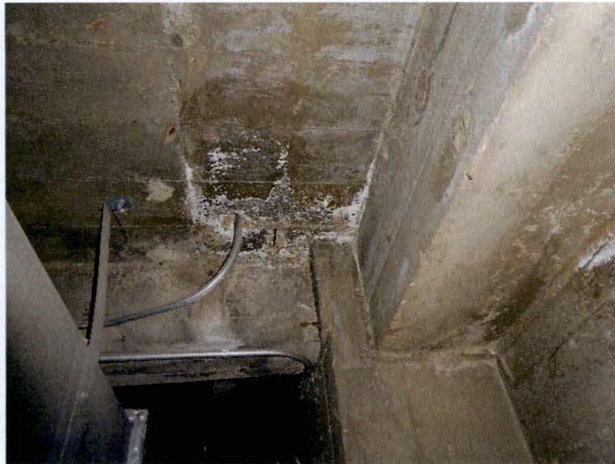
Photo 51: Efflorescence at hole in concrete for conduit – Tenth Floor.
