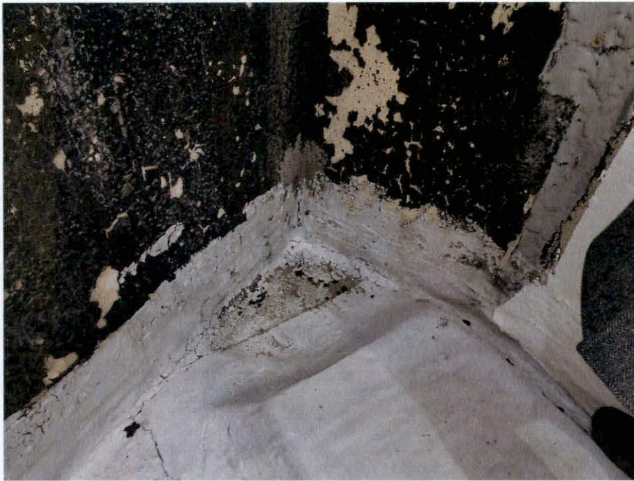
Photo 32: Failure at vertical parapet membrane – Roof.
