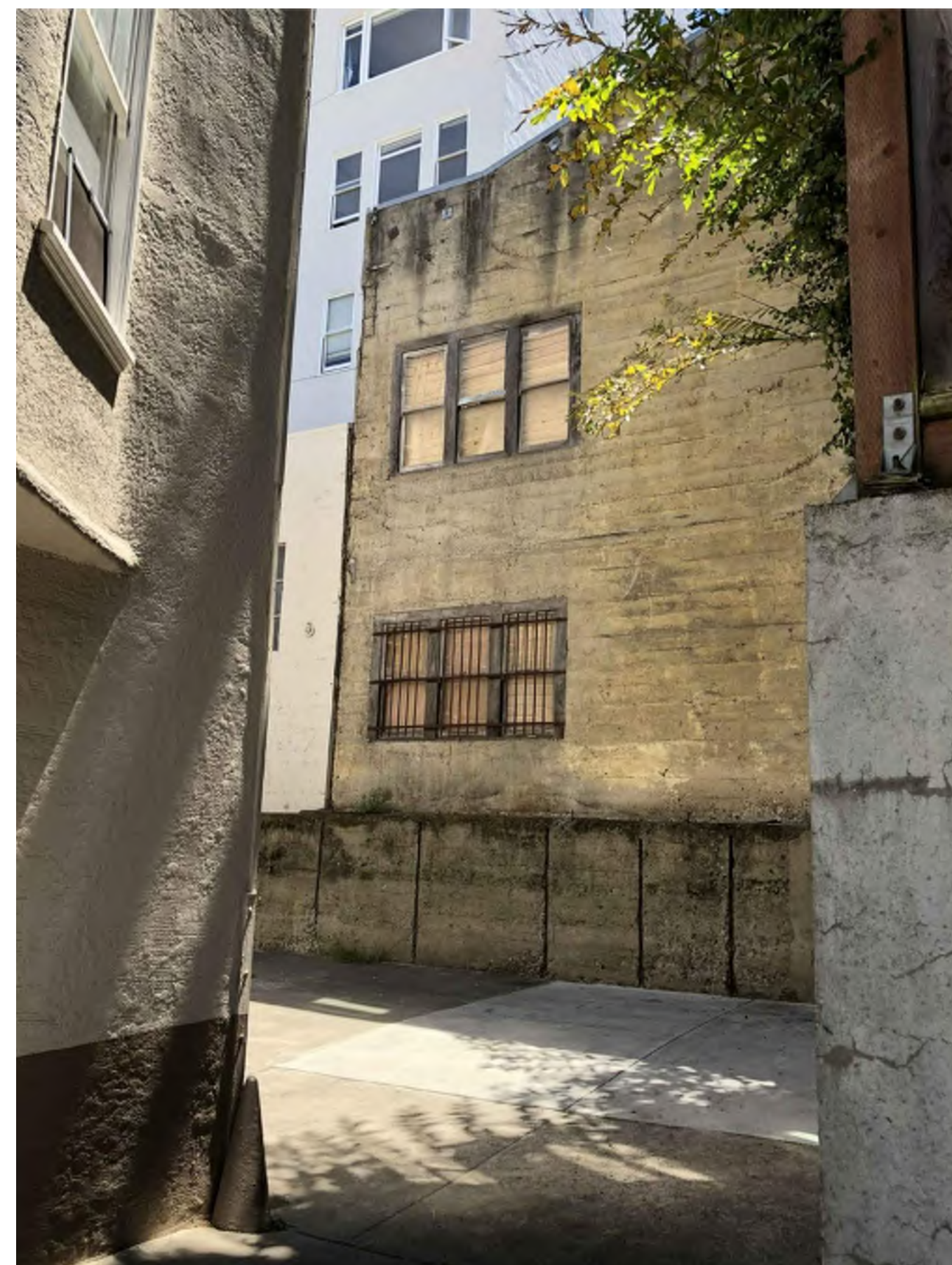
4 REAR BUILDING FACADE
