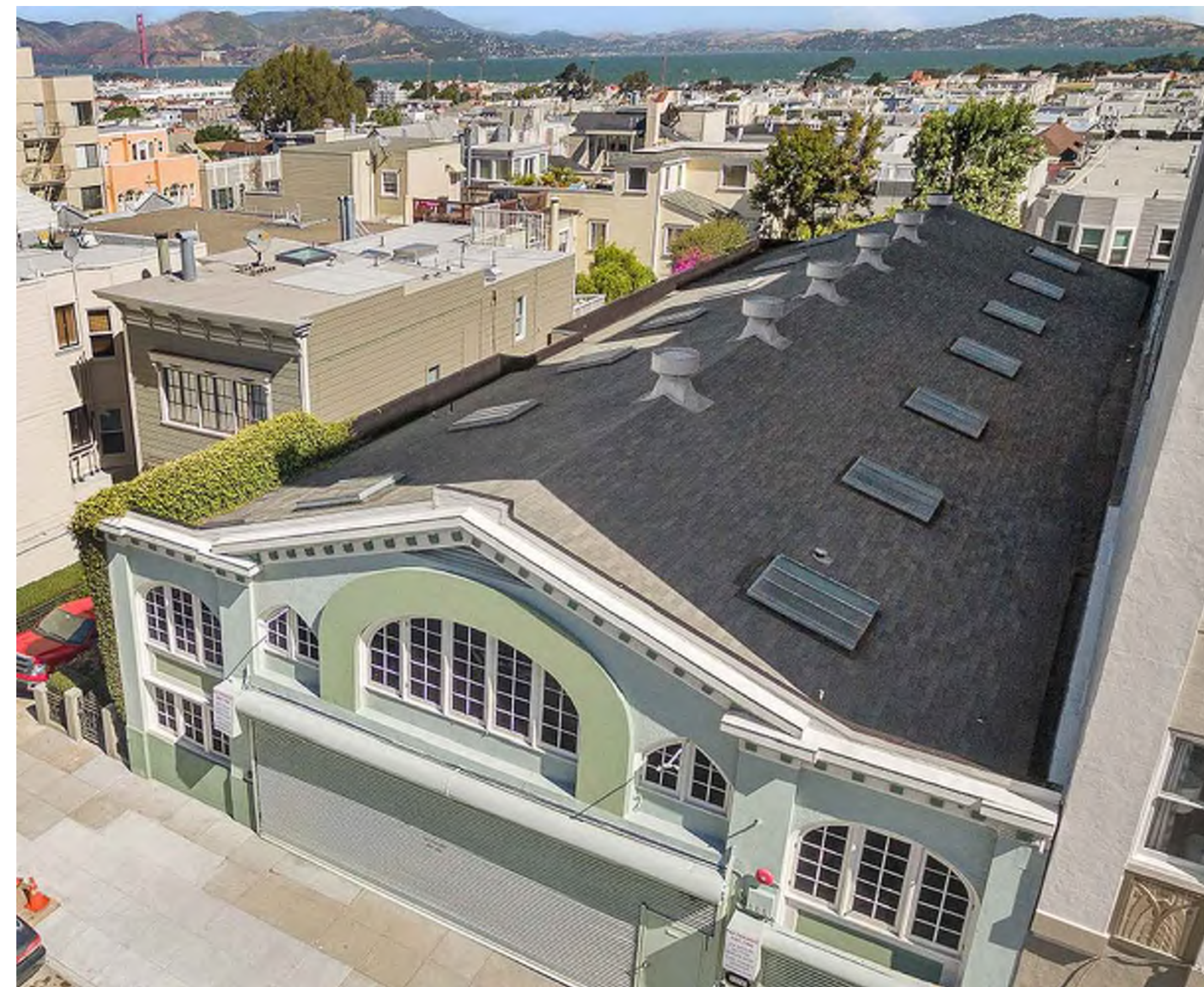
2 FRONT BUILDING FACADE & ROOF
