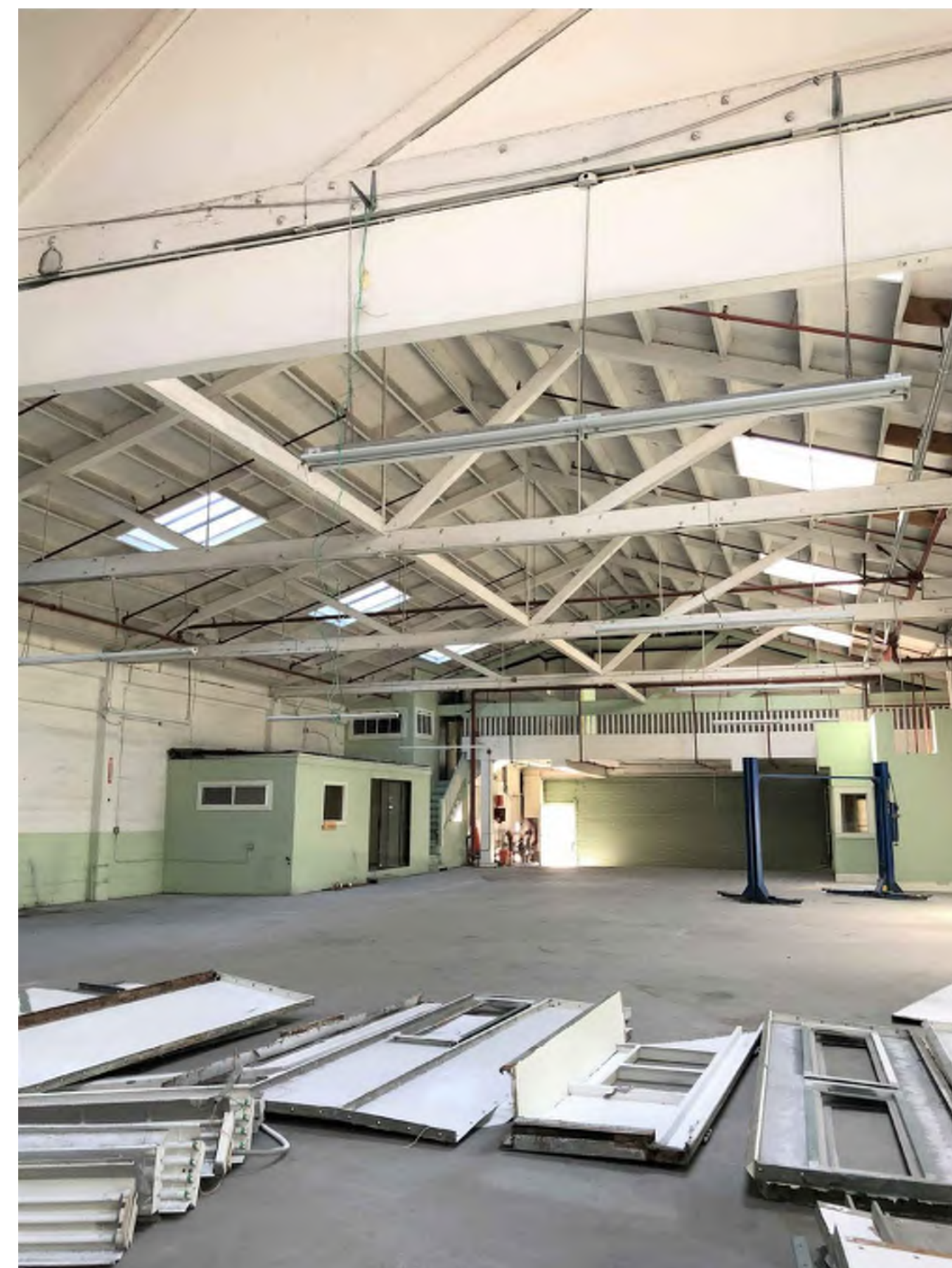
6 INTERIOR OF BUILDING AT FIRST FLOOR
