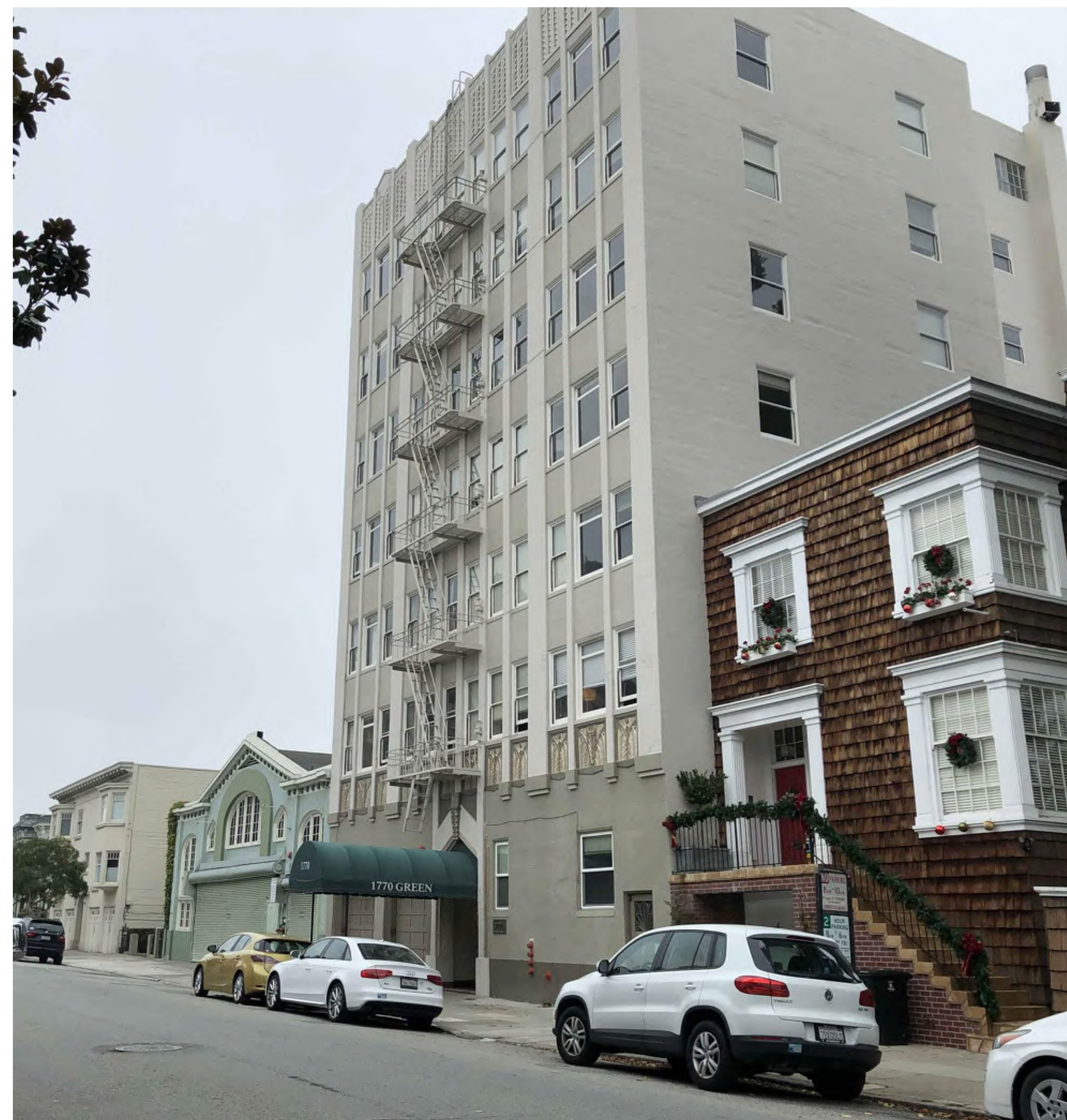
3 EXISTING VIEW 03 - VIEW FROM +/- 150 FEET SOUTHEAST OF SUBJECT PROPERTY
