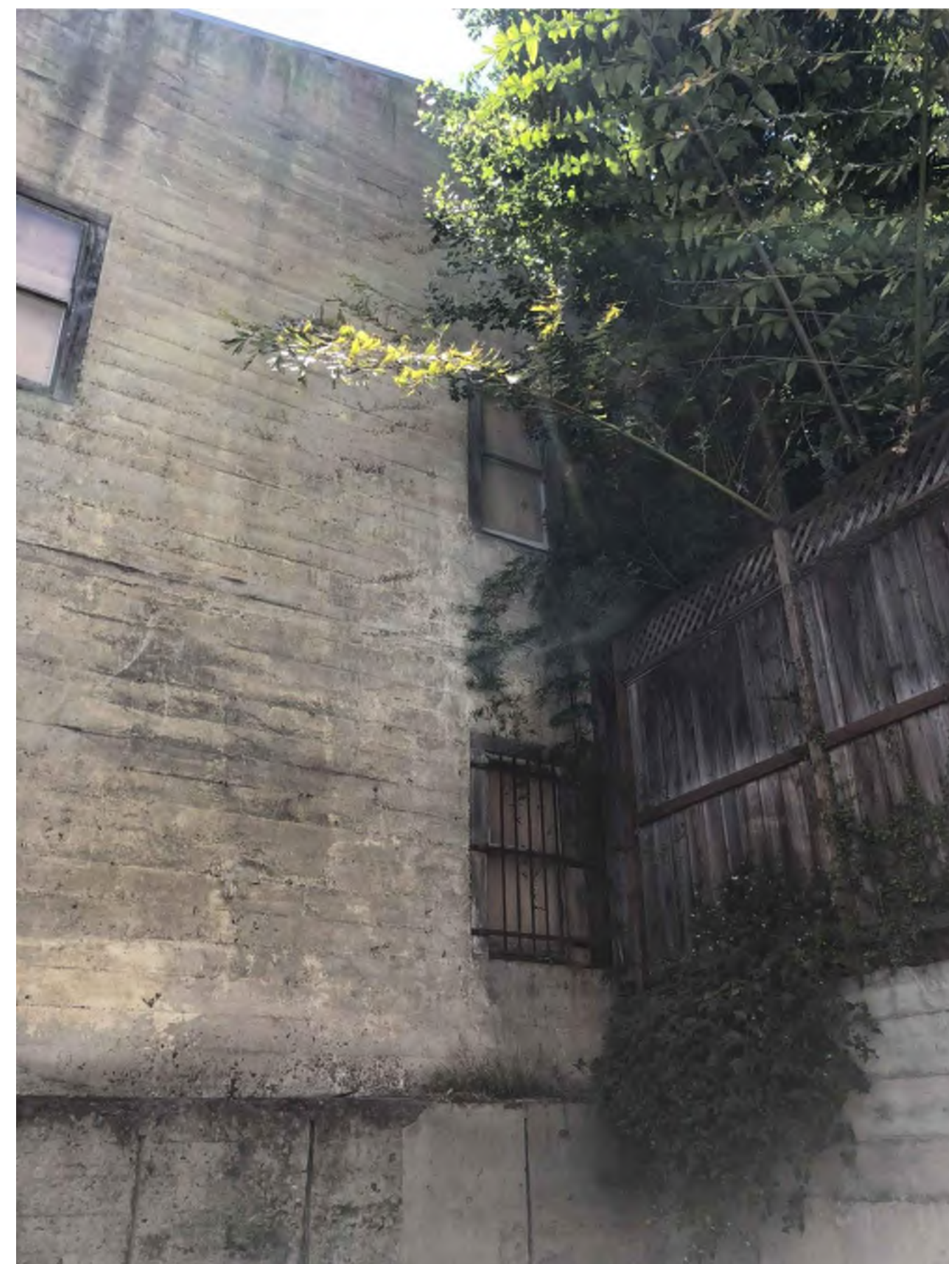
5 REAR FACADE BLOCKED BY ADJ. BLDG.
