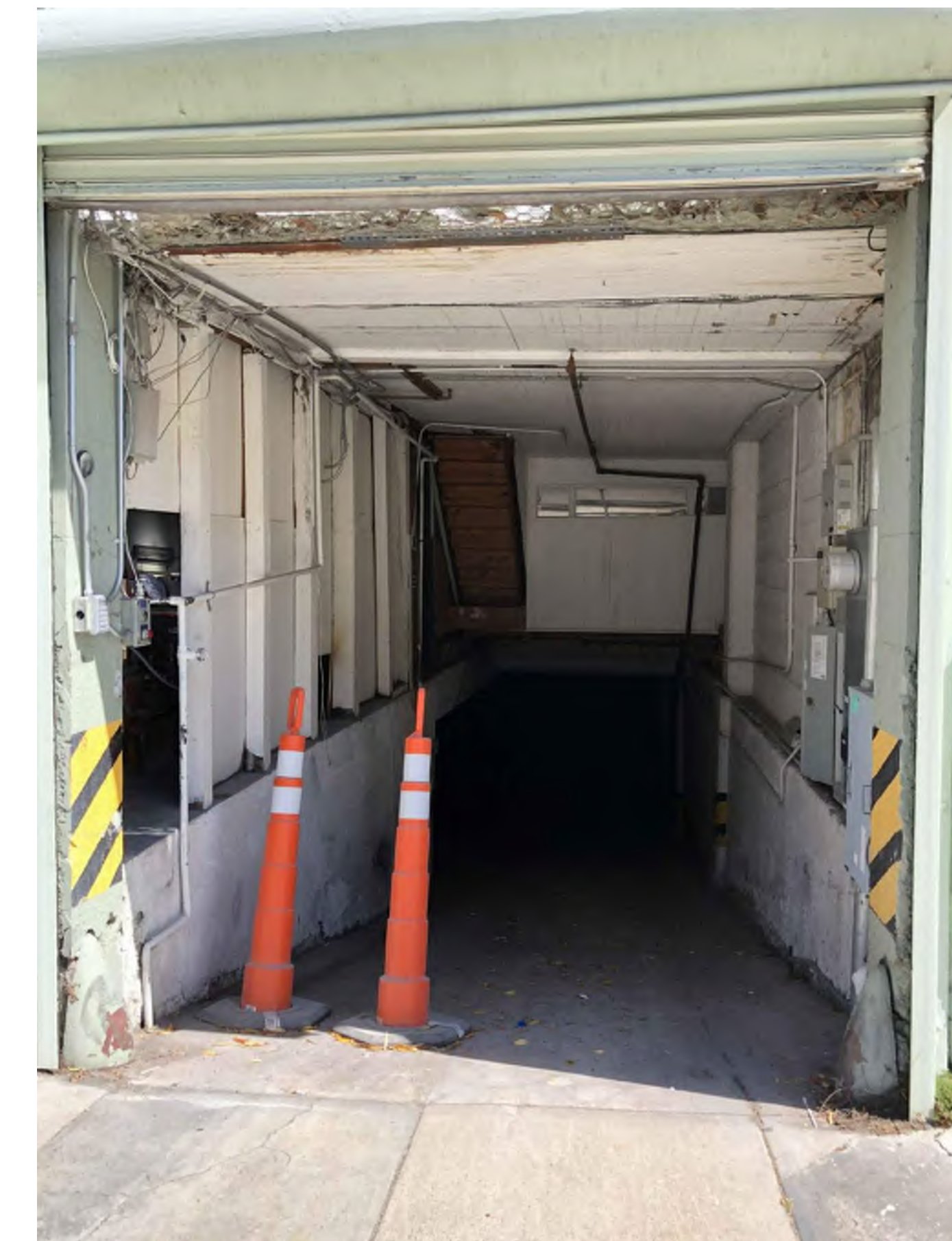
3 PARKING ENTRANCE AT FRONT FACADE
