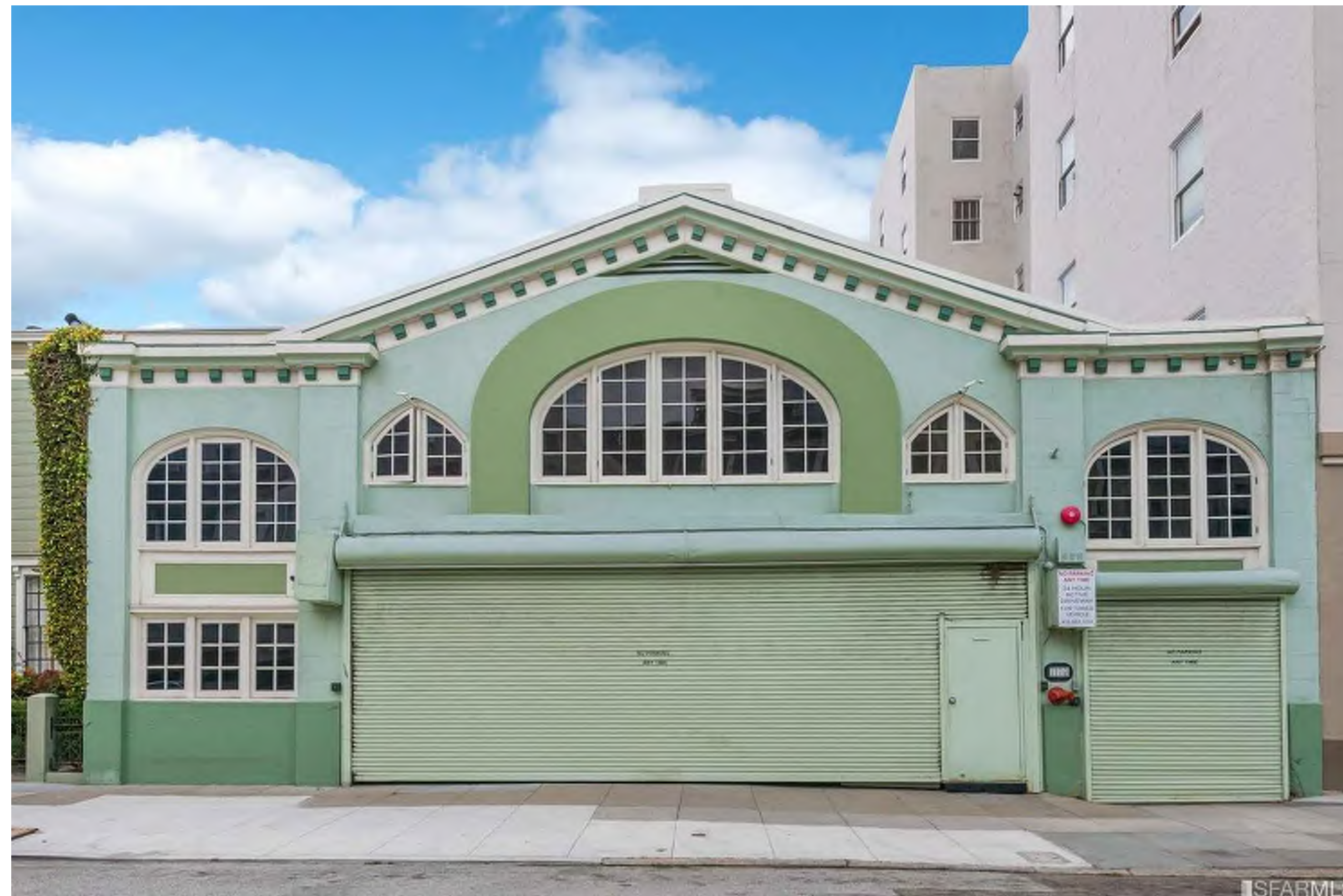
1 FRONT BUILDING FACADE
