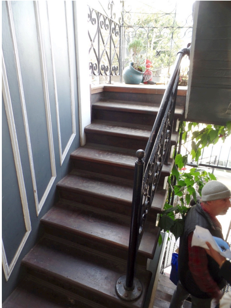
Figure 15: View of front entry stairs to third level. Note gap in baluster near landing (Garavaglia Architecture, 2023).
