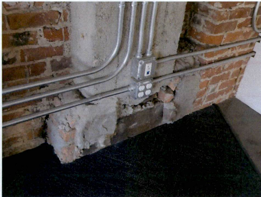
Photo 38: Exposed metal and damaged concrete coverage at column base -Third Floor.
