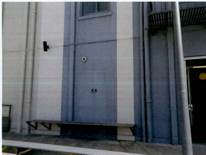
Photo I: View of cement plaster walls at north elevation. Cracking and deterioration of cement plaster visible. Looking south.
