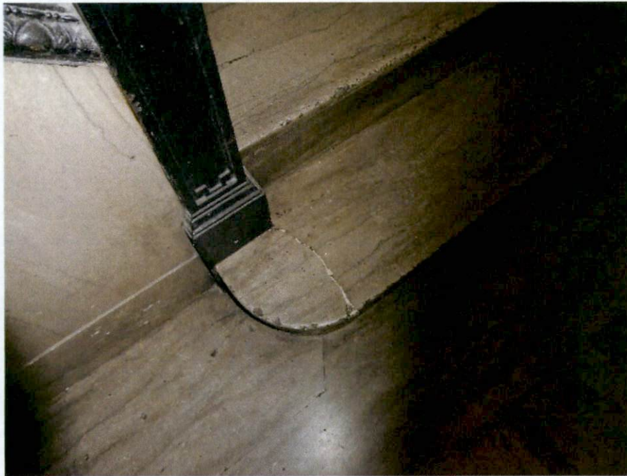
Photo 46: Cracked marble tread - Basement.
