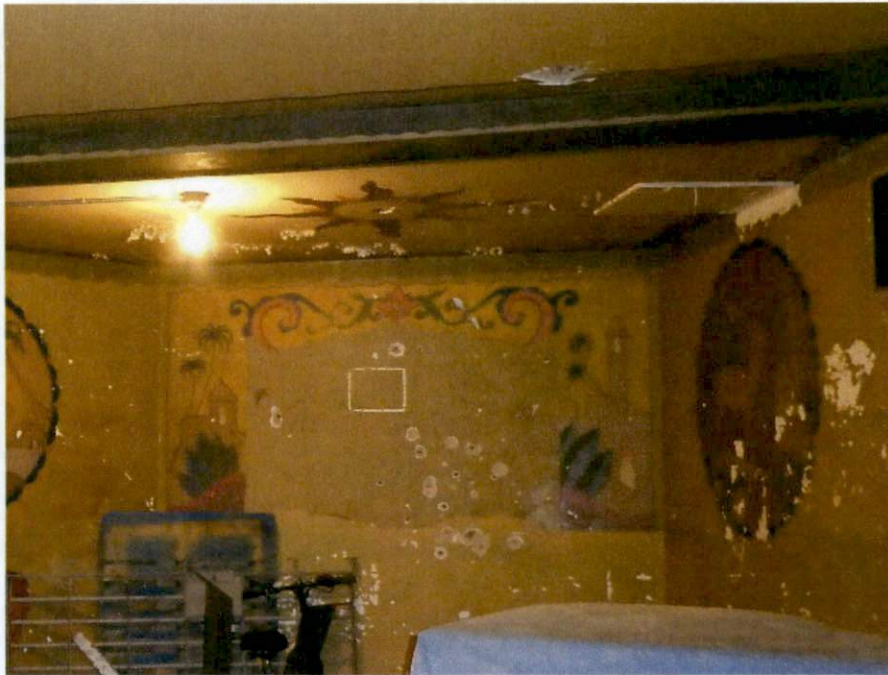
Photo 44: Murals on plaster walls with flaking paint and numerous holes.
