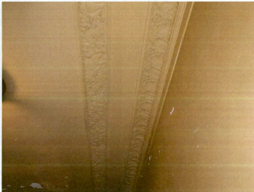
Photo 45: Original decorative crown molding and flaking paint in the lobby - Basement.
