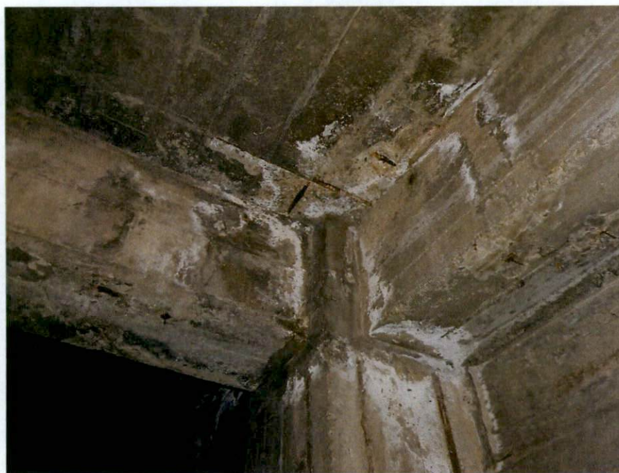
Photo HH: View of spalling, steel corrosion and efflorescence at mechanical attic 10 th level. Typical representation of conditions.
