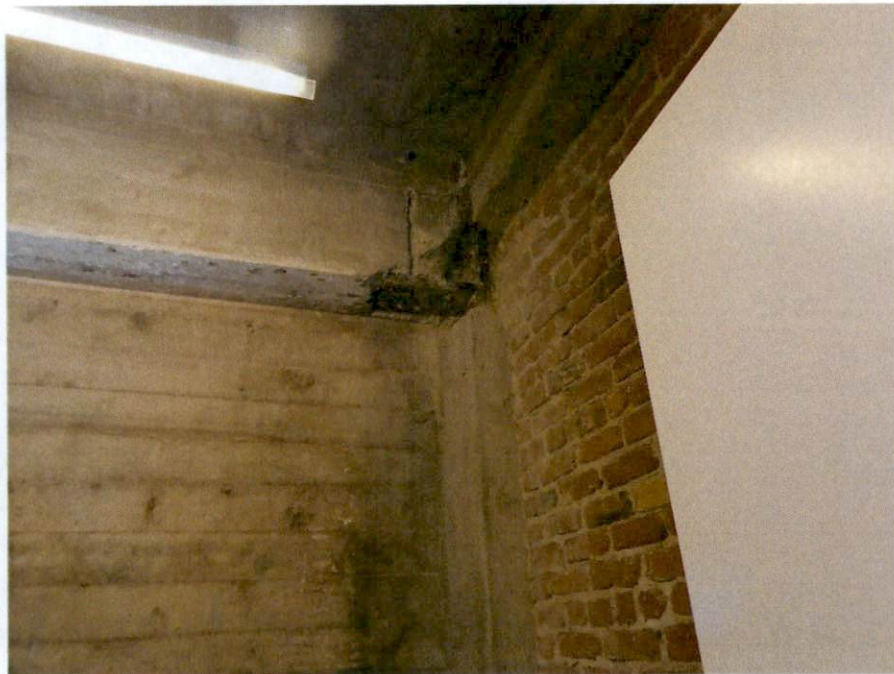
Photo Z: View of exposed steel at 5th level and cracked/ deteriorated concrete.
