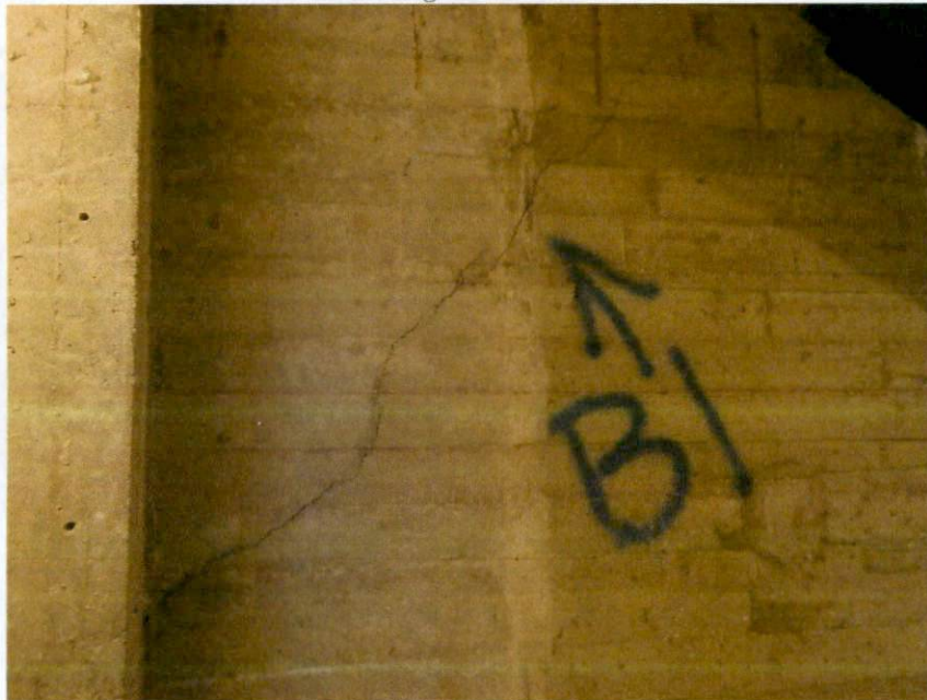
Photo 42: Example of crack in concrete wall at north stairwell - Third Floor.
