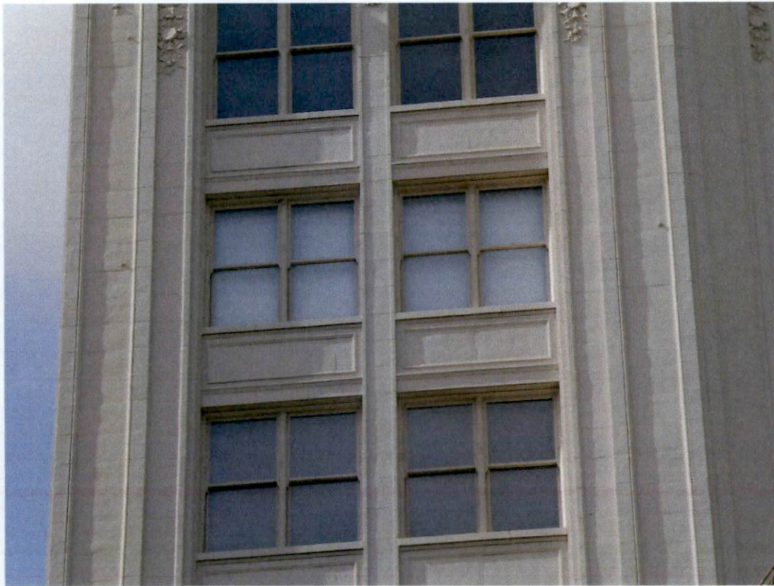
Photo 29. Example of replacement wood window sash in original frame – Market Street.
