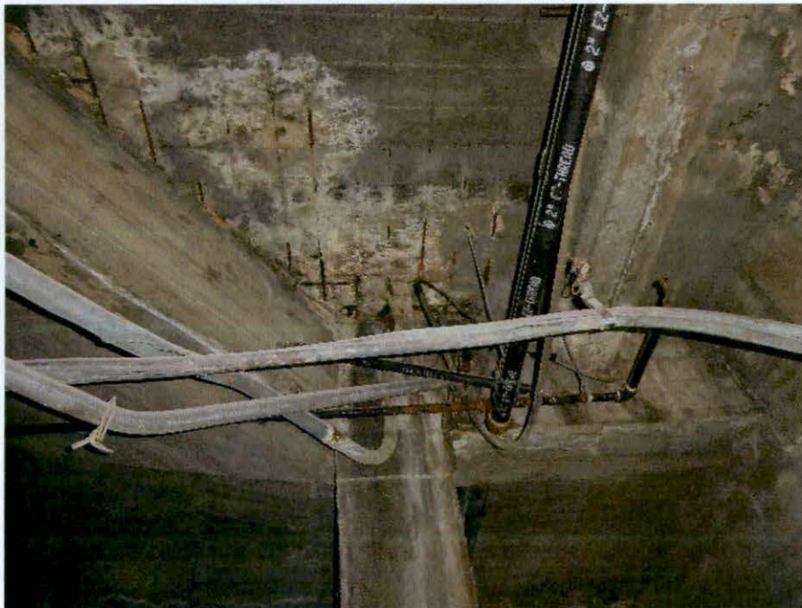
Photo 47: Deteriorated concrete and visible, rusting rebar overhead. Efflorescence is also present - Basement.
