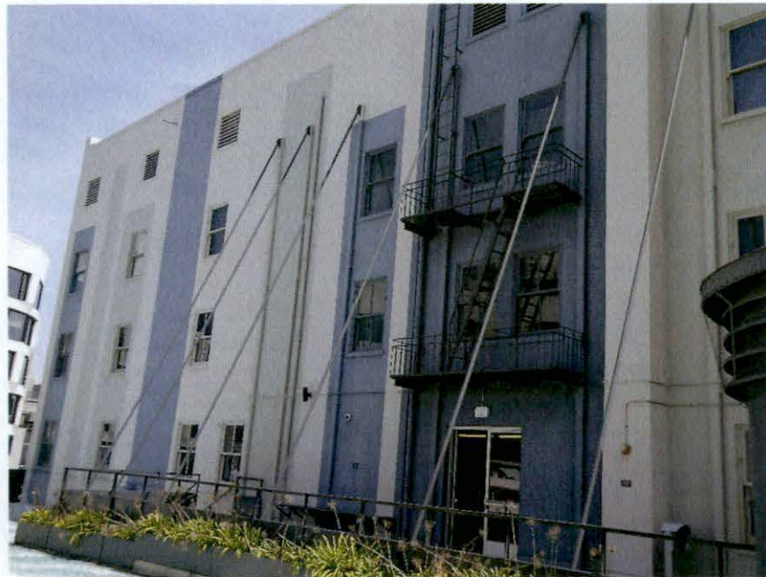
Photo H: View of metal fire escape on north elevation between 7th level and rooftop. Looking south.
