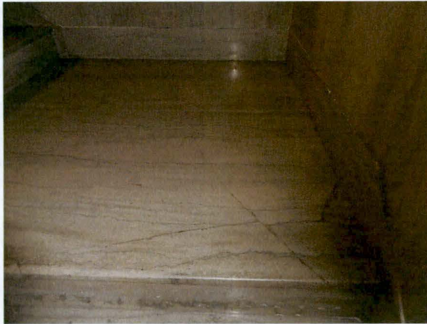
Photo 36: Example of horizontal cracks at marble stair landing - First Floor.
