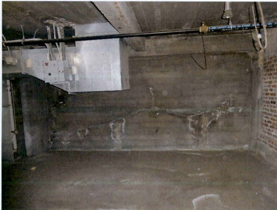
Photo 50: Horizontal cracking along exterior concrete wall - Tenth Floor.
