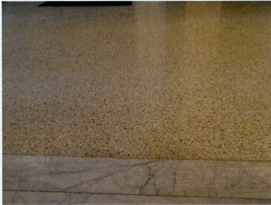
Photo 43: Original terrazzo and marble lobby flooring. Image is representative of typical material condition throughout interior lobbies – Second Floor.
