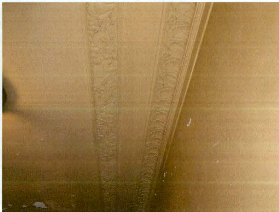
Photo 45: Original decorative crown molding and flaking paint in the lobby - Basement.
