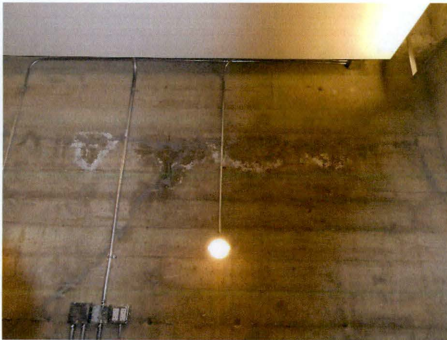
Photo 40: Example of efflorescence along crack in concrete wall - Ninth Floor.
