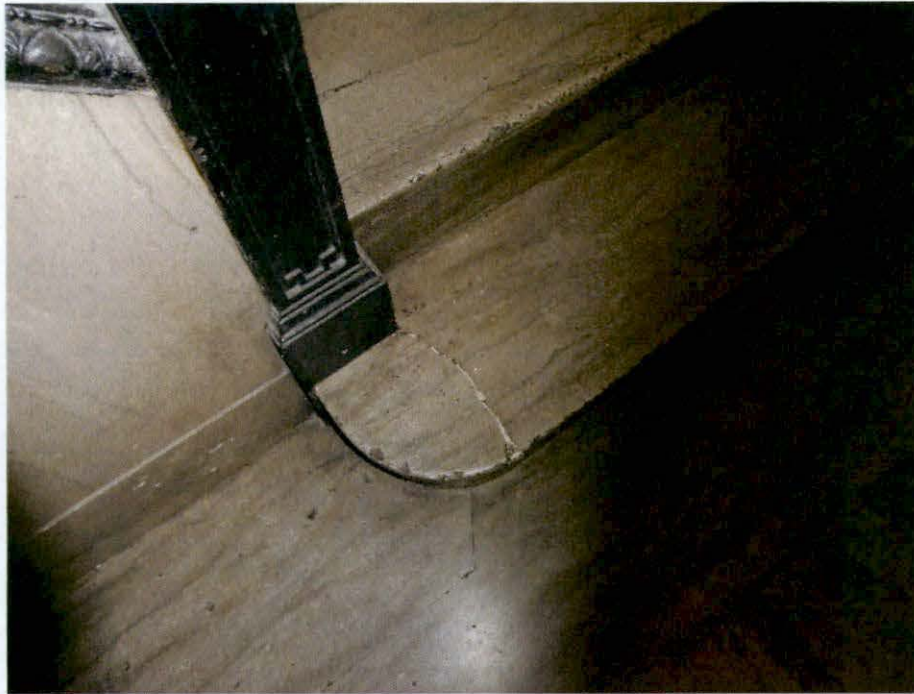
Photo 46: Cracked marble tread - Basement.
