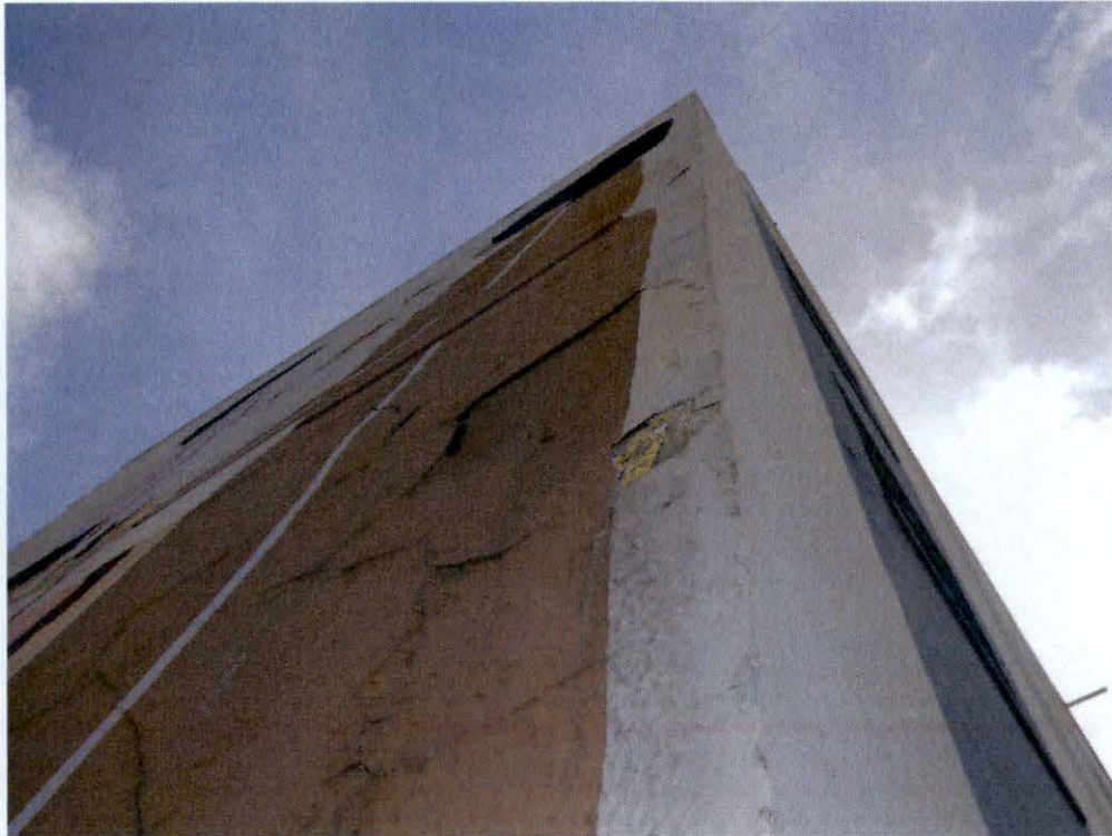
Photo 27: Detail showing delamination and peeling paint on cement plaster stucco – East Façade.
