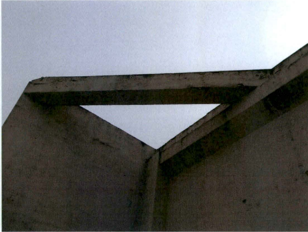
Photo 35: Cracks to parapet wall, lateral bracing at original sign location - Roof.
