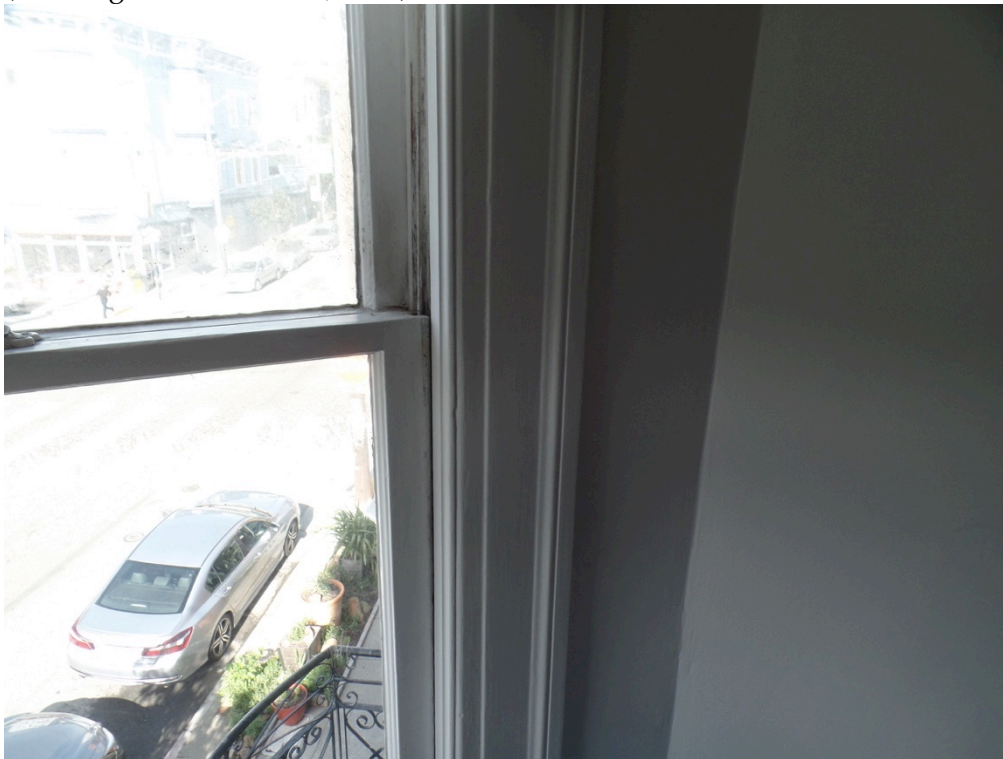
Figure 18: Interior view of front bay window in Unit 152A. Note damage at jamb and lower stile (Garavaglia Architecture, 2023).
