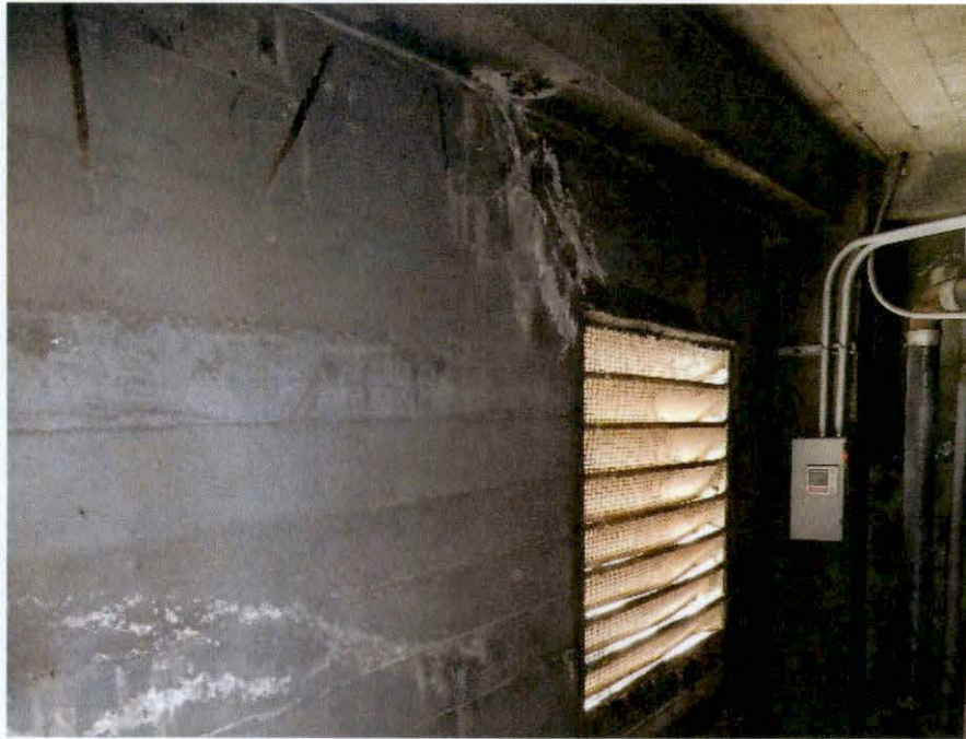
Photo 49: Cracking and efflorescence at opening in concrete for mechanical vent - Tenth Floor.
