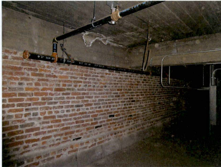
Photo FF: View of mechanical attic (tenth level) along interior of primary façade. Conditions of brick wall and efflorescence at concrete roof deck are typical throughout level.
