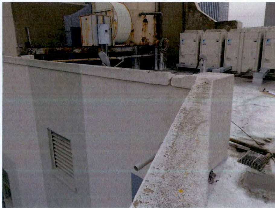
Photo 33: Cracking in cement plaster - Roof.
