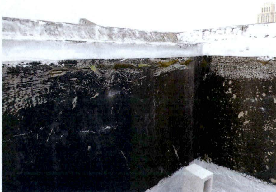
Photo 31: Parapet wall biological growth and cracking - Roof.
