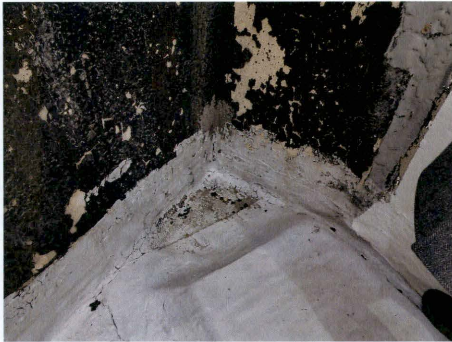
Photo 32: Failure at vertical parapet membrane – Roof.
