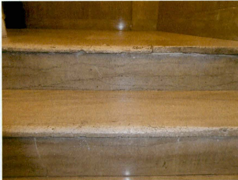
Photo V: Detail view showing damage to marble stairs between 1 st and 2 nd levels.
