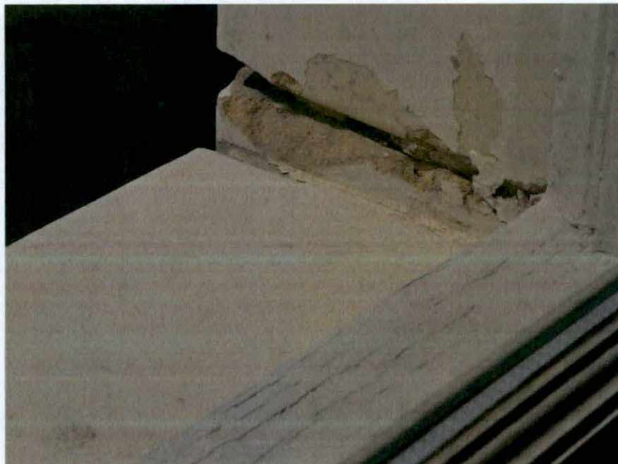
Photo 23: Example of missing and damaged mortar, paint delamination, and eroded terra cotta as well as splitting wood at the windowsill. Also visible is the original terra cotta glazing which is currently overcoated in paint - Market Street.
