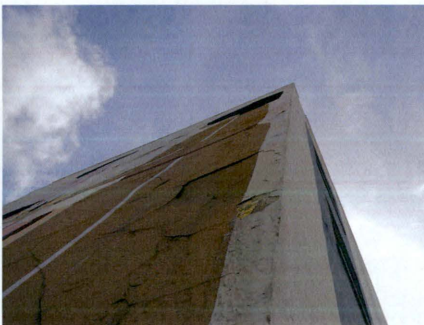
Photo M: Detail view of east exterior elevation seen from 7 th level rooftop looking southwest. Cement plaster and paint are spalling.
