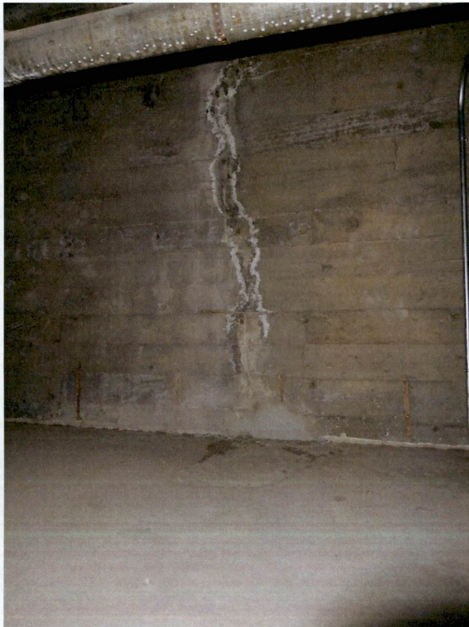
Photo 53: Vertical crack at concrete wall – Tenth Floor.
