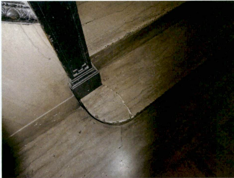
Photo 46: Cracked marble tread - Basement.
