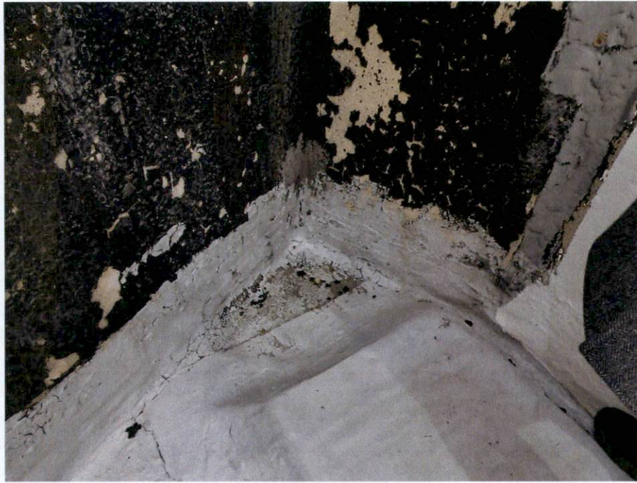
Photo 32: Failure at vertical parapet membrane – Roof.
