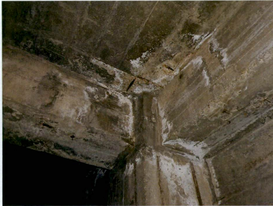
Photo HH: View of spalling, steel corrosion and efflorescence at mechanical attic 10 th level. Typical representation of conditions.
