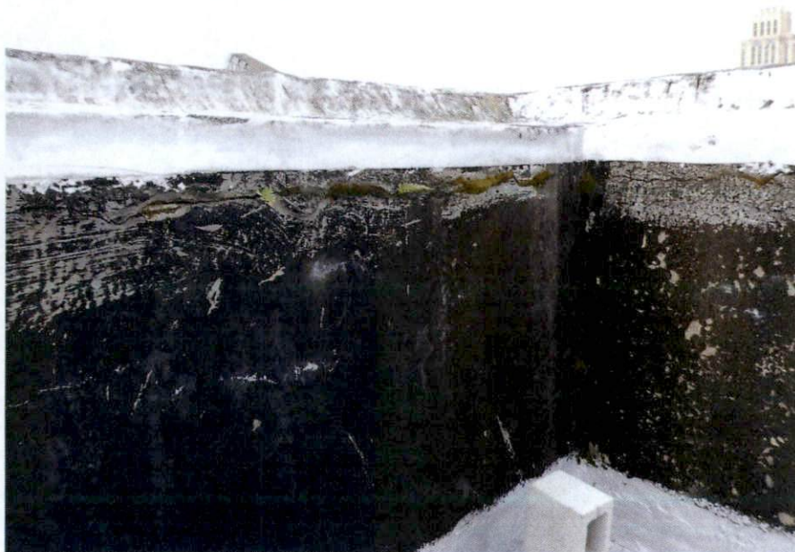
Photo 31: Parapet wall biological growth and cracking - Roof.
