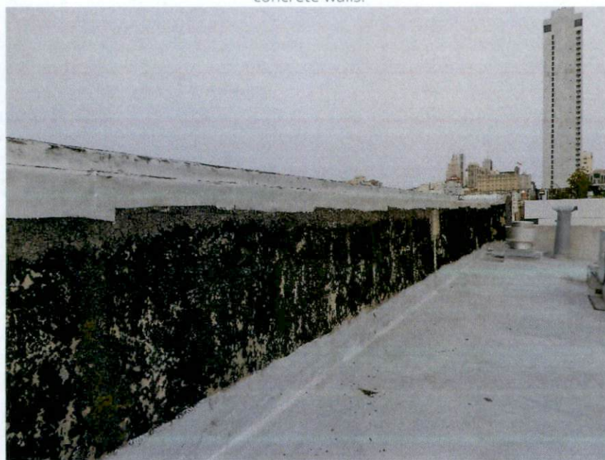
Photo O: View of parapet stem wall at roof level. Image shows damage to cement plaster and asphalt coating and biogrowth.
