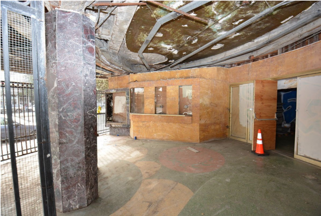
Terrazzo patterned flooring at the recessed corner entry.
