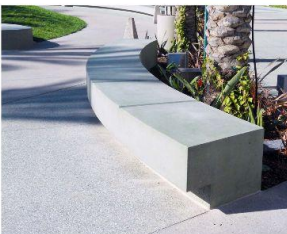
CONCRETE SEATWALL - FLAIN, SANDBLAST FINISH
