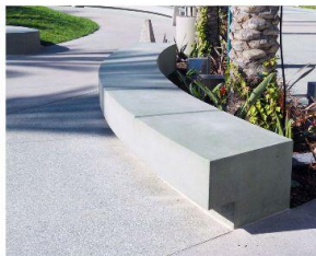
CONCRETE SEATWALL - FLAIN, SANDBLAST FINISH
