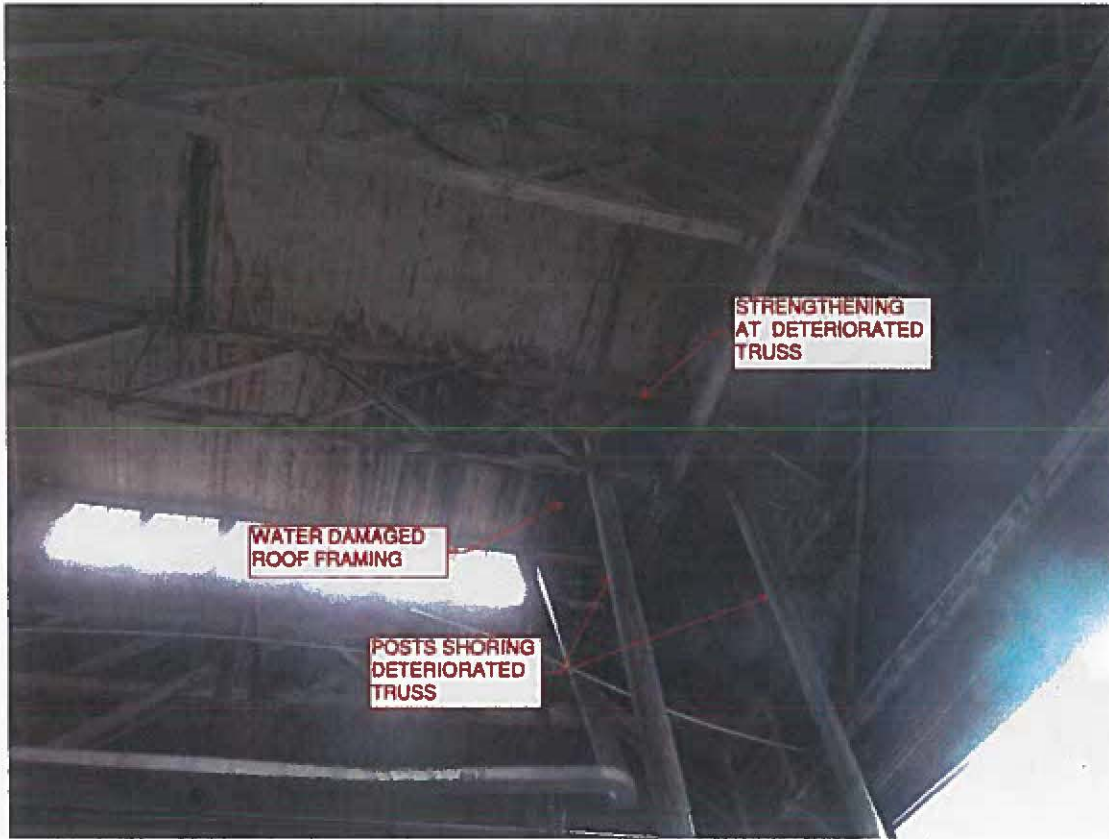
Figure 5 – Temporary shoring at damaged roof truss and framing, installed April 2017.
