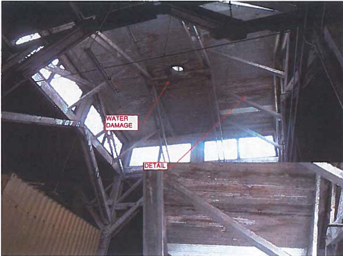
Figure 8 - Monitor water damage
