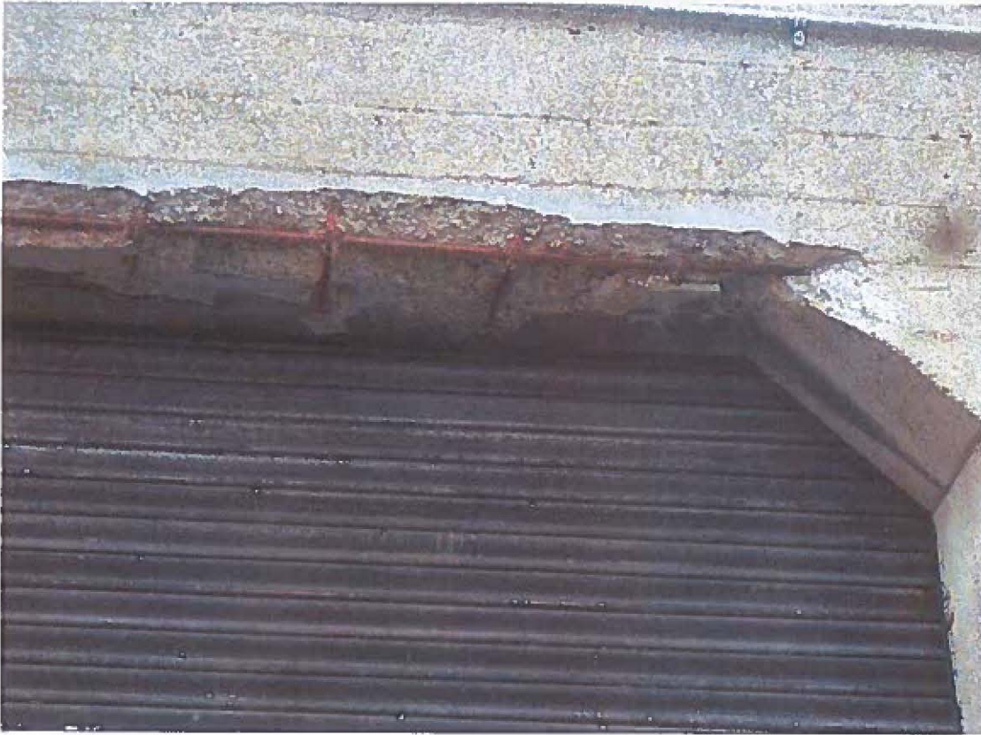
Figure 16 - Bay door header spalling. It appears a previous concrete repair has re-spalled.
