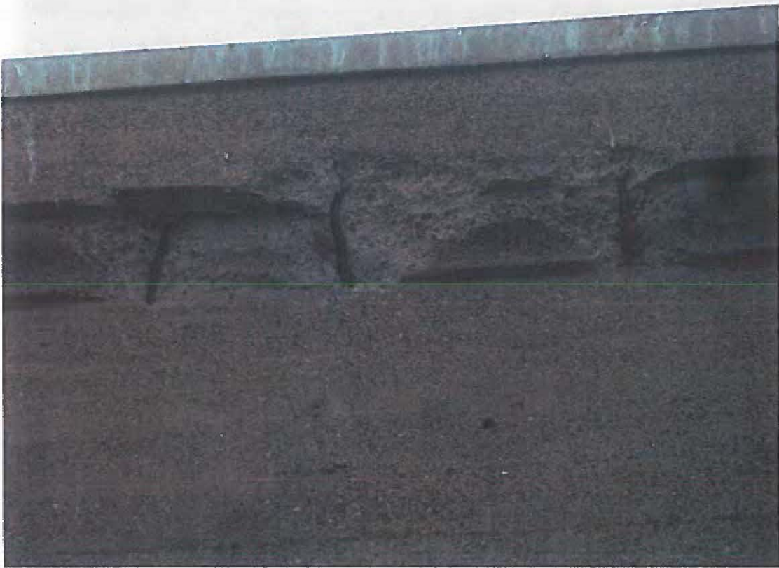
Figure 17 - Parapet spalling
