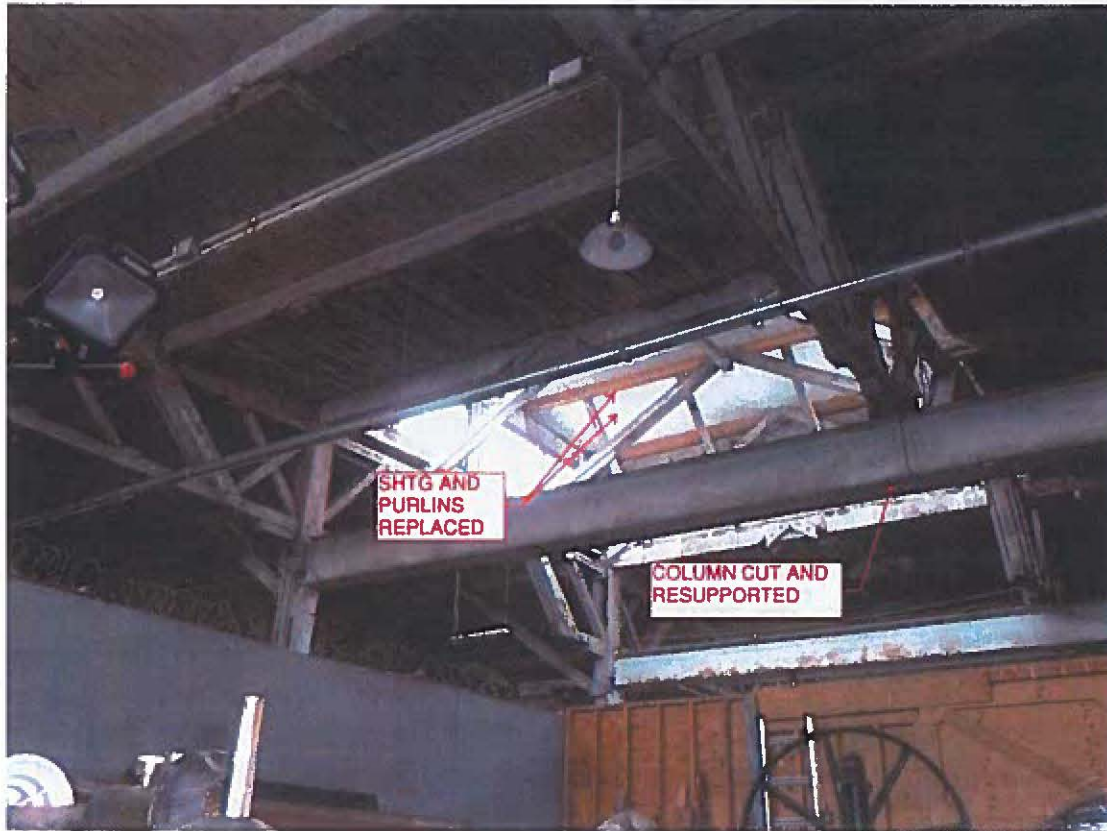
Figure 4 - Previously cut and resupported column. Previously replaced roof framing.
