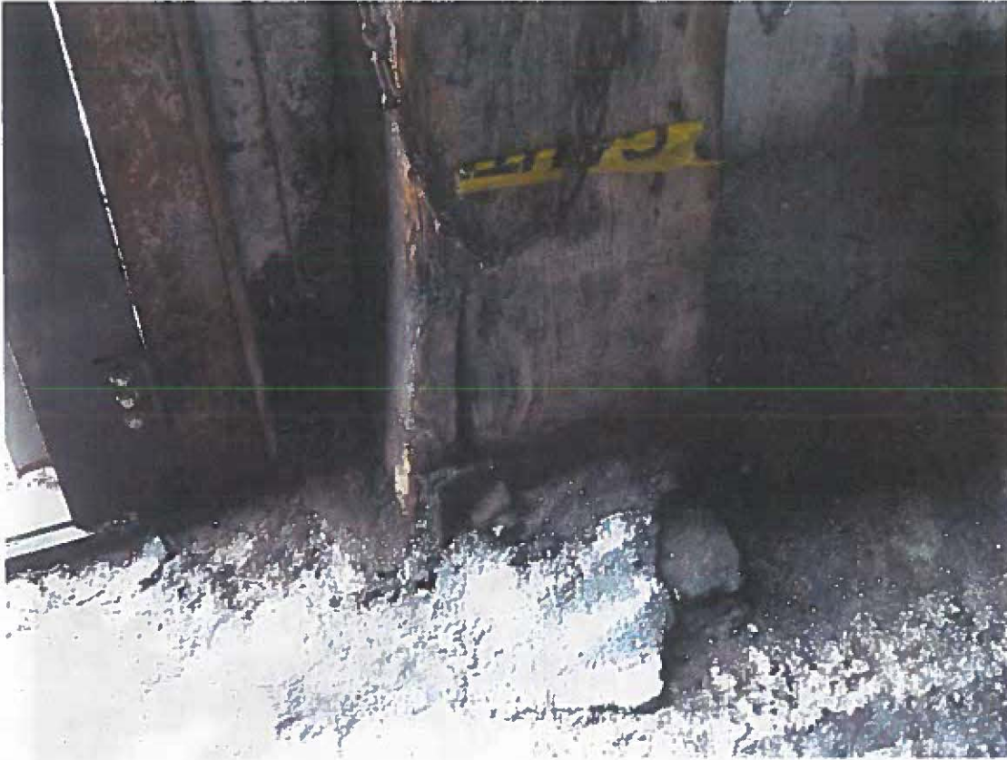
Figure 9 - Split column base at corroding base plate bolt next to bay door
