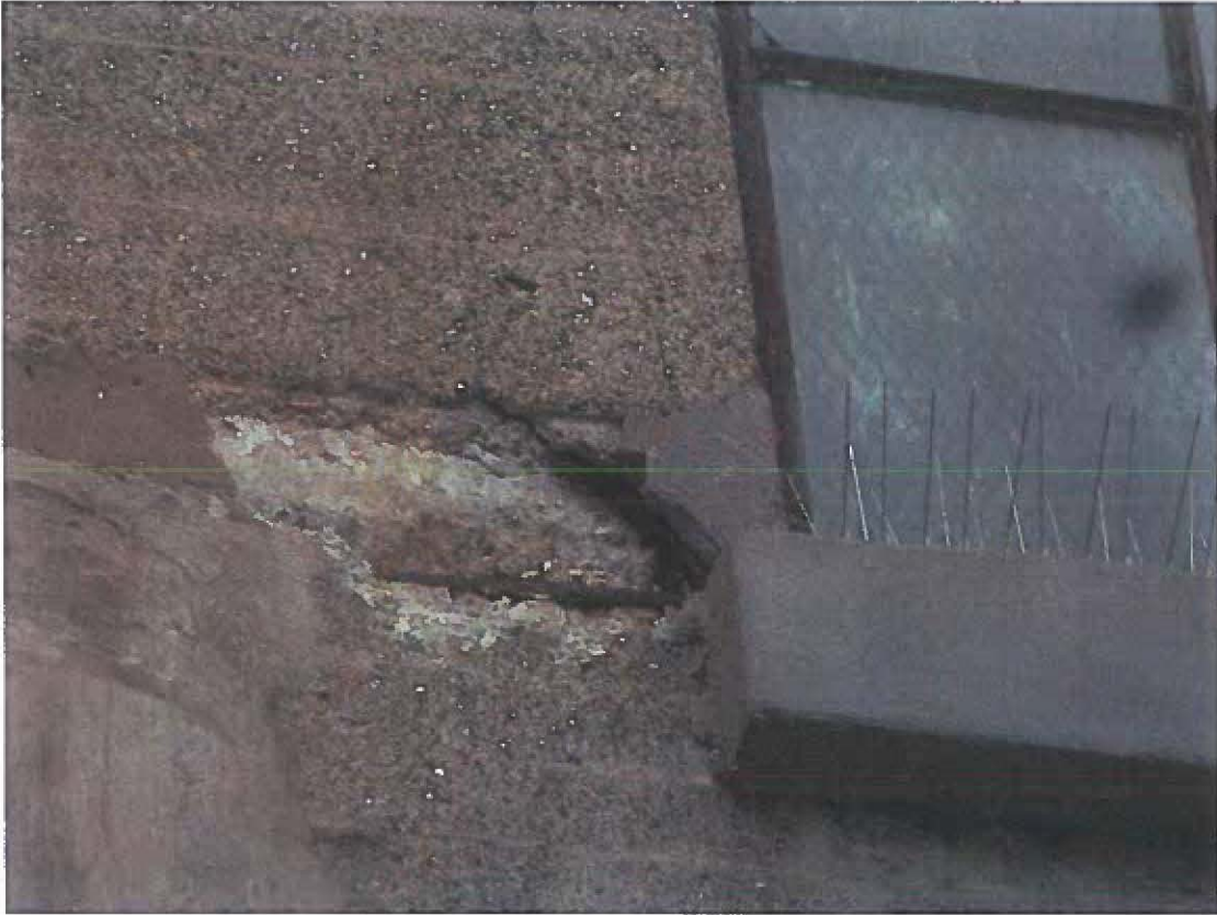
Figure 15 - Spalling at window corner
