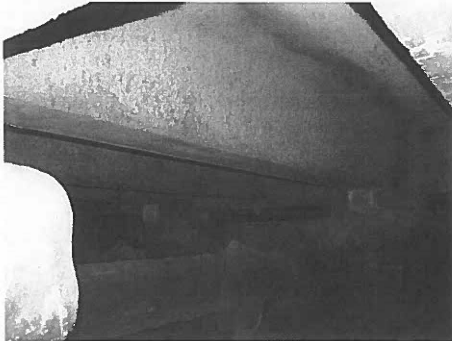
Figure 4 - Typical Shotcrete Beam Repair
