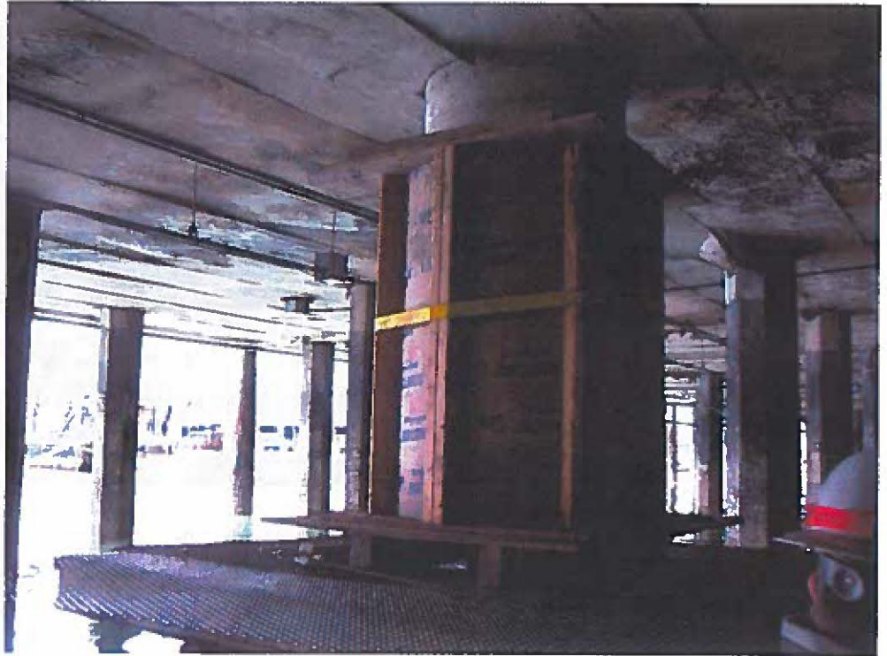
Figure 29 - Concrete Encasement Repair
