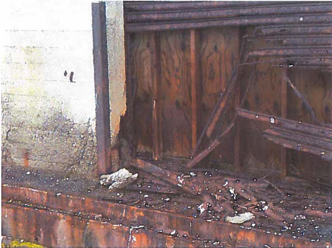
Figure 20 - Corrosion, spalling, and water intrusion at bay door along north apron.
