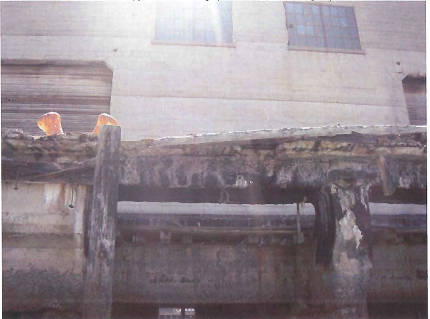
Photo 10. Spalling deck and corroded/exposed rebar
