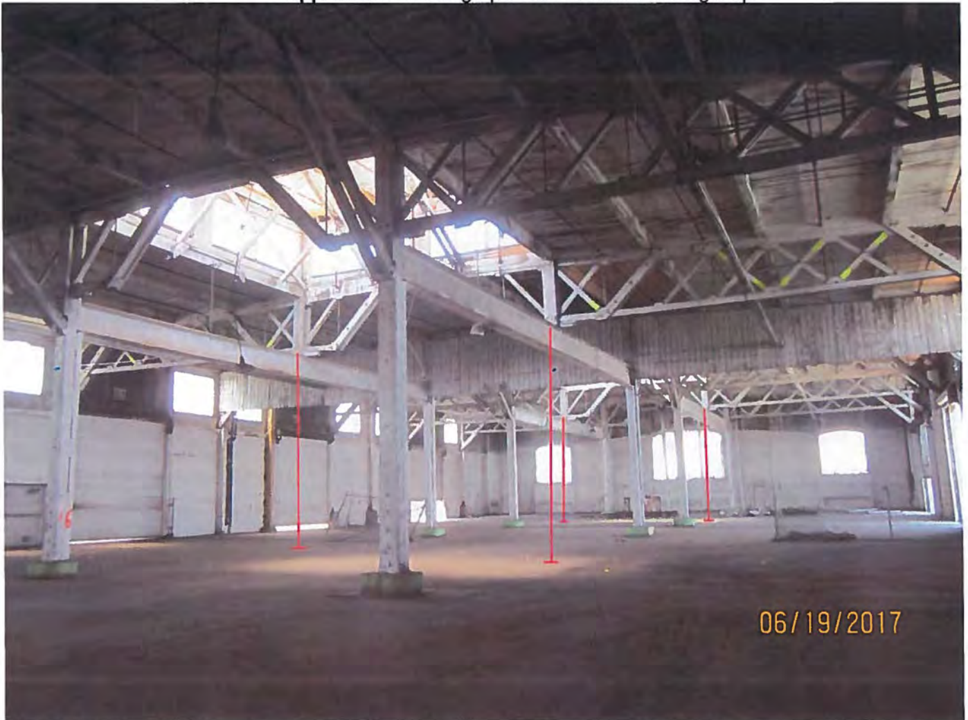
Photo 12. Steel beams and supplemental wood posts added in the past in order to remove original columns.
