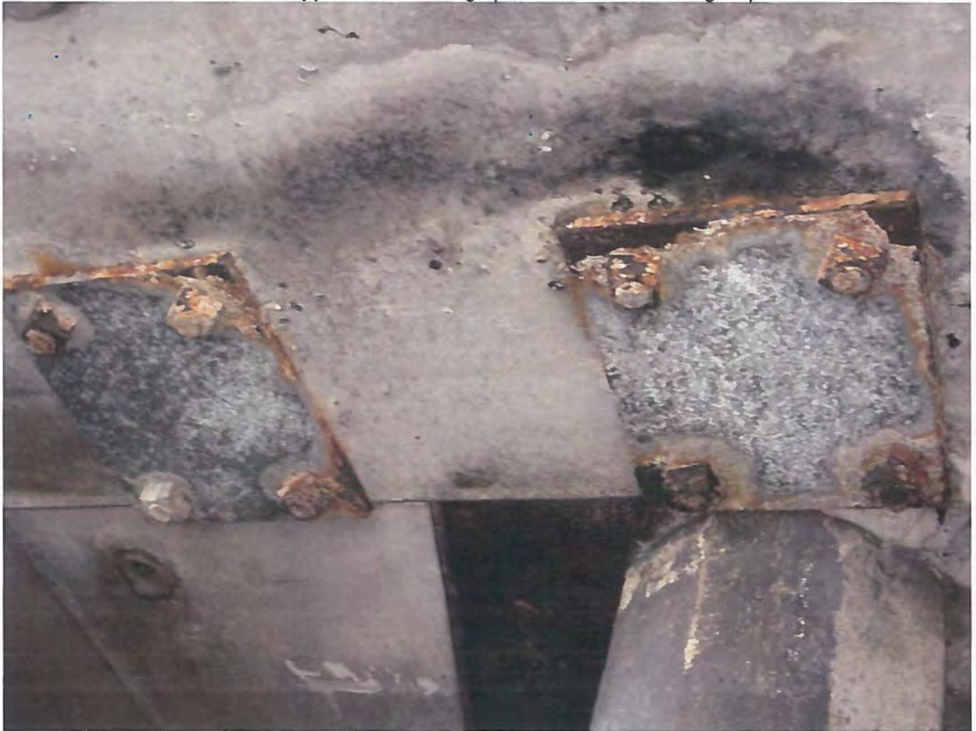
Photo 7. Corrosion on steel plates
