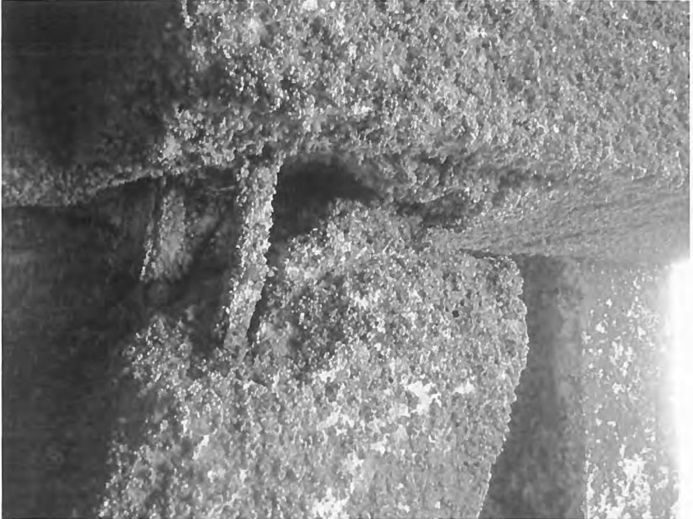
Photo 11. Close up of broken batter pile
