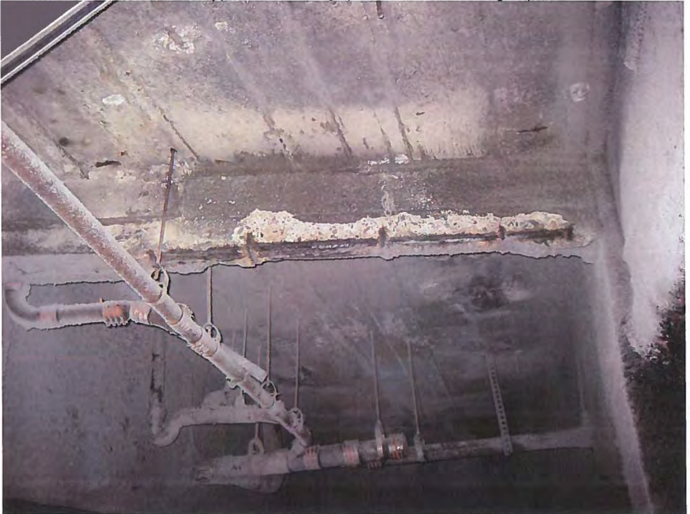
Photo 6. Spalling and exposed/corroded rebar on beam
