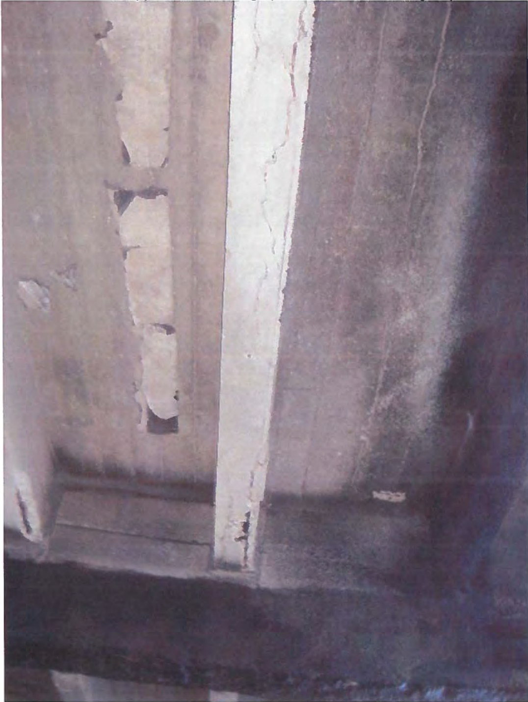
Photo 6. Concrete spalling at slab
