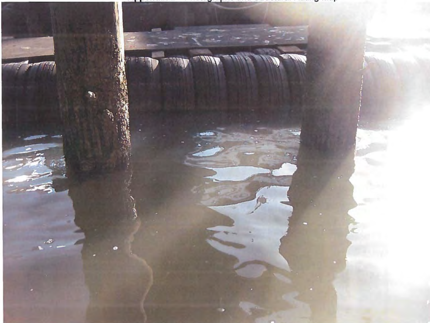
Photo 4. Deteriorated wood piles near metal deck
