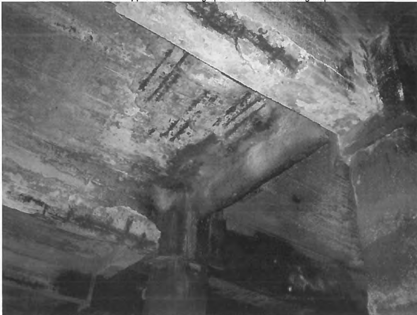
Photo 9. Spalling of concrete beams and slab
