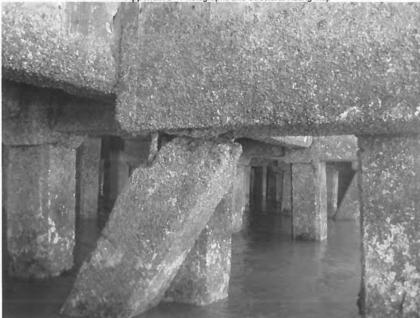
Photo 7. Broken batter pile
