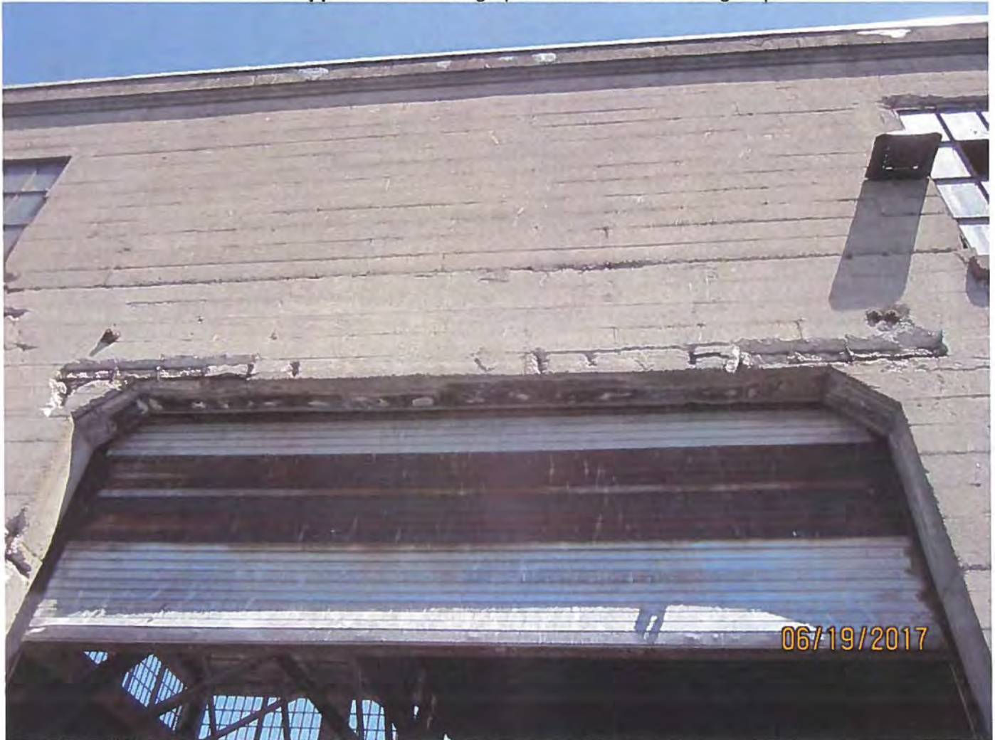
Photo 4. Spalls around roll-up door opening on north face wall. Repairs are planned as part of a future project.
