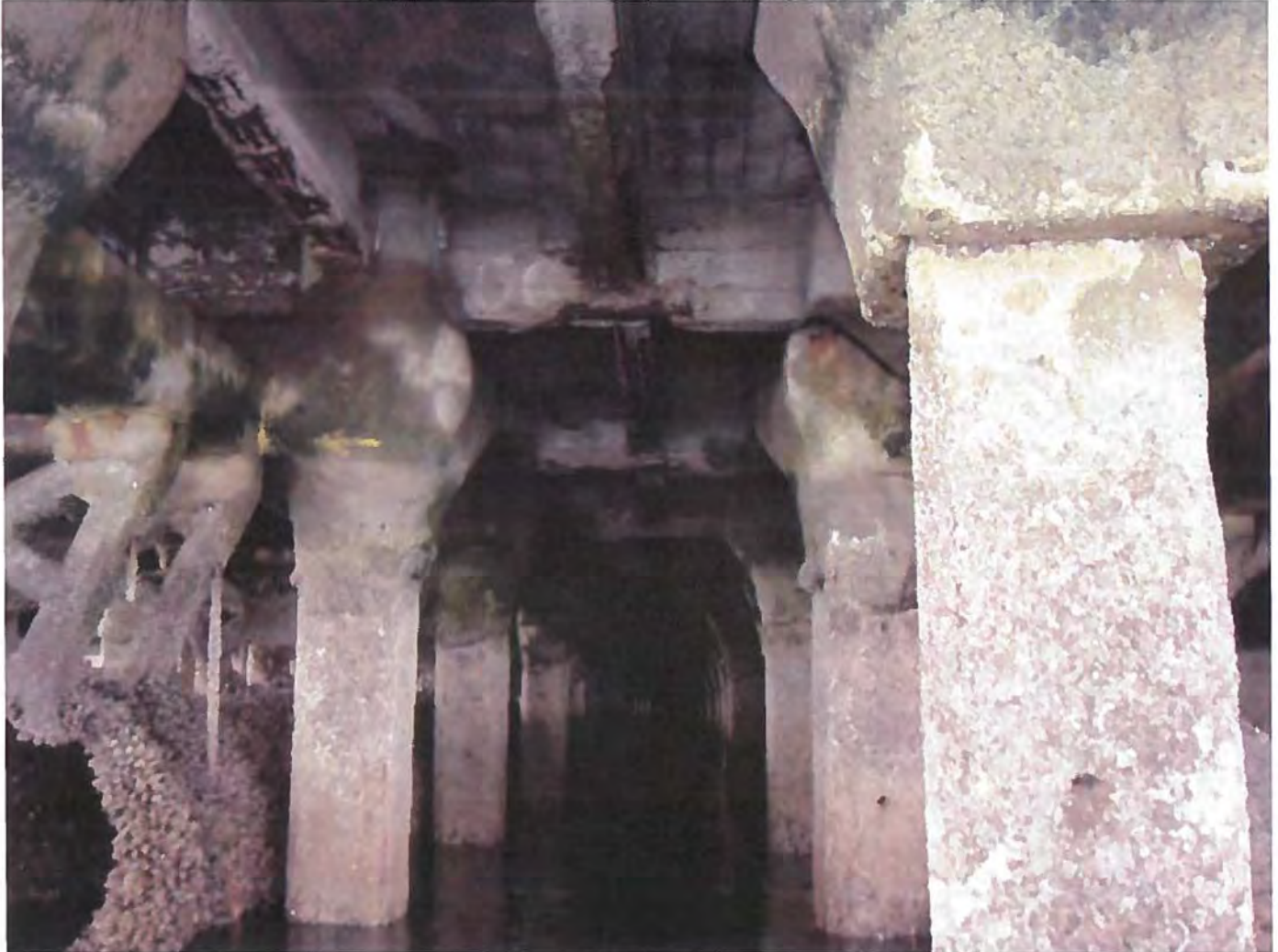
Photo 1. Spalled concrete beams and slabs above the outfalls under the Main Pier
