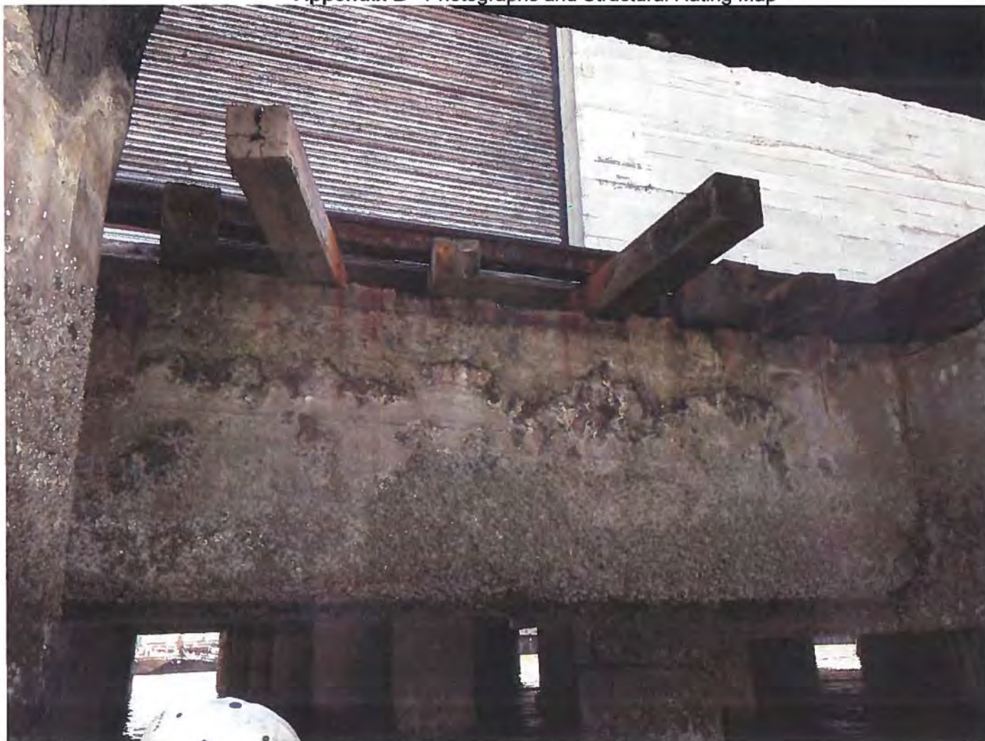
Photo 4. Hole in deck, hanging wood members
