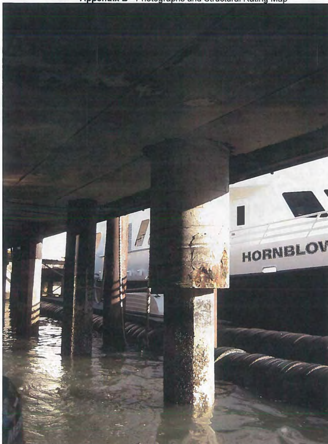
Photo 3. Crack on pile cap
