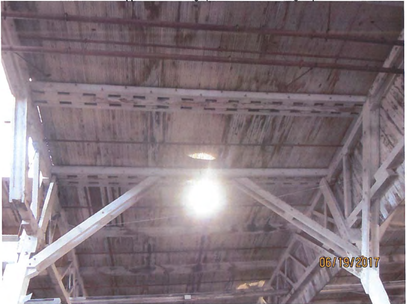
Photo 14. Wood roof beams strengthened in the past.
