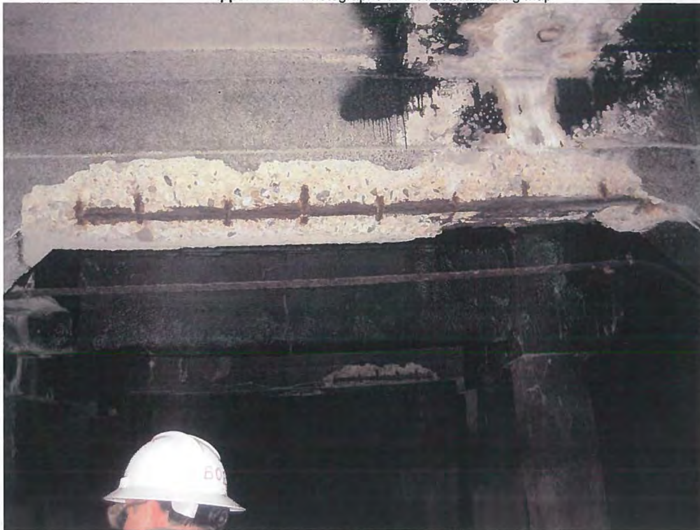
Photo 7. Spalling and exposed/corroded rebar at beam
