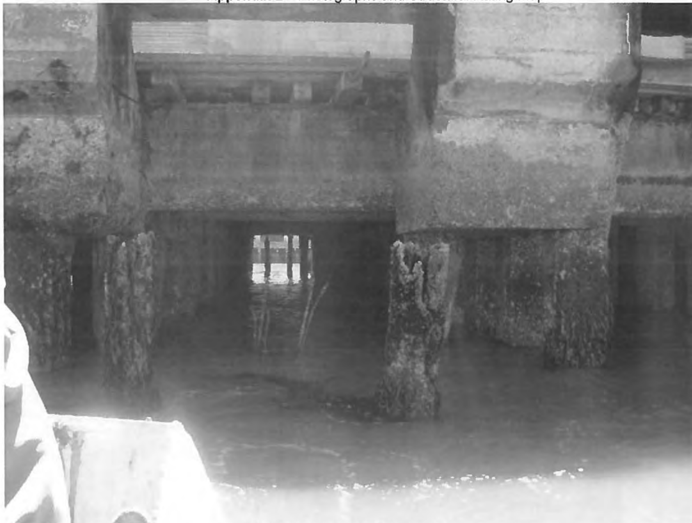
Photo 5. Deteriorated fender piles
