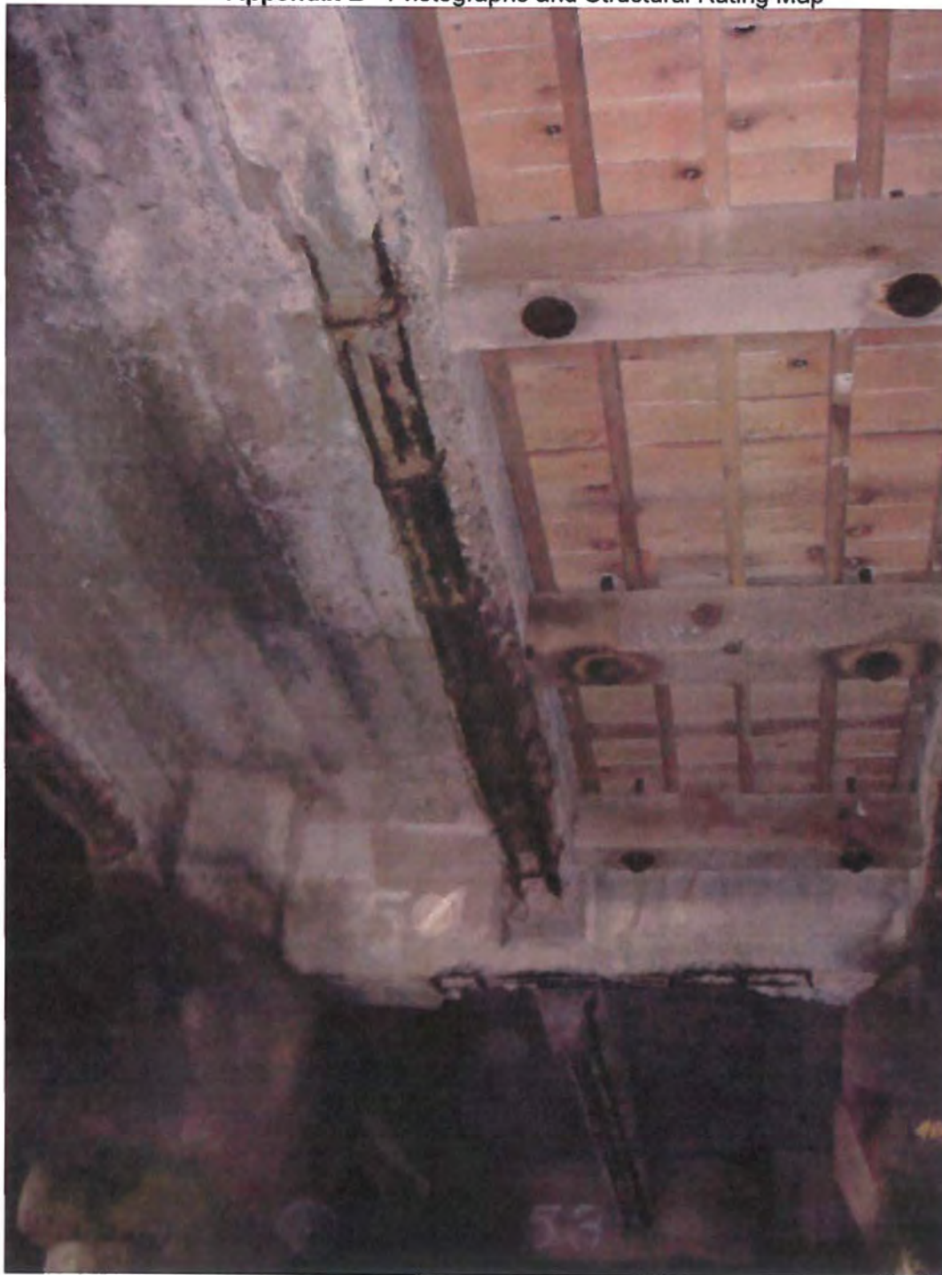
Photo 3. Concrete spalling, typical
