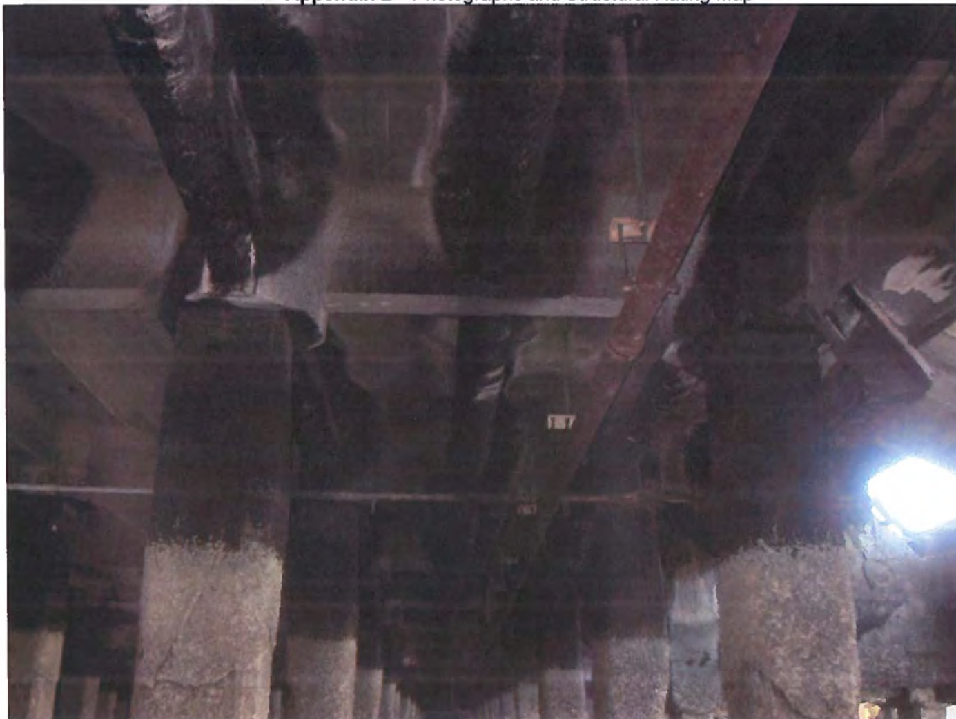
Photo 2. Gunite on concrete framing
