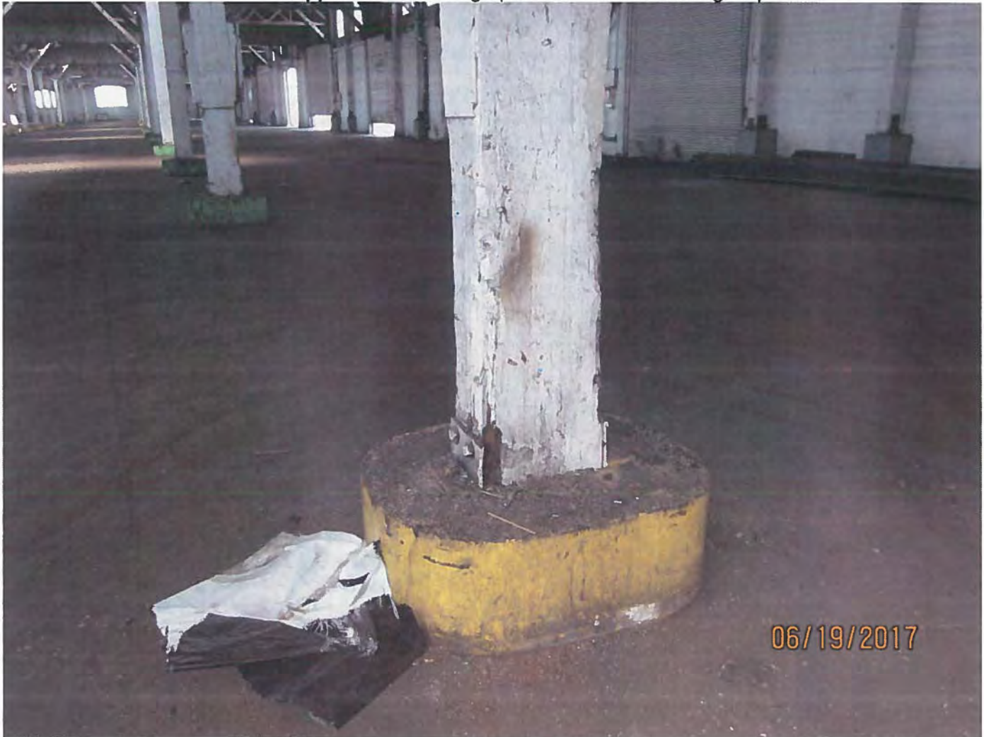
Photo 15. Interior wood columns on raised footings. Less susceptible to dry rot, but some have minor damage from vehicle impact.
