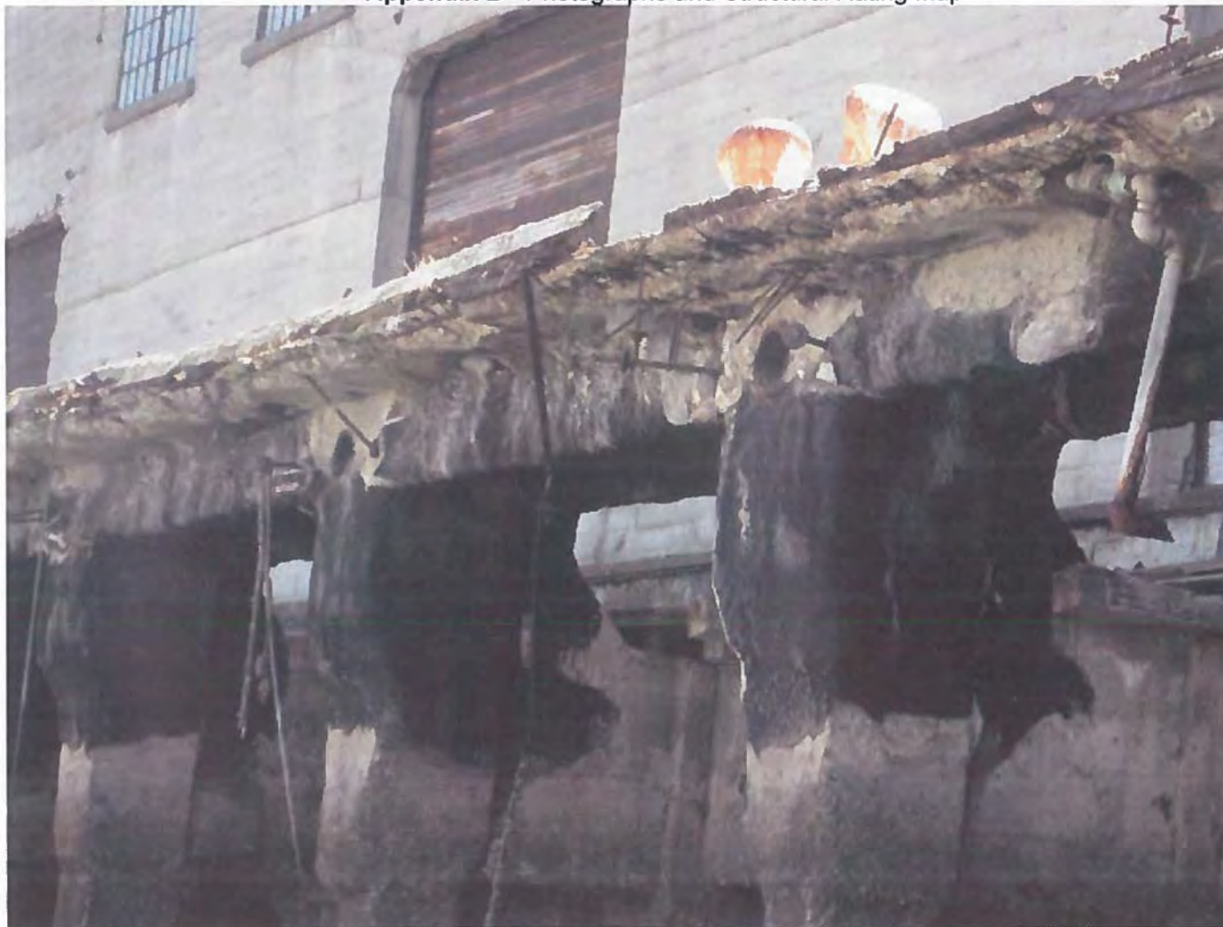
Photo 9. Deteriorated deck
