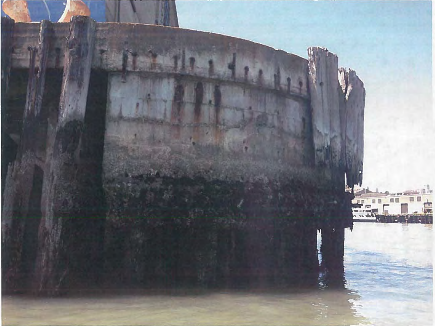
Photo 3. Deteriorated wood piles at pier corner
