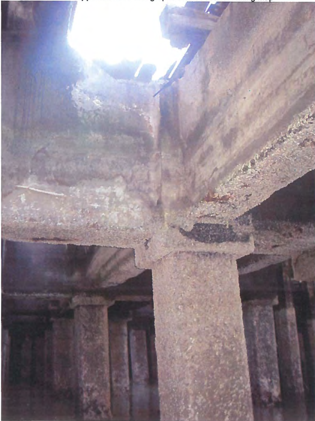
Photo 4. Hole at deck
