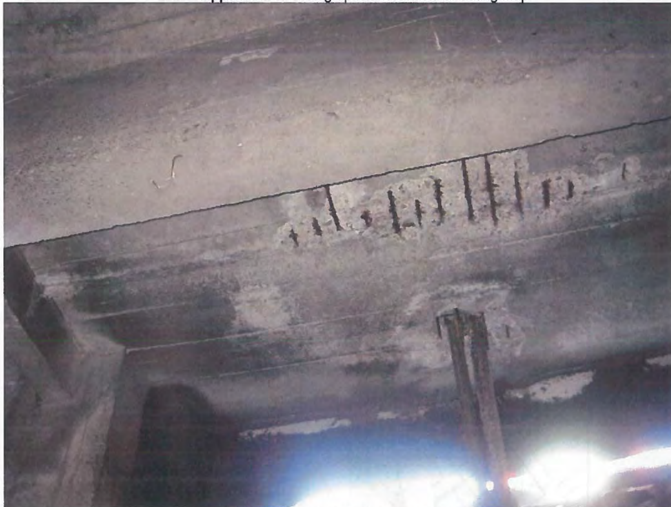
Photo 1. Spalling and corroded/exposed rebar at slab
