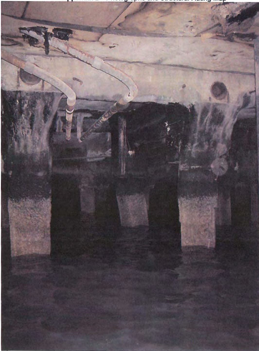
Photo 2. Piles out-of-plumb
