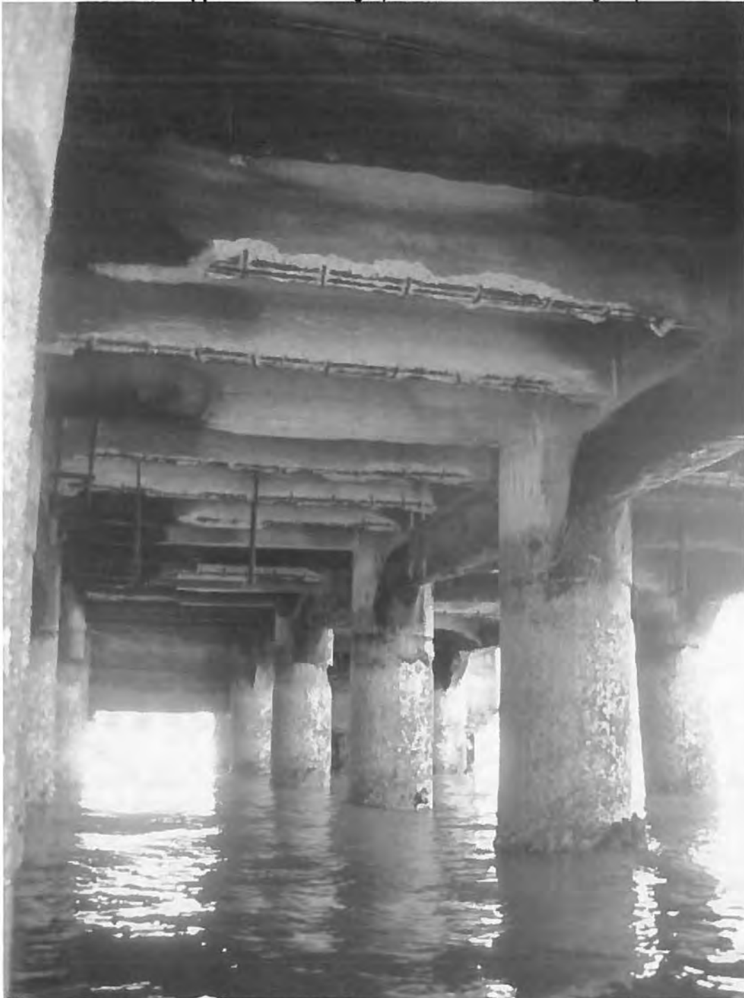
Photo 5. Spalling of concrete beam with exposed/corroded rebar
