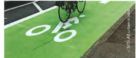
Standard asphalt with green surfacing
