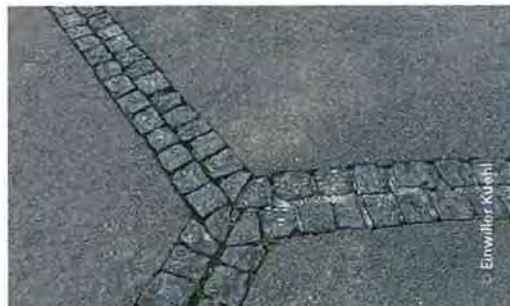
Asphalt with frame
