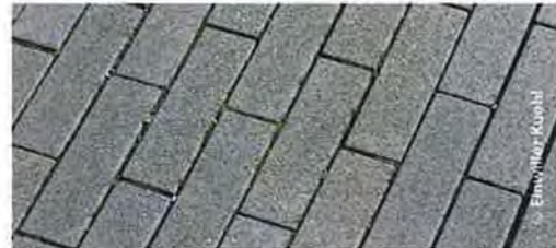
Concrete unit pavers
