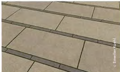
Pre-cast concrete and pre-cast permeable unit-pavers
