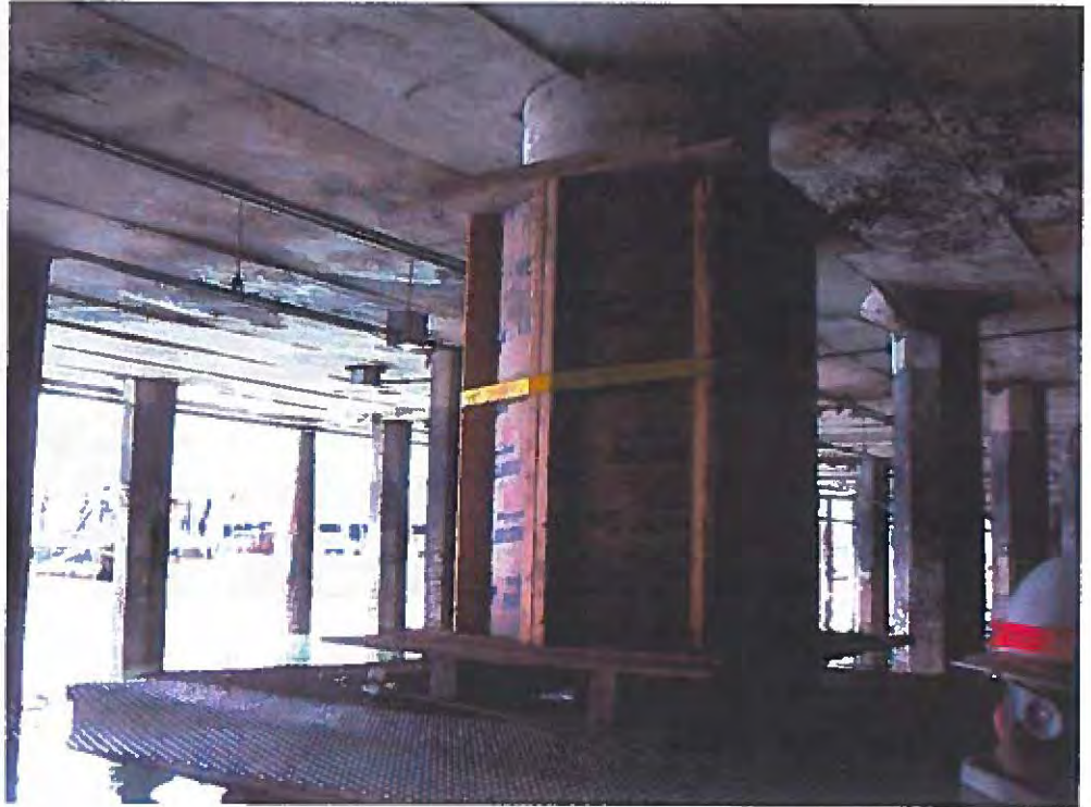
Figure 29 - Concrete Encasement Repair
