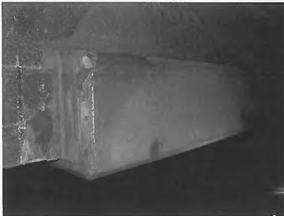
Figure 6 - Typical Cast in Place Beam Repair (5/14/2019)
