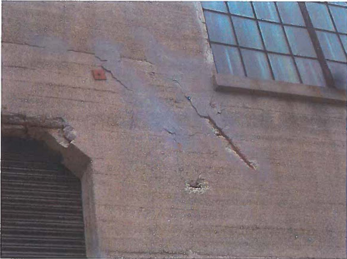
Figure 18 - Mid-wall patch re-spalling
