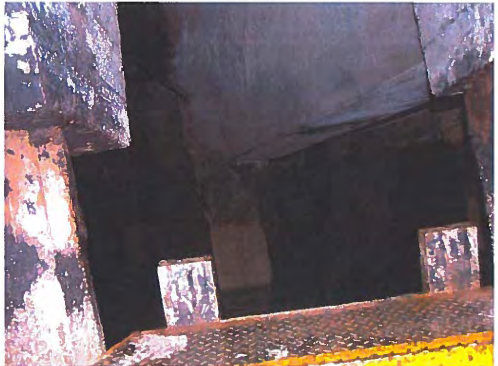
Figure 27 - Sunken Slab on Pier 31.5 (5/15/19)
