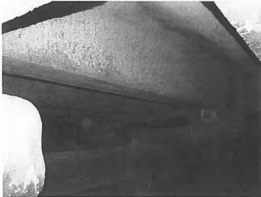
Figure 4 - Typical Shotcrete Beam Repair
