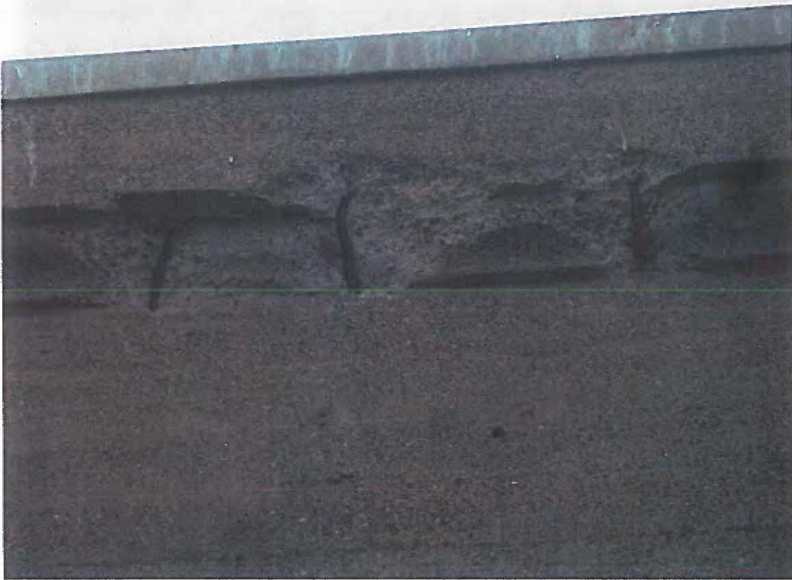
Figure 17 - Parapet spalling
