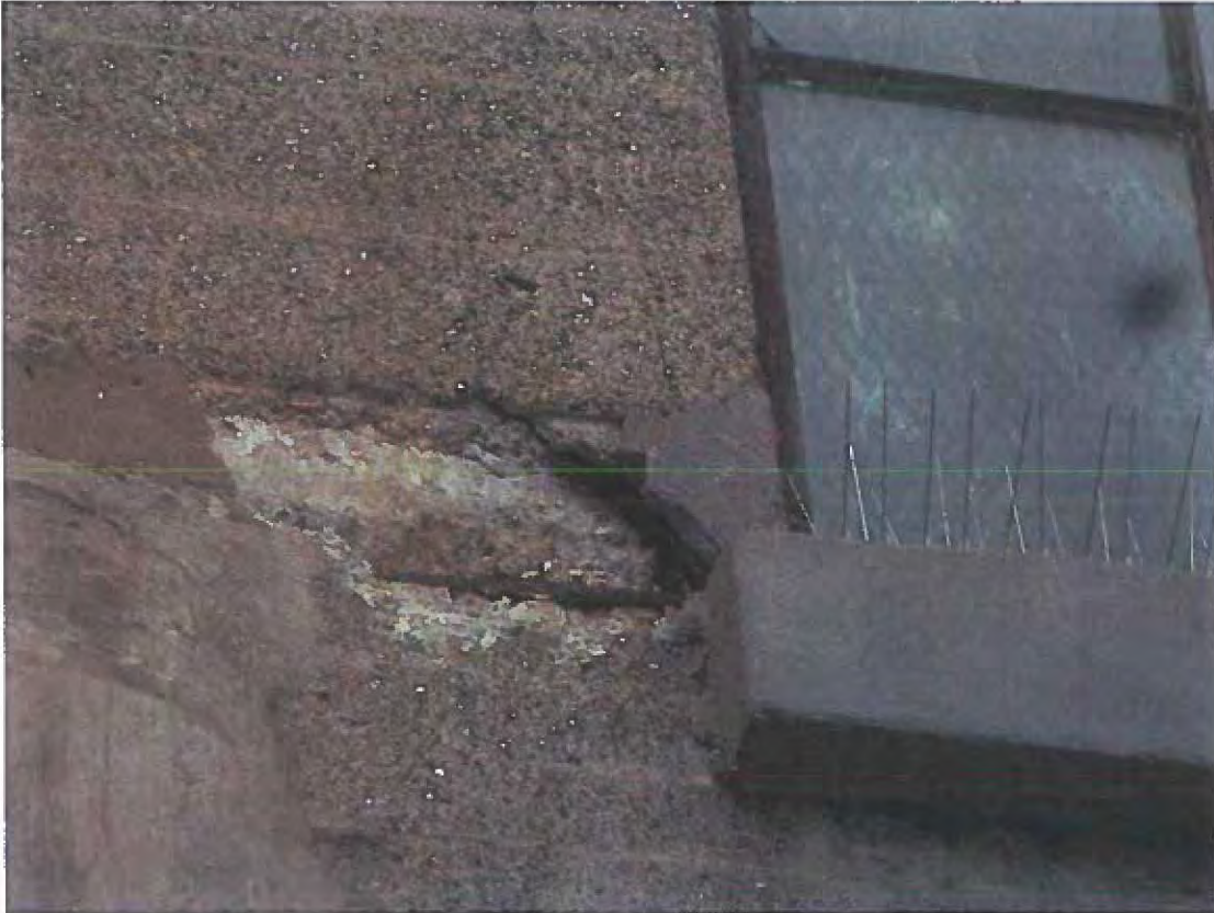
Figure 15 - Spalling at window corner
