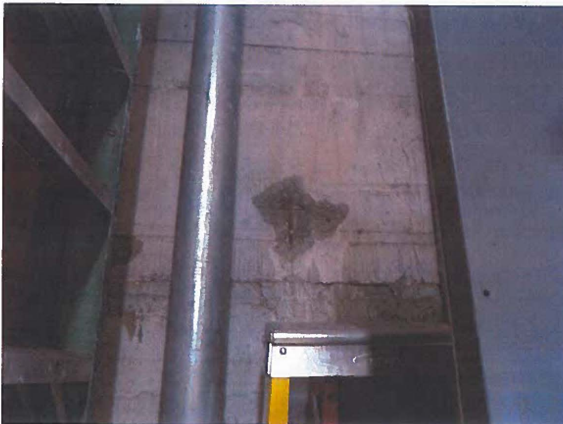
Figure 14 - Spalling at interior face of concrete wall
