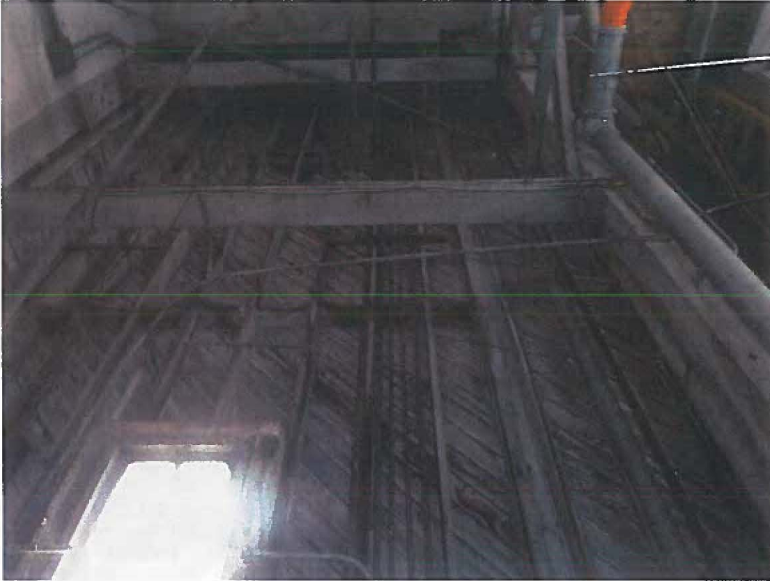
Figure 7 - Bulkhead Wall Framing
