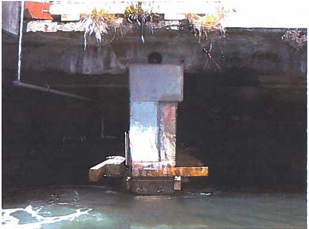
Figure 16 - Large Pile Cap Repair
