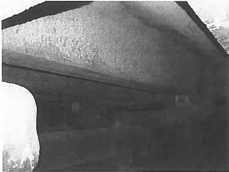
Figure 4 - Typical Shotcrete Beam Repair
