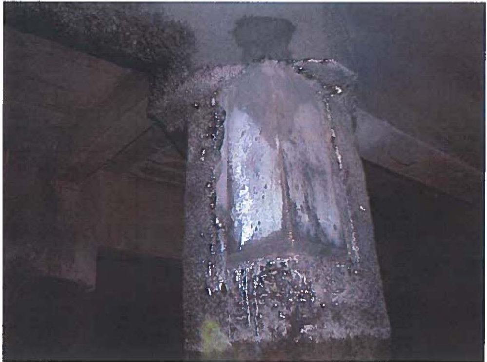
Figure 15 - Small Concrete Pile Cap Repair
