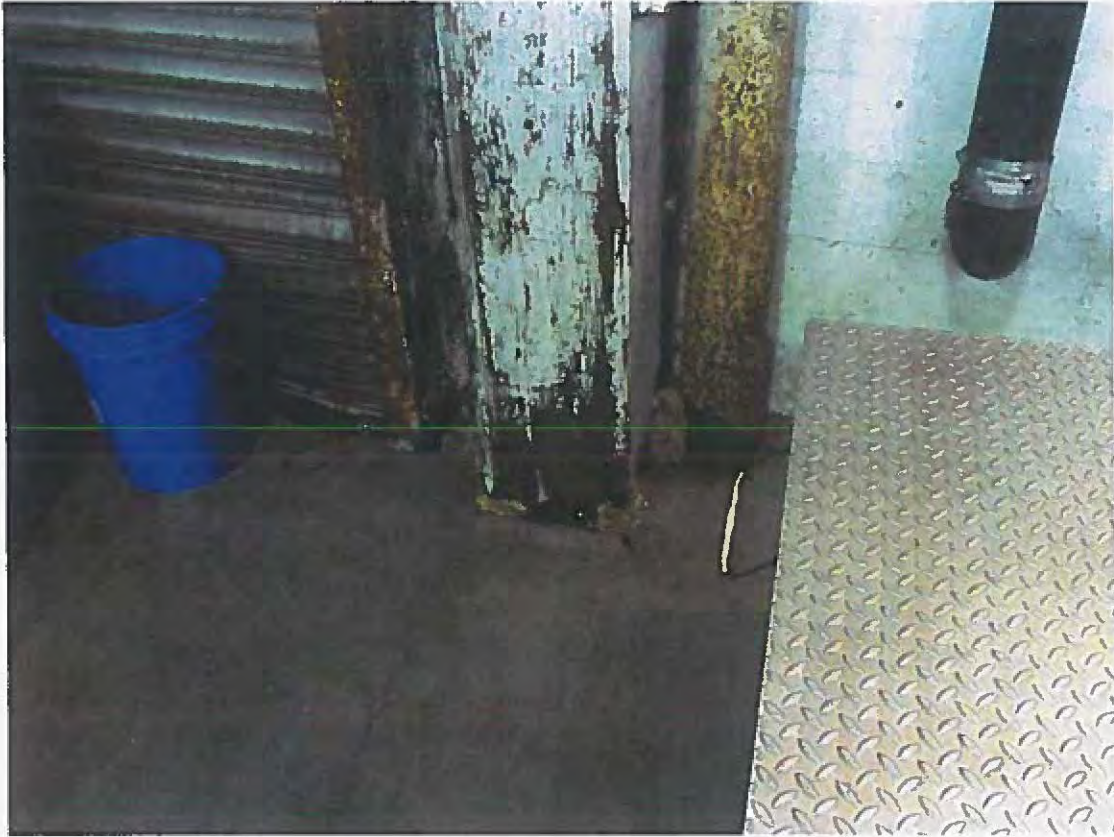
Figure 11 - Dry rot at column base next to bay door. Typical condition of timber column bases along exterior walls near bay doors and where it appears floors are frequently wetted.
