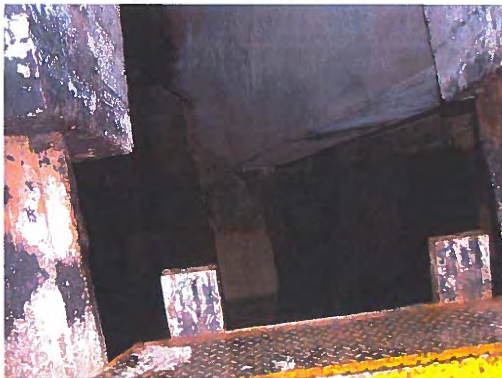
Figure 27 - Sunken Slab on Pier 31.5 (5/15/19)
