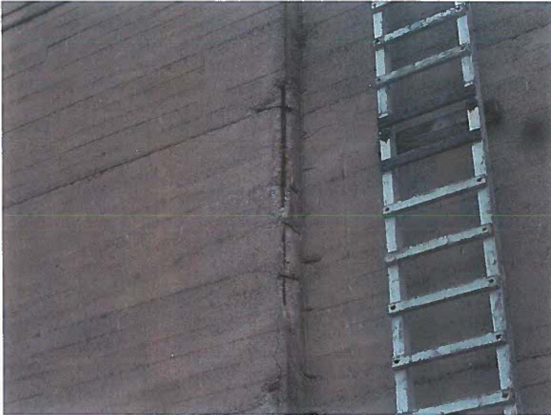
Figure 19 - Wall corner spalling
