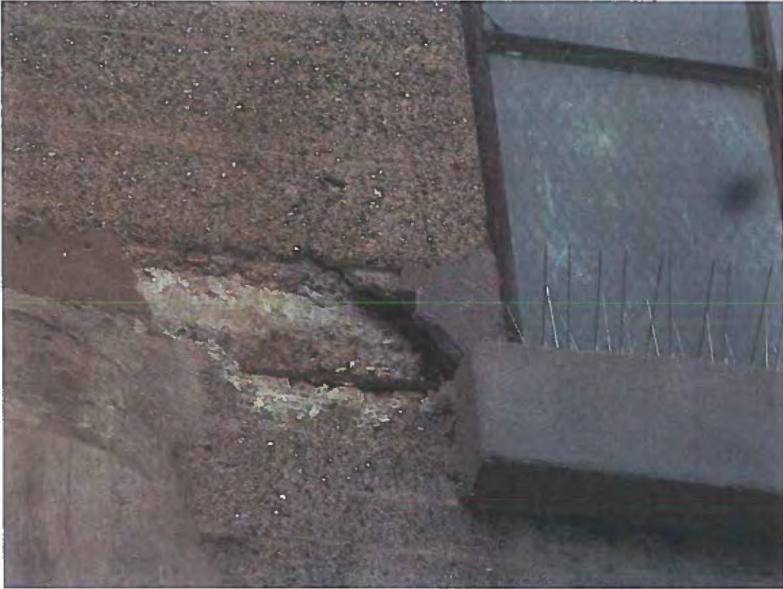
Figure 15 - Spalling at window corner
