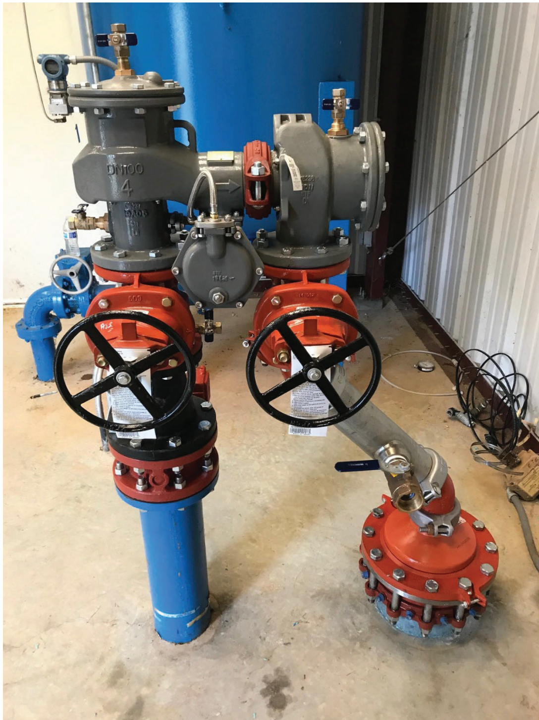
Diagram B. Backflow Device Downstream of Valve V-101
