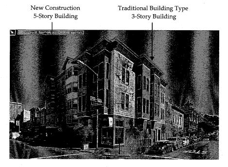
Study of Two Buildings: The corner building is a three-story building that was built pre-height limits. Next to it is a building of comparable height that fits within the existing height limit (50-X). The new building, however, is five stories. While the newer building conforms to the height limit it is not performing up to the livability and comfort standards of the older building stock.
