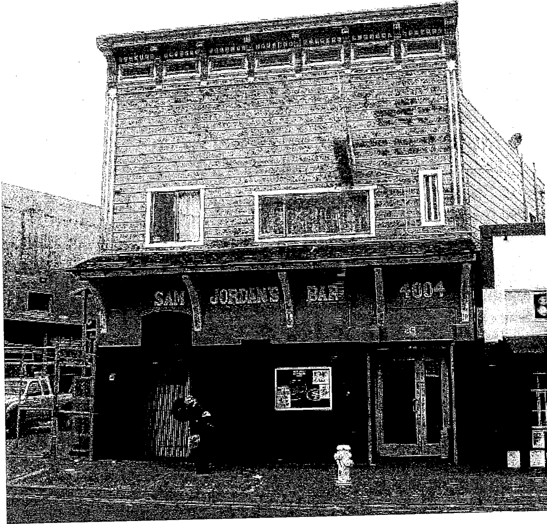
4004-4006 Third Street, Sam Jordan's Bar, primary facade.
