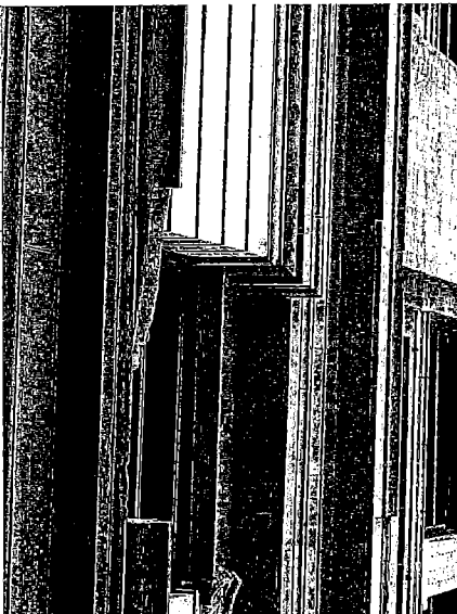
View of deteriorated colusa sandstone
