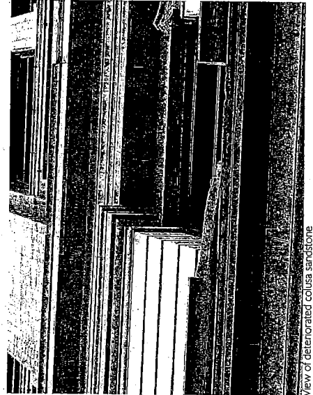
View of deteriorated colusa sandstone
