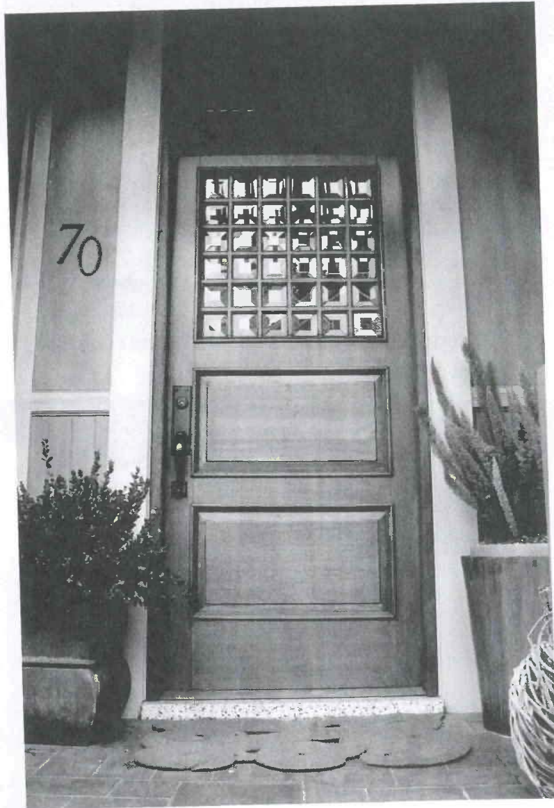
Front door. Inspect annually. Maintenance will require sanding, restain and clear coat every 3-4 years. Replace/adjust hardware as necessary.
