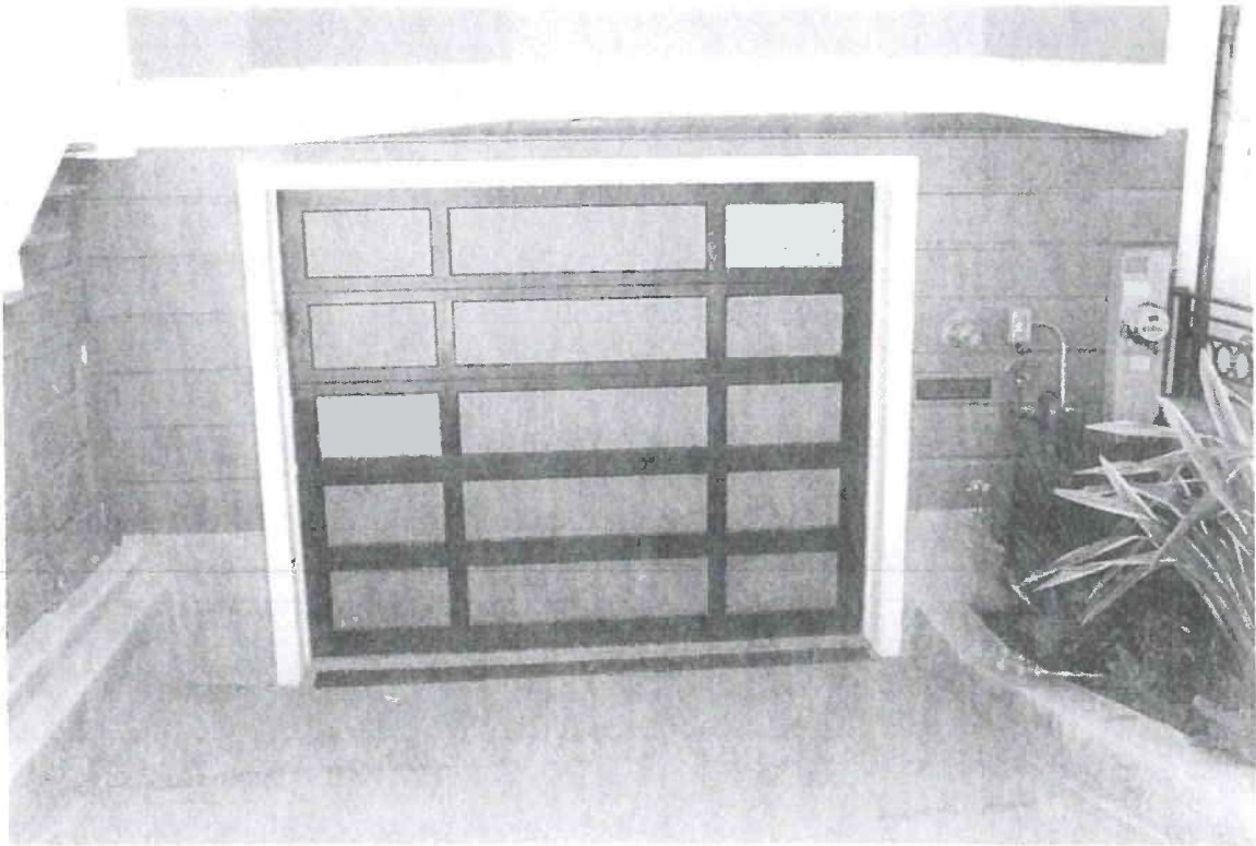
Garage door, trench drain and permeable concrete driveway
