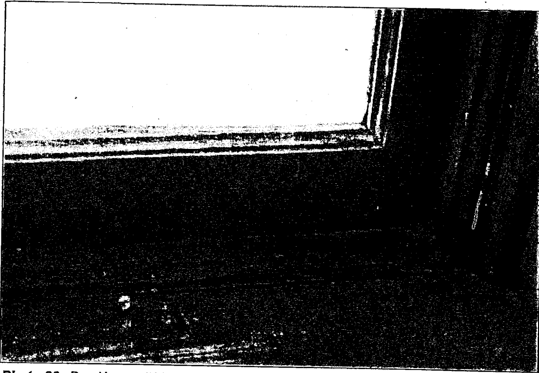
Photo 26. Burr House, 1772 Vallejo Street, 94123. Window at mansard roof. Note water damage at sill and frame.
