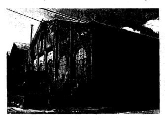
strengthening would essentially provide a complete new steel structural system to pick up the roof load, with a horizontal diaphragm system to transfer lateral loads. The entire system would lie within the envelope of the existing building. The vulnerable perimeter UMB walls would change from a structural element to a cladding tied into the new structural system. The existing 17-foot high mezzanine at the northwest corner would be continued along the remainder of the
