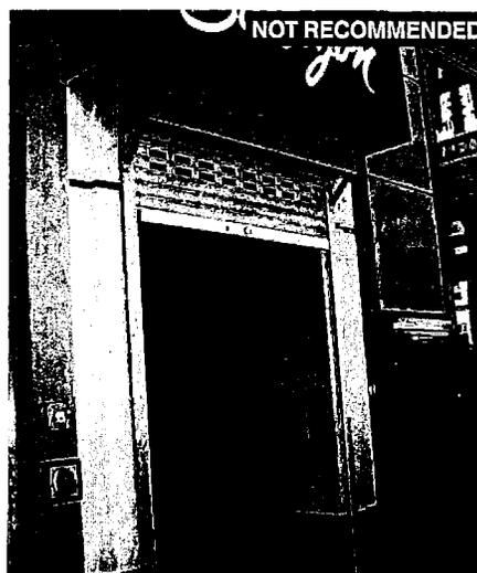
LEFT: When an external security grate is installed, its operational mechanism should be hidden from view. When fully retracted, the security grate should be concealed within the façade or behind the cladding.
