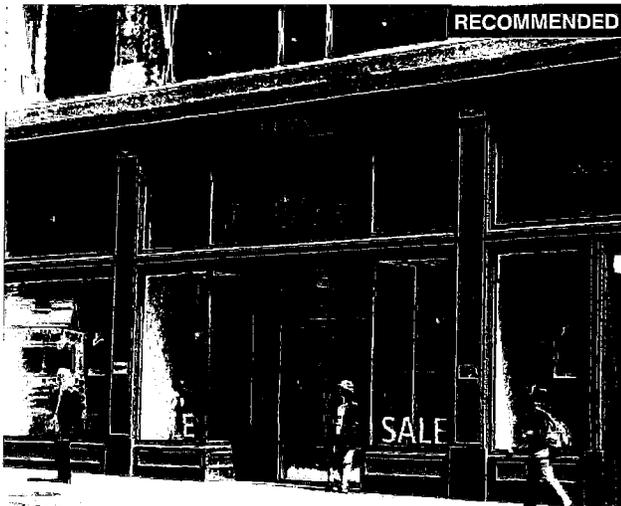
These contemporary entry doors have been located within the historic storefront. Original cast iron elements such as columns, bulkheads and the prism glass transoms have been restored. This treatment is recommended.
