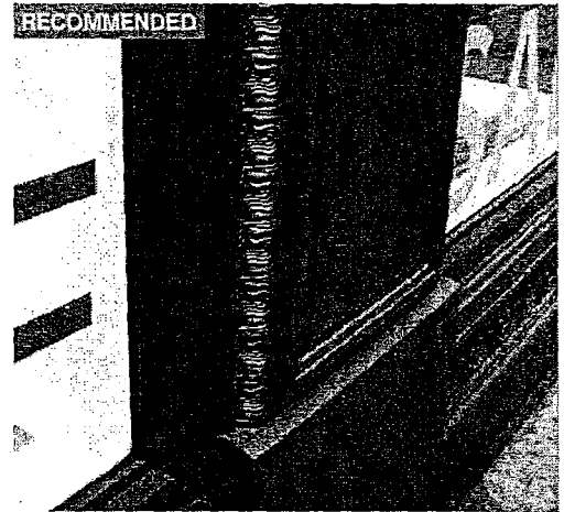
The profile on this pier and bulkhead are indicative of historic commercial architecture and should be preserved.
