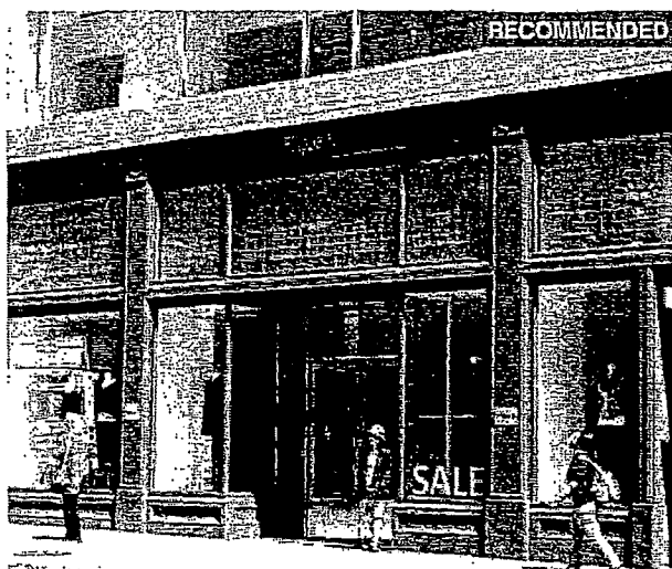
These contemporary entry doors have been located within the historic storefront. Original cast iron elements such as columns, bulkheads and the prism glass transoms have been restored. This treatment is recommended.
