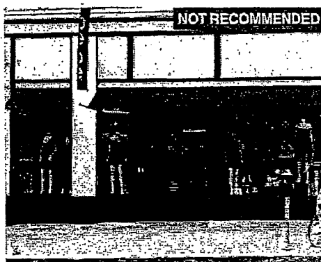
Opaque or painted glass should not be used within the transom windows. If clear glass cannot be used, translucent patterned glass is a preferred alternative. This restricts light entering the store and is not recommended.
