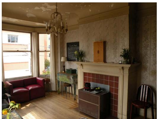
Figure 25 Rube Goldberg's living room with the bay window facing Oak Street and original fireplace mantel. The gas heater insert appears to be from the third quarter of the 20th Century but appears to be a reversible addition that did not damage the original materials or workmanship of the fireplace. Note original wallpaper on the east wall of the living room.
