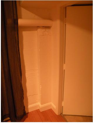
Figure 45 Impressions on the basement wall reveal that the foundations are caste board-formed concrete.
