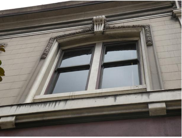
Figure 11 Primary façade window with Beaux Arts decorations of garlands, shaped keystone, and curved lintel. Two sets of paired windows in this form center the second stories of both the Gough Street façade and the Oak Street elevation.
