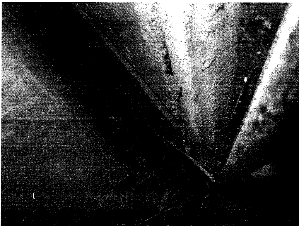
Figure 2. Soil-wood contact between stair foundation and wood property-line wall has caused decay..
