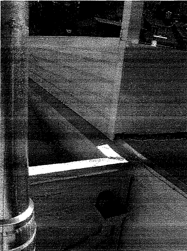
Figure 3. Soil-wood contact caused decay in property-line wall.
