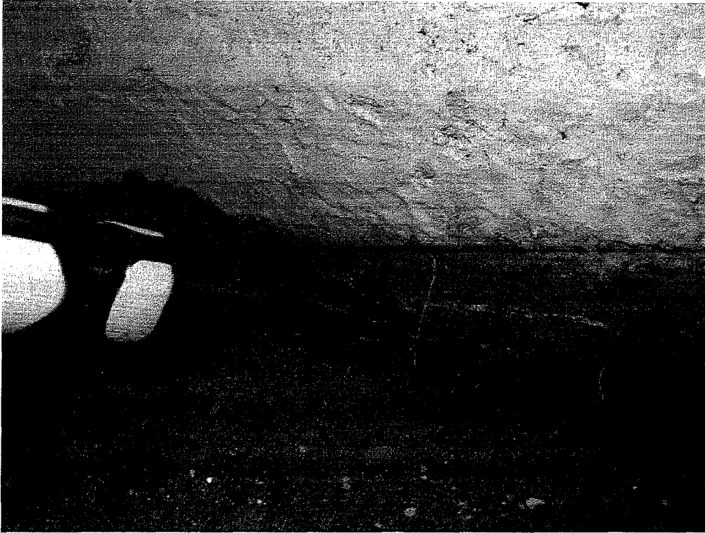
Figure 3. Soil-wood contact caused decay in property-line wall.
