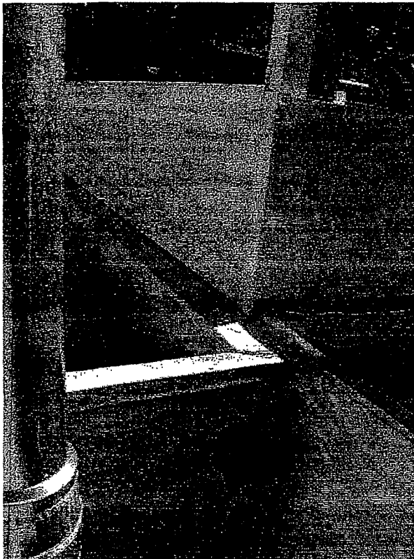
Figure 3. Soil-wood contact caused decay in property-line wall.
