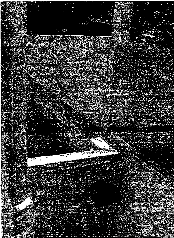
Figure 3. Soil-wood contact caused decay in property-line wall.
