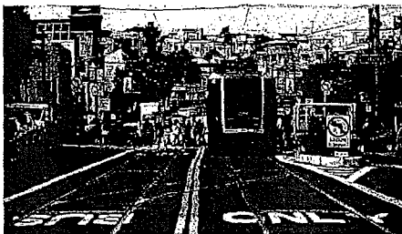
Transit-only lanes dedicate space for the buses to navigate through the traffic congestion.
