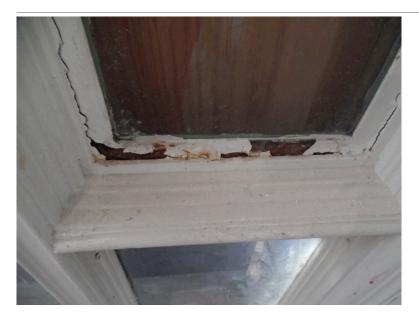
**Figure 22.** Peeling paint and corrosion at ground floor window. (Photograph by Garavaglia Architecture, Inc., April 2015.)
