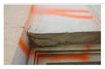
**Figure 18.** Cracked concrete above window at the seventh floor along the north elevation. (Photograph provided by RLJC, April 2015.)
